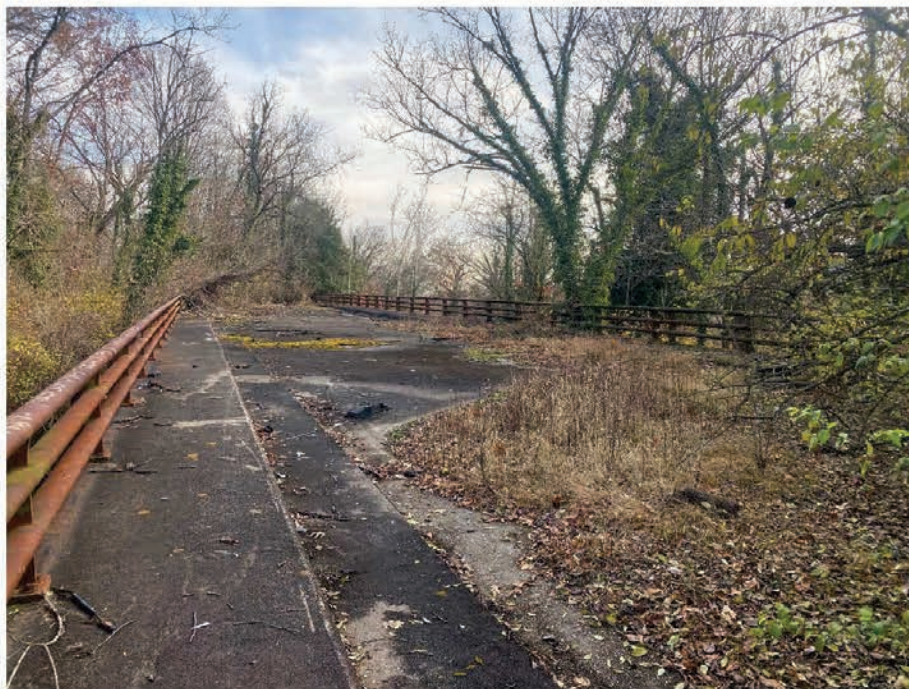
Photo: Bridge to nowhere from bridge deck
