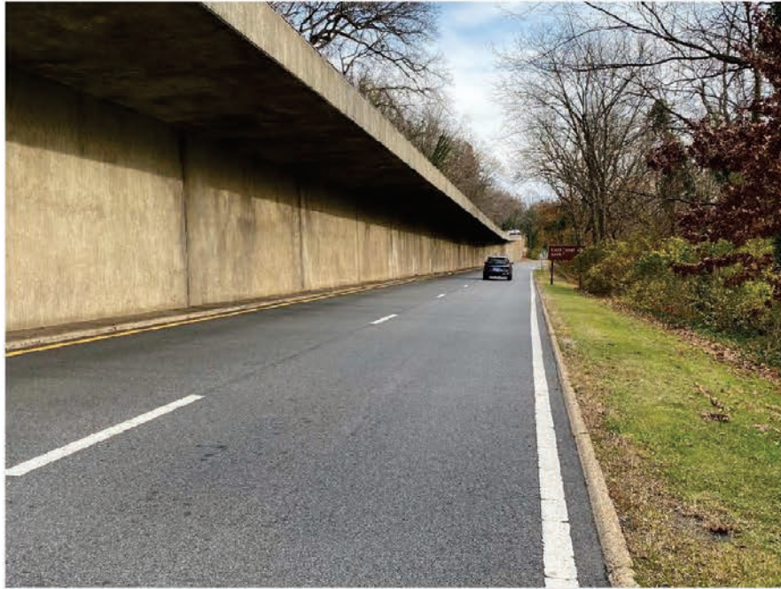
Photo: Cantilever structure from southbound Clara Barton Parkway
