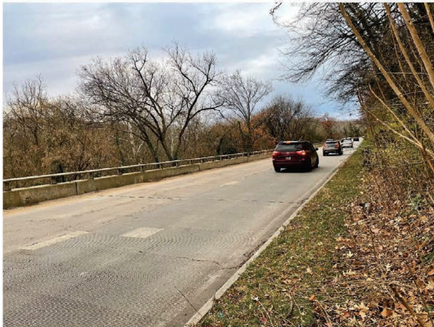
Photo: Cantilever structure from northbound Clara Barton Parkway
