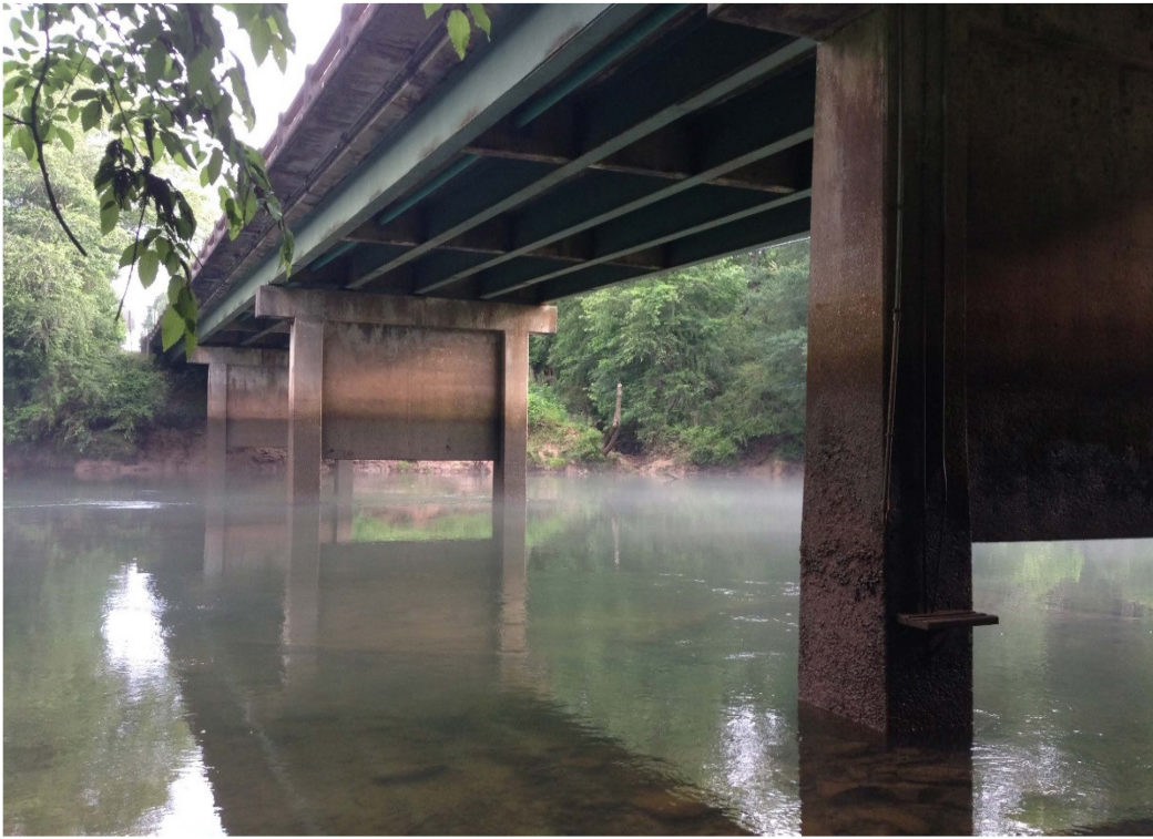
Picture of piers, looking North across the river.
