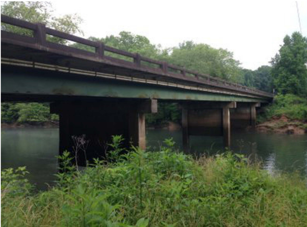
Upstream Side of bridge, looking North across the river.
