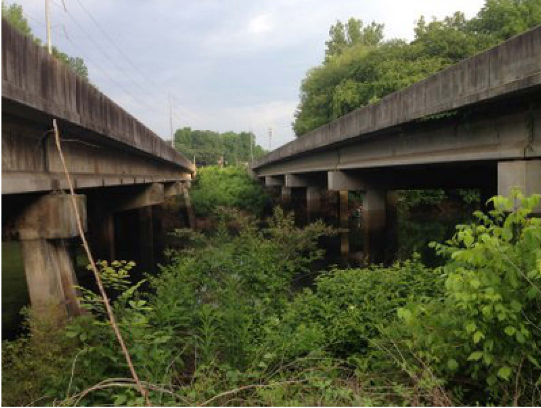
Downstream bridge at State Bridge Road/Pleasant Hill Road
