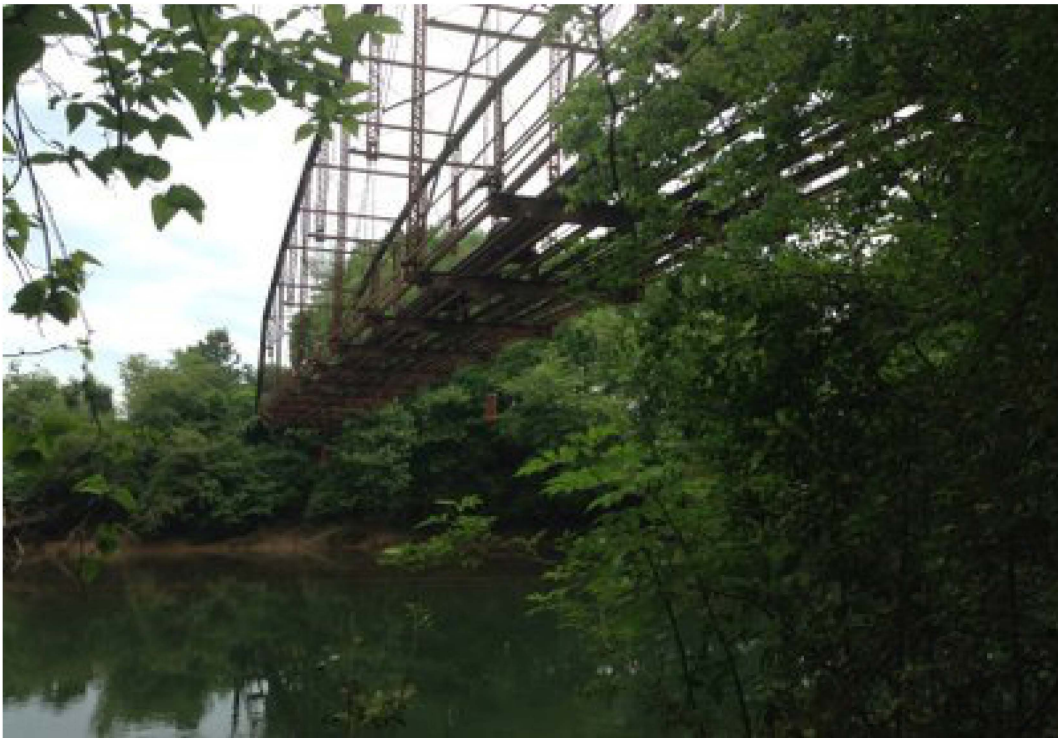
Upstream pipe crossing/trestle at Rogers Bridge Road
