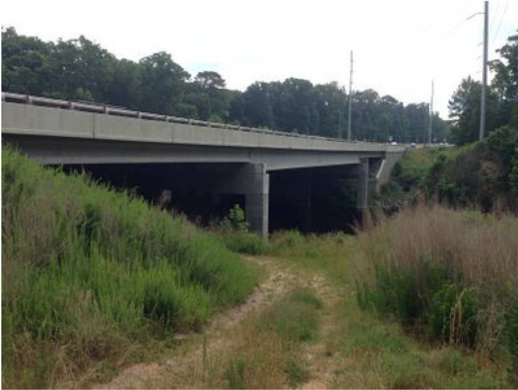
Upstream Bridge at McGinnis-Ferry Road
