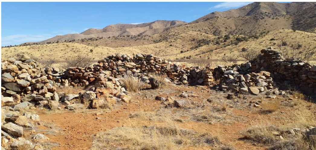
Figure 54. Dragoon Springs Station, showing ruins with low, partially collapsed stone walls arranged in rough rectangular enclosures on a reddish dirt floor
