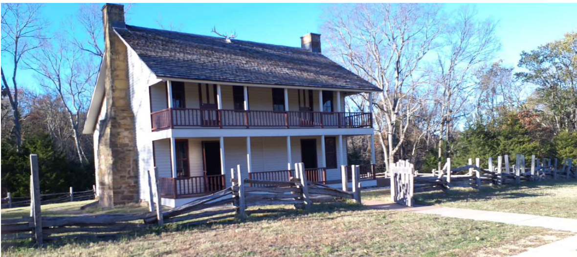
Figure 12. Elkhorn Tavern, showing the restored historic tavern building at the battlefield site, with adjacent historic road trace
