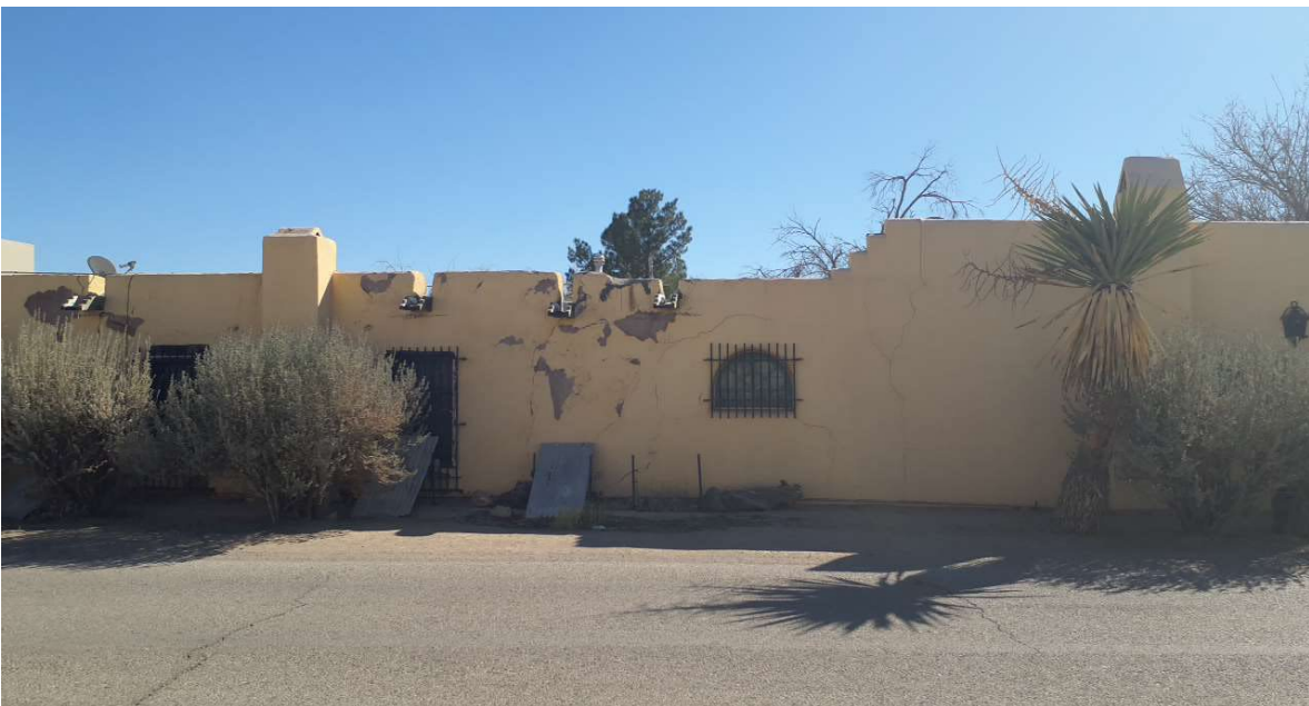
Figure 45. San Elizario Station, showing an adobe building with a flat roof and stepped parapet, with a yucca plant and paved roadway emphasizing the historic border community setting
