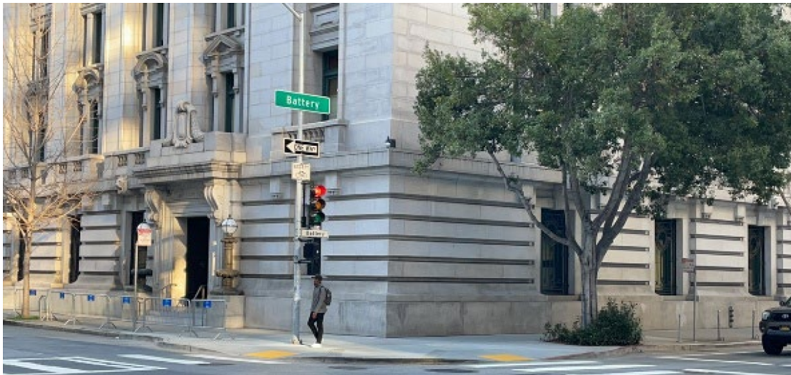
Figure 72. San Francisco Post Office in 2025 at the corner of Battery Street, showing a monumental Beaux-Arts stone building with heavy rusticated walls, ornate window surrounds, and recessed arched entrances
