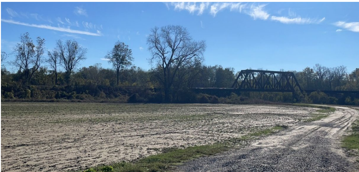
Figure 15. Madison Terminus, showing an open agricultural field at the terminus with a gravel track in the foreground and a steel railroad bridge in the background marking the transition from rail to stage travel
