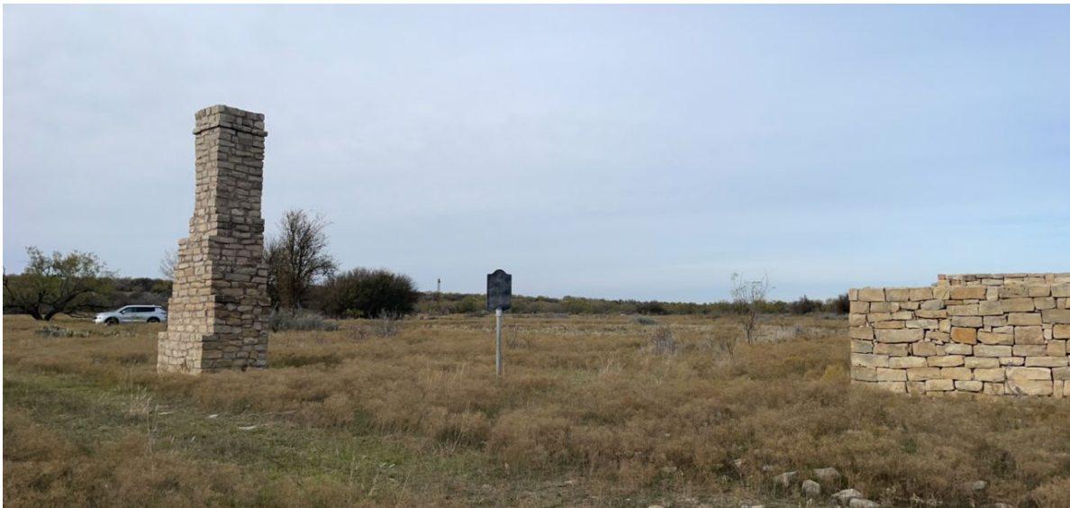
Figure 34. Smith's Station in 2025, showing a stone chimney and a reconstructed low stone wall at the former Butterfield Overland Mail Company stage station site
