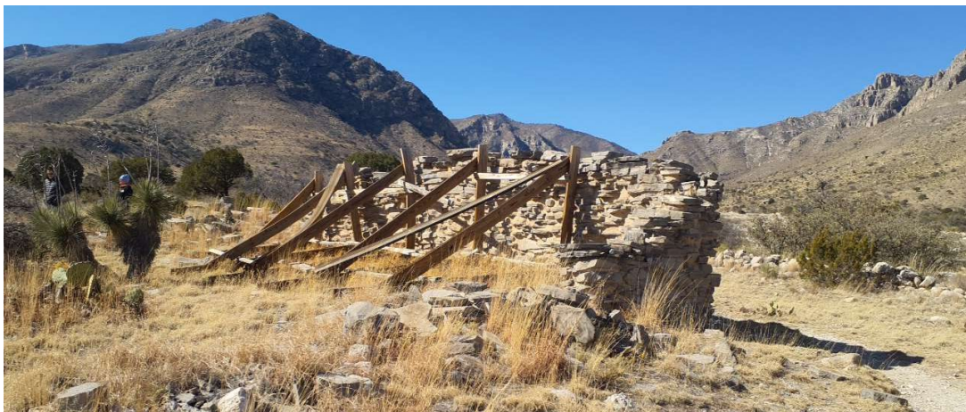
Figure 38. The Pinery Station in 2025, showing a stone foundation and reconstructed wooden supports at the former stage station
