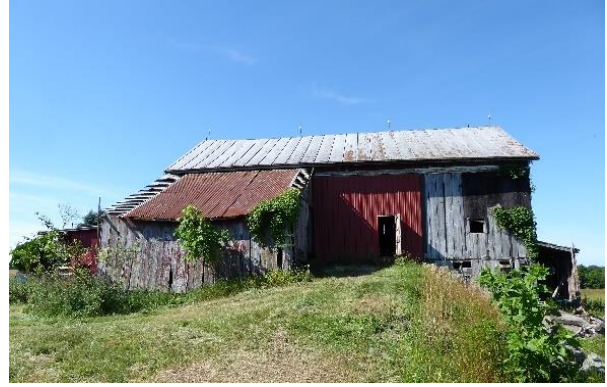
North elevation positive drainage. Photo: HPTC, 06/21/17.
