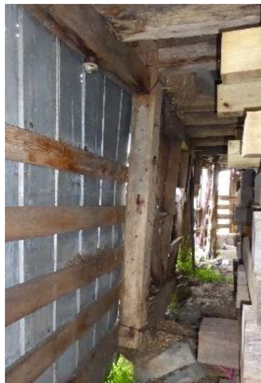
P4 supports the rim beam at the west elevation timber-frame foundation wall of the wagon shed. It is likely historic. Photo: HPTC, 06/21/17.
