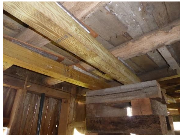
Modern cribbing and supplemental framing support the joists in the wagon shed due to deteriorated foundations. Photo: HPTC, 06/21/17.
