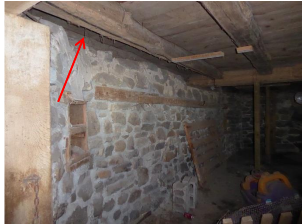
The western interior foundation wall sill plate is exposed along its interior length. Photo: HPTC, 06/21/17.
