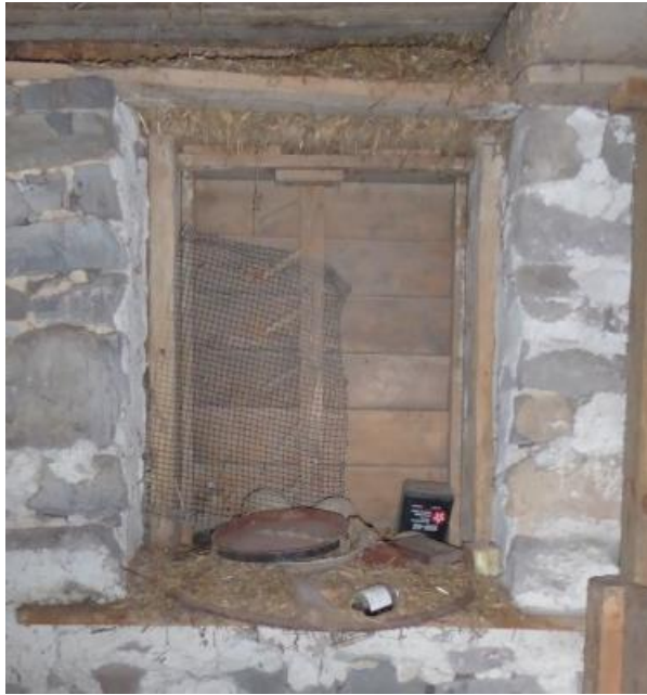
The interior of the original louvered opening in the barn's north elevation stone foundation wall. Note the mechanism which moved all the slats at the same time. Photo: HTPC, 06/21/17.
