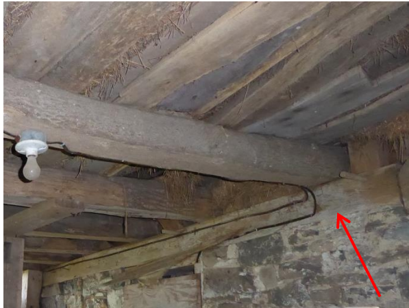
The sill plate atop the western interior stone foundation wall (arrow) supports the perpendicular joists above the wagon shed. Photo: HPTC, 06/21/17.
