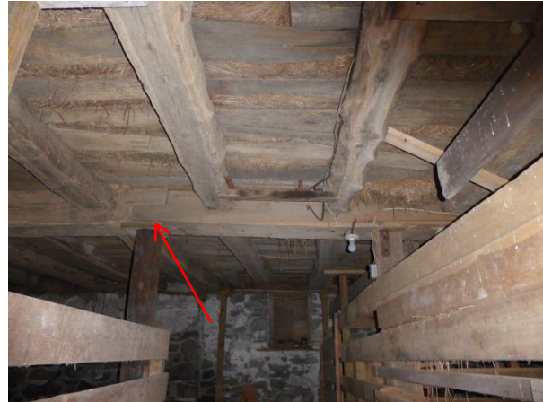
The summer beam is half lapped at the mid-point. The joint is supported by modern replacement P22. Photo: HPTC, 06/21/17.
