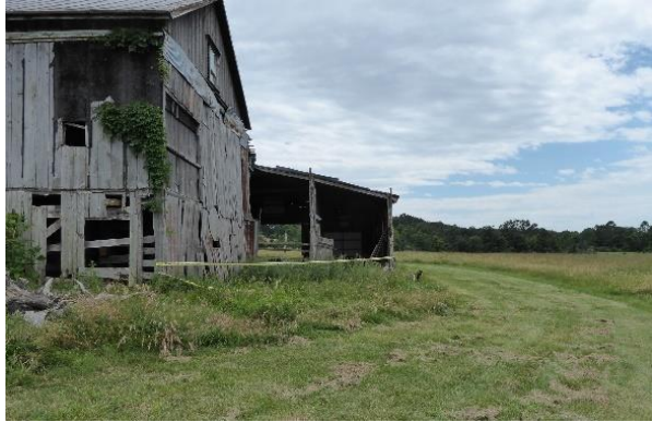
West elevation neutral drainage. Photo: HPTC, 06/21/17.
