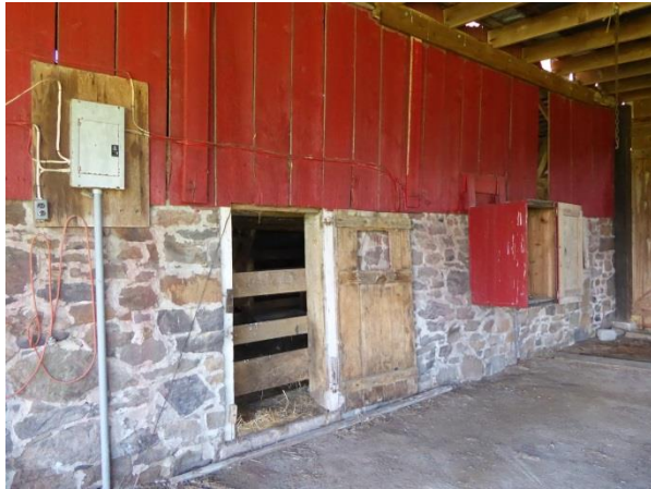
Part of the bank barn is supported by a stone foundation. Photo: HPTC, 06/22/17.
