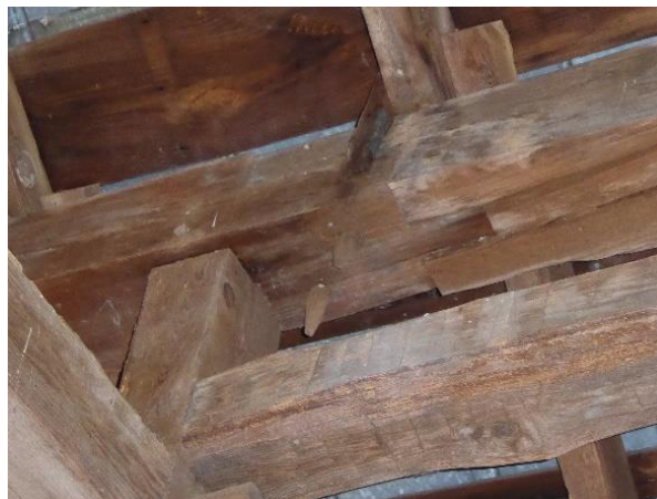
The mortise-and-tenon timber frame of the Bishop Barn is typical for bank barns. Photo: HPTC, 06/21/17.
