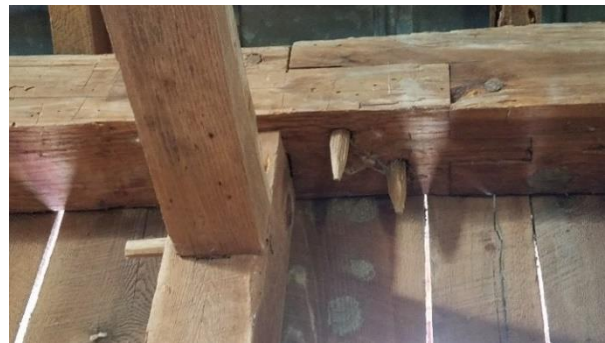
The barn utilizes pegs at the mortise and tenon connections. This complex scarf joint is located in the roof plate and is a CDF. Photo: HPTC, 06/21/17.
