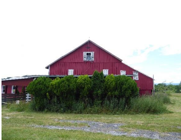
The east elevation of the bank barn and outshed granary is obscured by a modern loading shed and vegetation. Photo: HPTC, 06/21/17.
