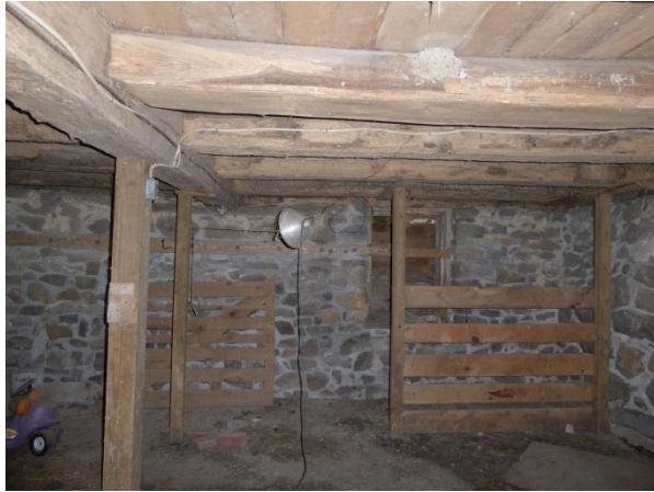
The N-S joists are half lapped over the summer beam at the midpoint. Photo: HPTC, 06/21/17.
