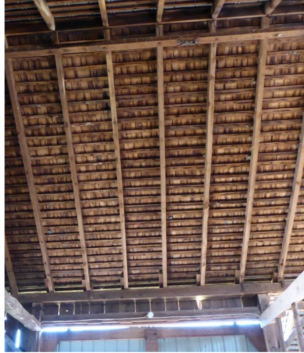
Original wood shingles can be seen on the underside of the north slope of the barn gable roof. Photo: HPTC, 06/20/17.
