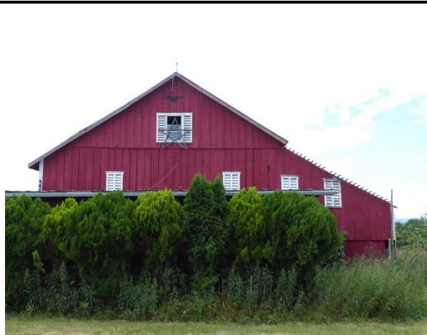
The bank barn has an asymmetric gable roofline. The outshed granary has steep shed roofline. Photo: HPTC, 06/22/17.
