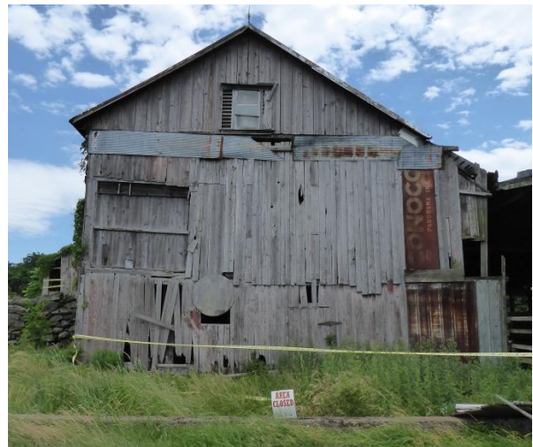
The exterior of the west wall. The siding is not historic and was likely cobbled together when the addition was removed. Photo: HPTC, 06/21/17.
