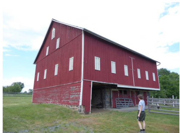
The Basil Biggs Farm Barn is also similar in construction as the Bishop Barn. Photo: HPTC, 06/21/17.
