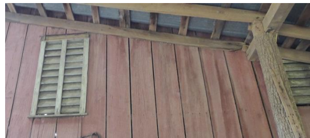
One of the louvered openings on the barn's south elevation is completely covered by an addition. Its paint is fading and it is missing a piece of trim. Photo: HTPC, 06/21/17.
