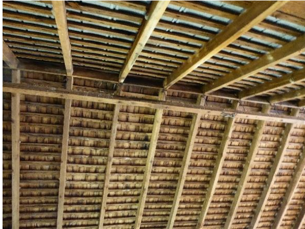
The rafters meet at the continuous ridge plate. A hay track is hung from this plate. Photo: HPTC, 06/21/17.
