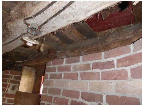
The east elevation sill exposed on the interior of the lower level. Photo: HPTC, 06/21/17.
