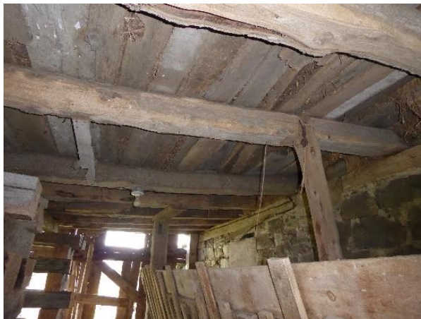
The joists above the wagon shed do not match suggesting they have been replaced over time. Photo: HPTC, 06/21/17.
