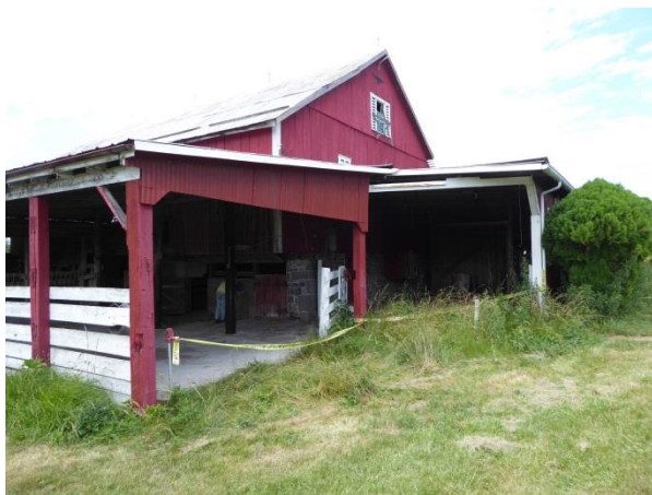
The loading shed on the east elevation, right, and the garage on the south elevation, left, are not CDFs. Photo: HPTC, 06/22/17.
