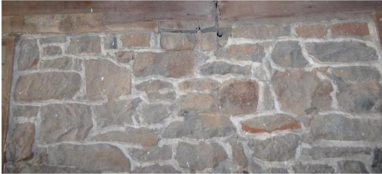
The stone foundation walls, in a random rubble pattern, seen at the Bishop barn in granite, are a typical foundation material for bank barns. Photo: HPTC, 06/21/17.
