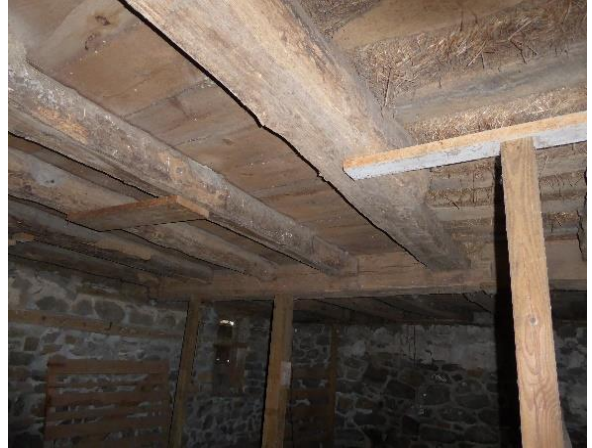
Exposed upper level structural floor framing as seen from the lower level of the barn. Photo: HPTC, 06/21/17.
