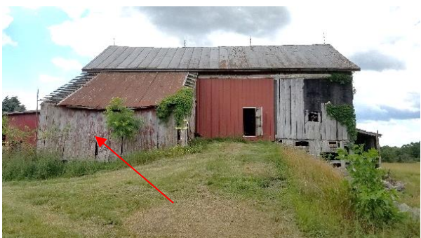
Attached outshed granary on the north elevation of Bishop Barn. Photo: HPTC, 06/21/17.
