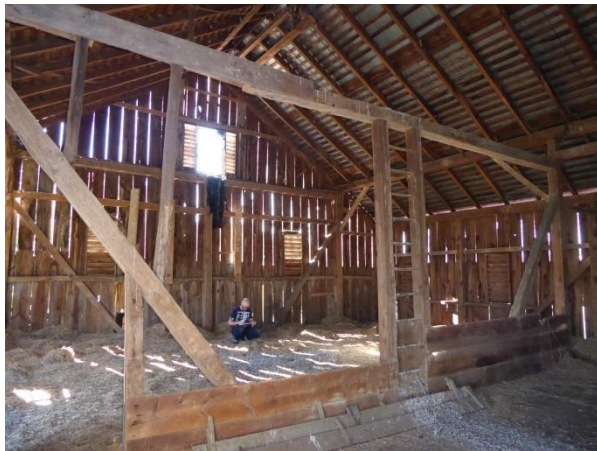
The upper level of the barn is framed with hand-hewn and circular-sawn timbers. Photo: HPTC, 06/21/17.
