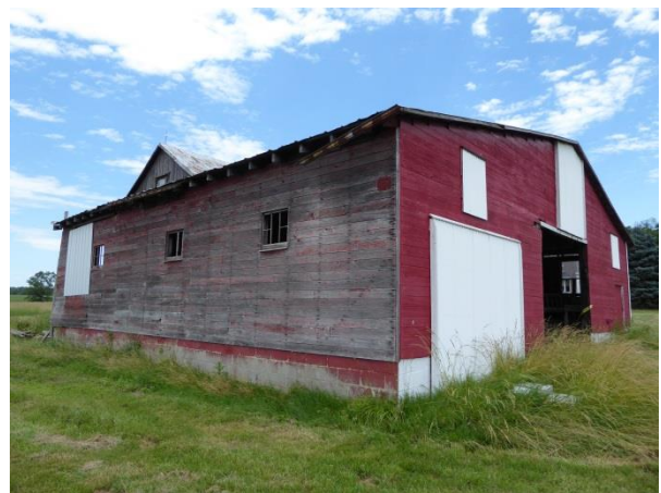
The milking parlor on the south elevation is not a CDF. Photo: HPTC, 06/22/17.
