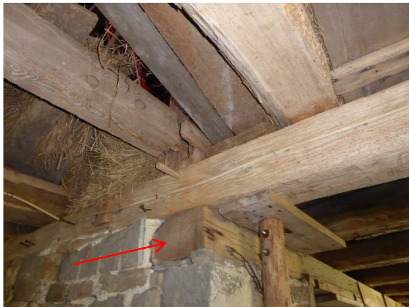
The south forebay wall sill (arrow) supports the perpendicular floor joists and runs under the west stone foundation wall sill. Photo: HPTC, 06/21/17.
