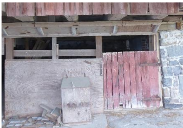
The doors located in the lower level forebay are nearly identical with long doors above. D004 is seen here. Photo: HPTC, 6/21/17.
