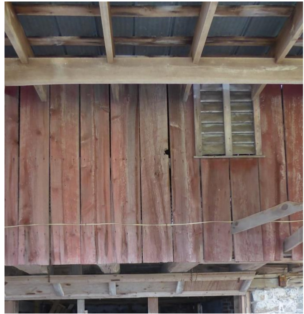
The exterior siding on the barn and the louvered openings are likely original, but are partially obscured by non-CDF additions. Photo: HPTC, 06/22/17.
