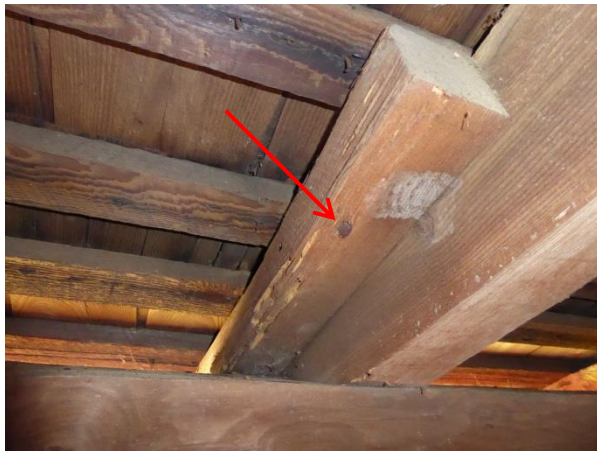
A sprocket added to the end of a rafter on the south slope. Note the spike holding the two together. Photo: HPTC, 06/20/17.
