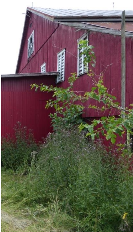
The east elevation is clad with painted vertical siding boards. Photo: HPTC, 06/21/17.
