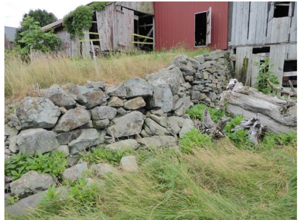
The bank on the north addition is a CDF. Photo: HPTC, 06/21/17.
