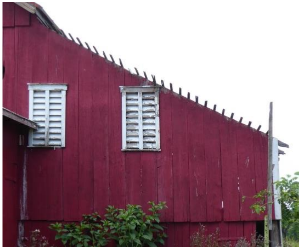
Extant louvers in the east elevation of the outshed granary. Photo: HPTC, 06/21/17.
