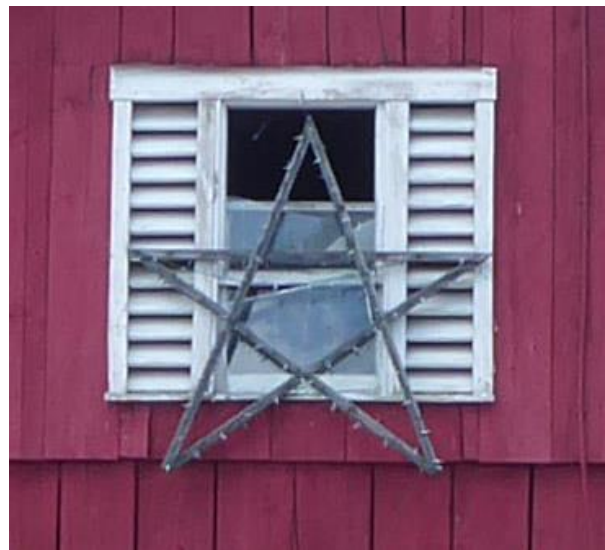
The tripartite louvered opening under the east gable end. The sash in the center are not original. Photo: HPTC, 06/21/17.
