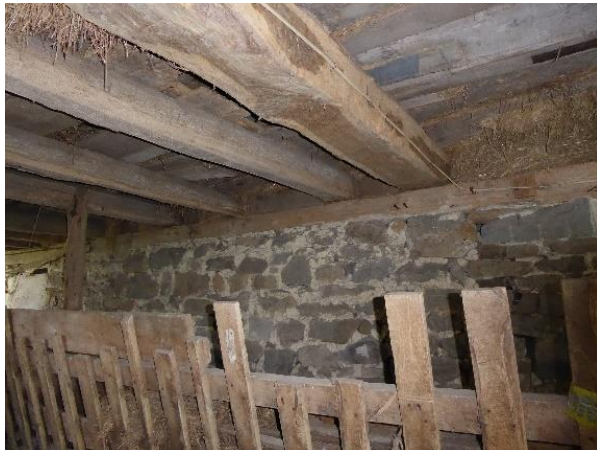
The east ends of the joists above the wagon shed are supported by the sill atop the west interior stone foundation wall. Photo: HPTC, 06/21/17.
