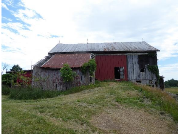
The north elevation with historic outshed granary addition. Photo: HPTC, 06/21/17.
