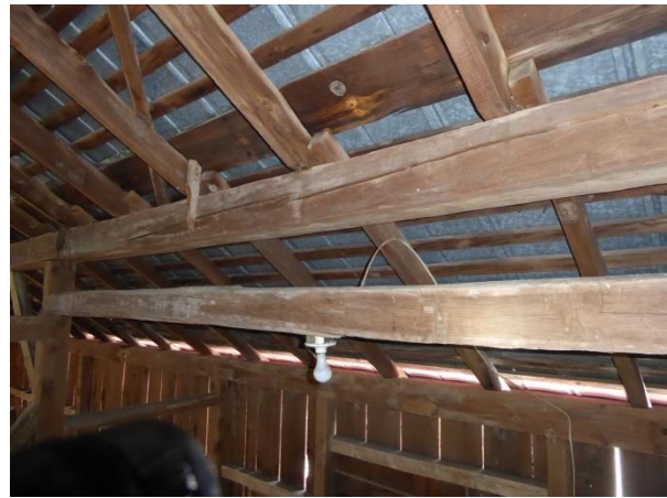
The retained original skip sheathing provides stabilization from racking. Wood shingles wood have also been attached to the sheathing originally. Photo: HPTC, 06/21/17.
