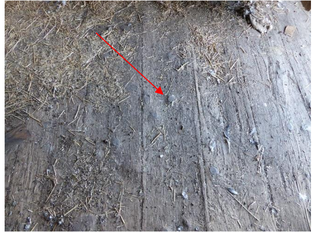
Threshing floor wood flooring is held down with face-nailed spikes. Photo: HPTC, 06/21/17.
