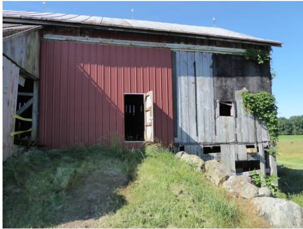
The north elevation of the barn. The sliding barn door is in the center. The outshed granary covers the eastern portion. Siding and vines cover the western portion. Photo: HPTC, 06/21/17.
