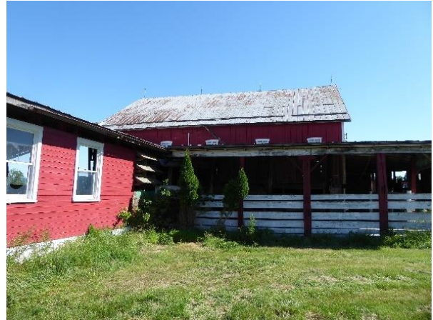
The south elevation with modern milking parlor (left) and modern garage (right). Photo: HPTC, 06/21/17.
