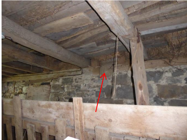
The barn summer beam is supported on its west end by the interior stone foundation wall. Photo: HPTC, 06/21/17.
