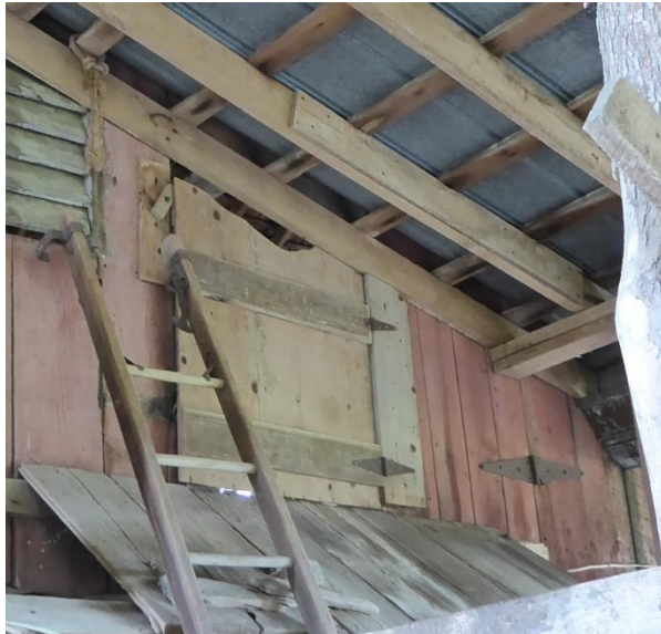
D002 has been altered so that it could be somewhat usable despite the addition roof. Photo: HPTC, 06/21/17.
