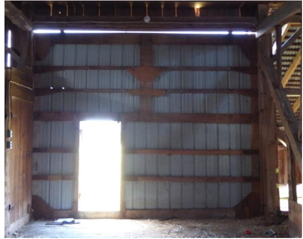
The interior of D101 with wood framework supported the metal cladding. Photo: HPTC, 06/21/17.
