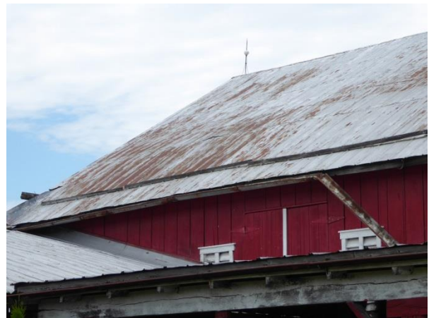
The ribbed metal roofing of the south slope of the bank barn is not character defining, as it likely postdates the period of significance. The snow boards are not CDFs either. Photo: HPTC, 06/22/17.
