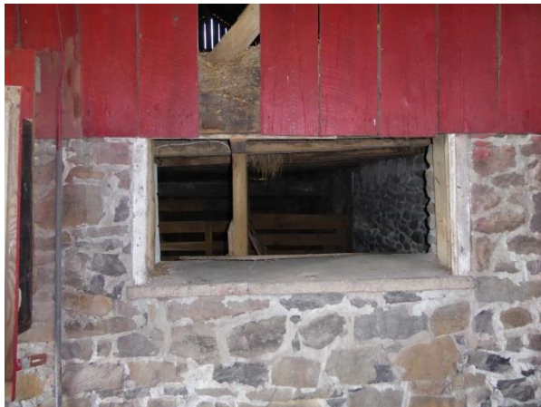
One of the louvered openings on the barn's south elevation is completely covered by an addition. Its paint is fading and it is missing a piece of trim. Photo: HTPC, 06/21/17.
