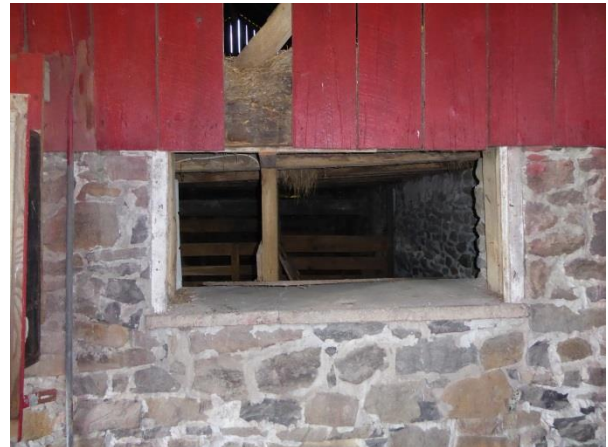
The window opening on the east elevation of the barn stone foundation has been altered and is no longer a CDF. Photo: HPTC, 06/22/17.
