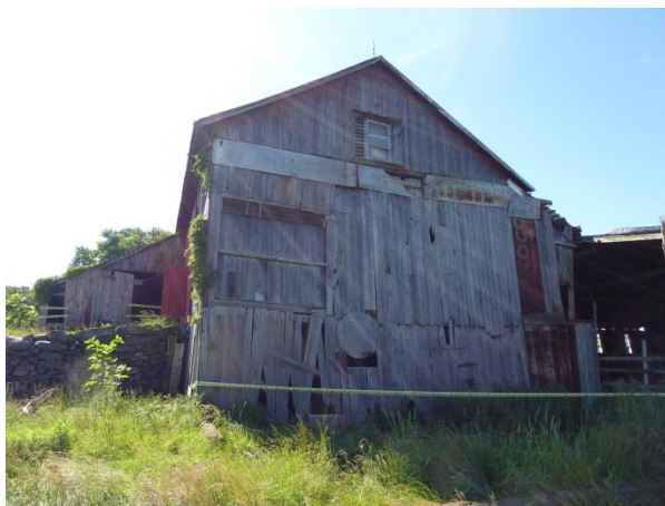
The shape and mass of the bank barn and outshed granary addition (left) are character-defining features. Photo: HPTC, 06/21/17.
