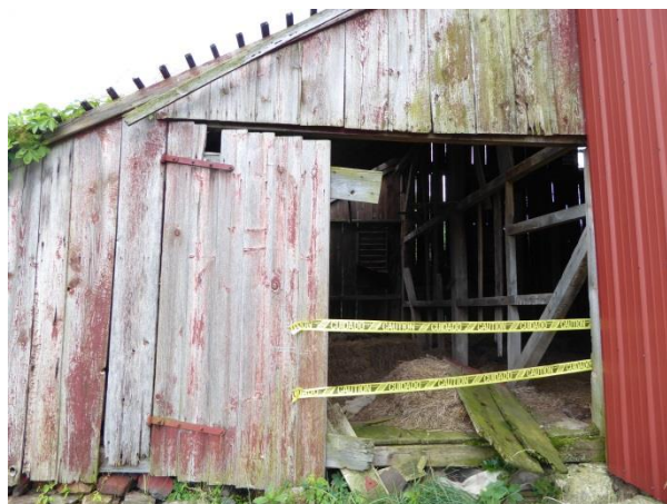
One of the paired doors remains at D003. Photo: HPTC, 06/20/17.
