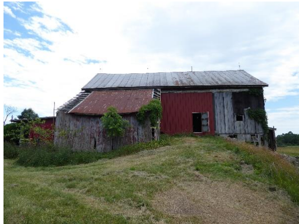
A typical bank barn has a bank to provide access to the upper level, seen at the Bishop Barn on the north elevation. Photo: HPTC, 06/21/17.
