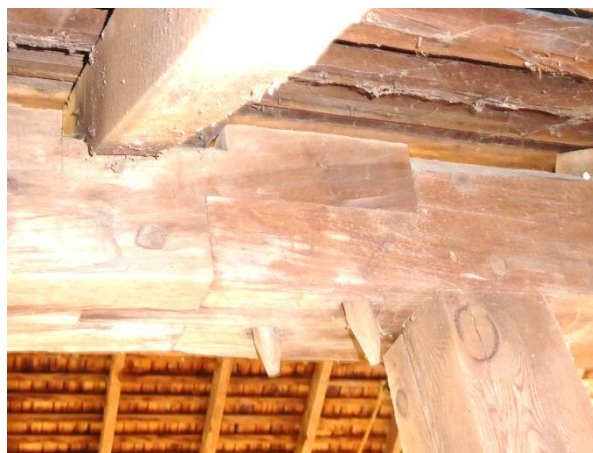
Long pieces of the roof plate are pegged together using a halved bridled scarf joint to run the entire length of the barn from the west exterior wall to the east exterior wall over the two bents. Photo: HPTC, 06/21/17.
