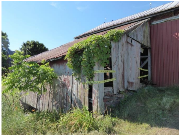
The outshed granary on the north elevation is a CDF. Photo: HPTC, 06/21/17.
