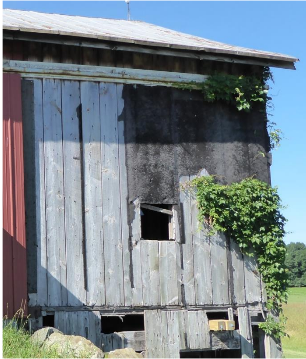
A louvered opening is hidden behind the black roofing material on the north elevation of the barn. The opening has been altered for access into the interior granary. Photo: HPTC, 06/21/17.
