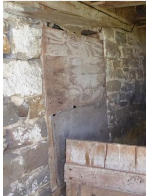
The opening in the west elevation stone foundation wall likely matched that seen in the north elevation originally. Photo: HTPC, 06/21/17.
