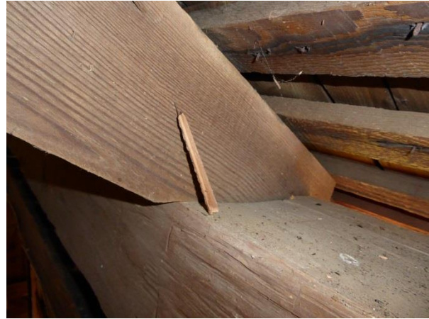
The housed birdsmouth rafter tail on the south slope at the roof plate. This connection is also spiked. Photo: HPTC, 06/21/17.
