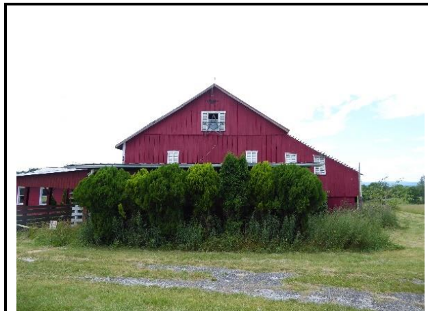
The Bishop Barn has asymmetrical gable-end walls to compensate for the extended forebay on the south elevation. Photo: HPTC, 06/21/17.
