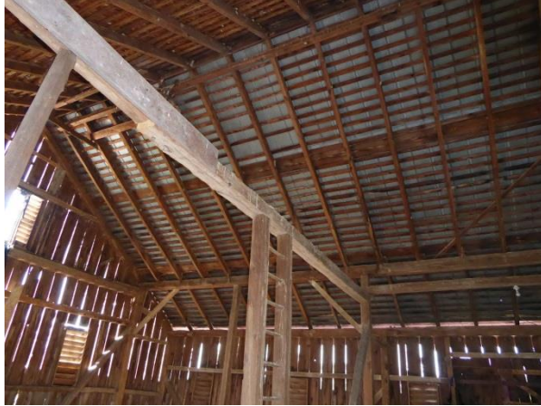
Exposed roof framing as seen from the upper level of the barn. Photo: HPTC, 06/21/17.
