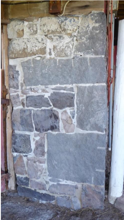
Coursed ashlar and rubble stone foundation walls. Note the quarry marks. Photo: HPTC, 06/22/17.
