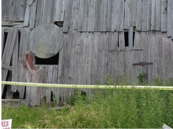
A non-original window and door opening on the west elevation of the lower level wagon shed. Photo: HPTC, 06/22/17.
