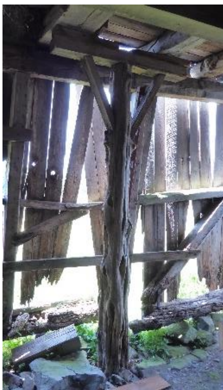
P3 is a replacement post located along the west elevation of the timber-frame foundation wall of the wagon shed. Photo: HPTC, 06/21/17.
