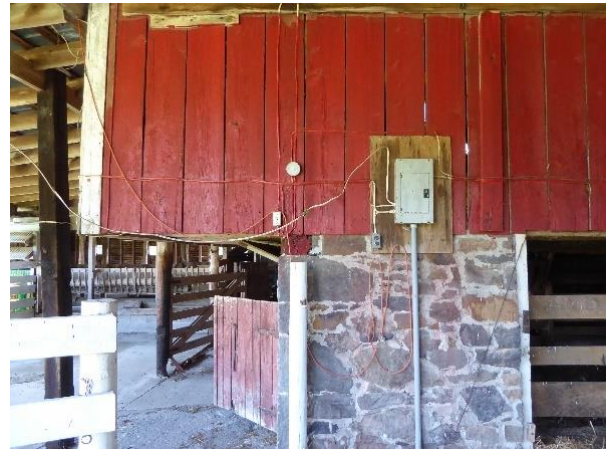
A typical bank barn includes an overhanging forebay. At the Bishop Barn, the forebay is located on the south elevation. Photo: HPTC, 06/21/17.
