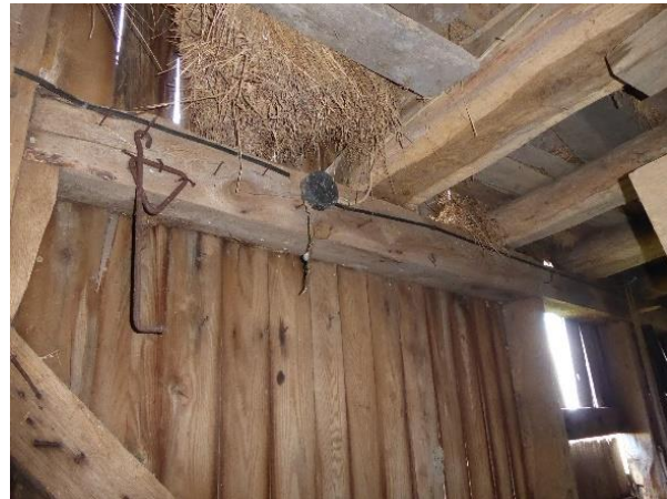
The west ends of the joists above the wagon shed are supported by the horizontal beam in the west frame exterior wall. Photo: HPTC, 06/21/17.
