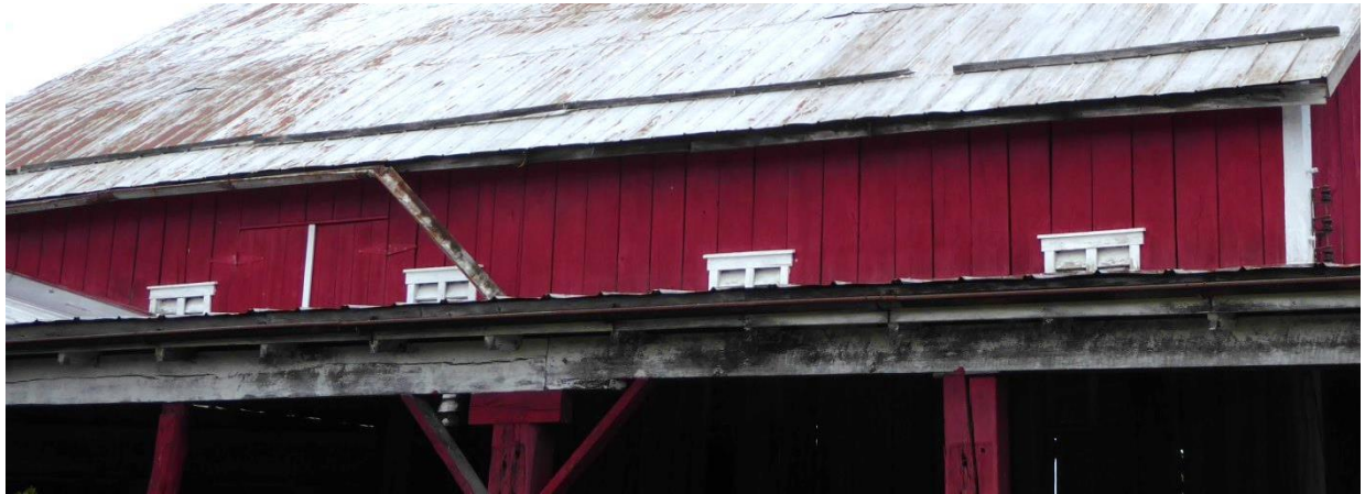
Original threshing are located on the south elevation of the upper floor of the barn. They are covered and made inoperable by the roof of the garage addition. The original louvers have also been covered with roofs of additions. Photo: HPTC, 06/22/17.
