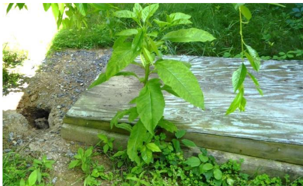
D002, exterior, with resident groundhog. Photo: HPTC, 06/08/17.
