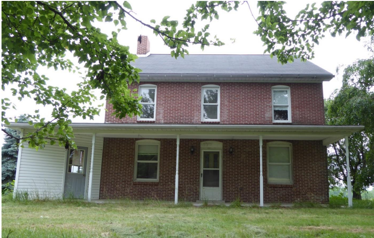
East elevation. Second-floor window openings of the main block are CDFs. First-floor door opening is a CDF, but first-floor window openings are not. Openings in the sunroom (at left) are not CDFs. Sash and doors throughout the house are not CDFs. Note missing transom over main block door opening. Photo: HPTC, 06/07/17.
