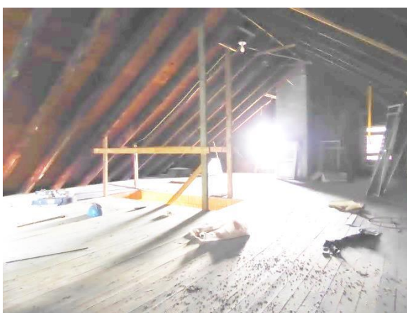
Attic (Room 301), looking southeast. Photo: HPTC, 06/08/17.
