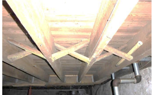
Exposed first-floor structural floor framing in Basement (Room 001) is a CDF. Photo: HPTC, 06/08/17.
