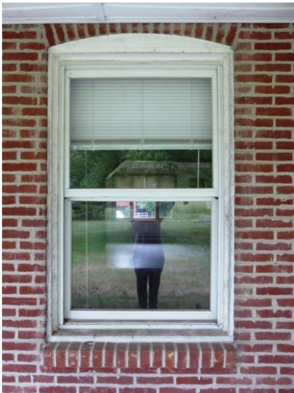
First-floor window opening, main block, east elevation. Photo: HPTC, 06/07/17.
