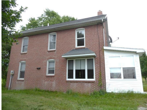
The west elevation. Photo: HPTC, 06/07/17.
