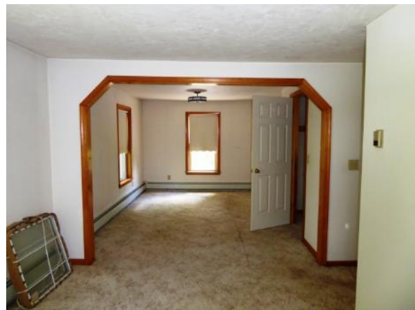
The loadbearing wall which bisects Rooms 201 has also been largely removed. Photo: HPTC, 06/08/17.
