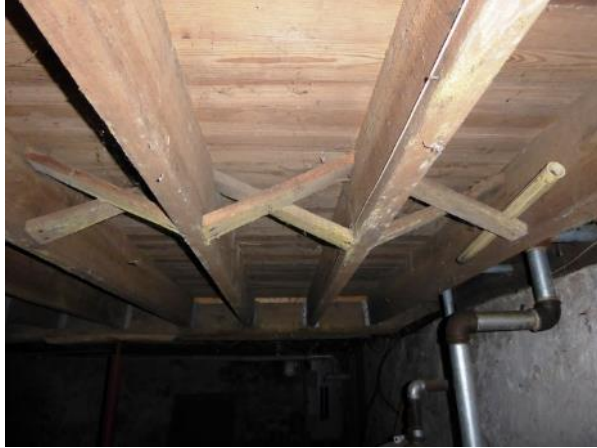
Cross bracing between joists. Photo: HPTC, 06/08/17.
