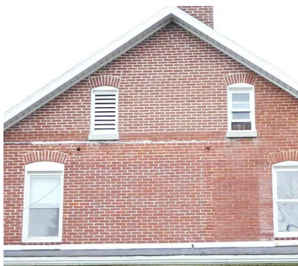
South elevation. The white line below the third-floor windows is likely a former roofline. W202 (at left in this photo) was likely a door. Photo: HPTC, 06/07/17.
