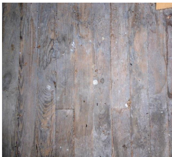
Historic wood flooring, Room 301. Photo: HPTC, 06/08/17.
