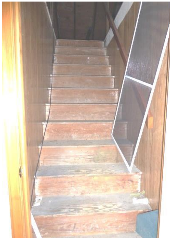
Attic stair, accessed from the second floor in Room 201. Photo: HPTC, 06/08/17.
