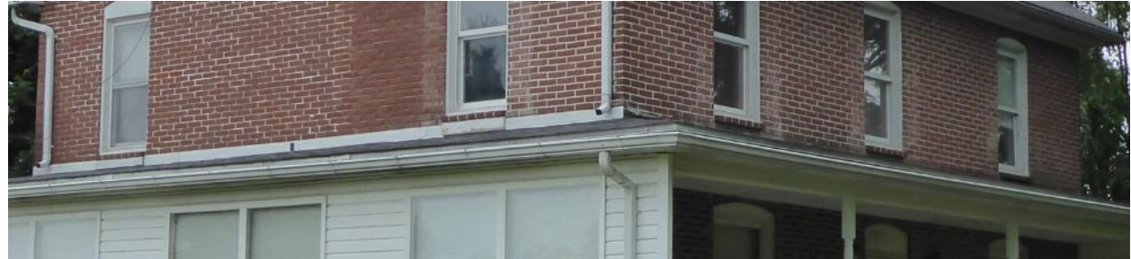
Sidewall trim over flashing on the east elevation of the main block is not extant. Photo: HPTC, 06/07/17.
