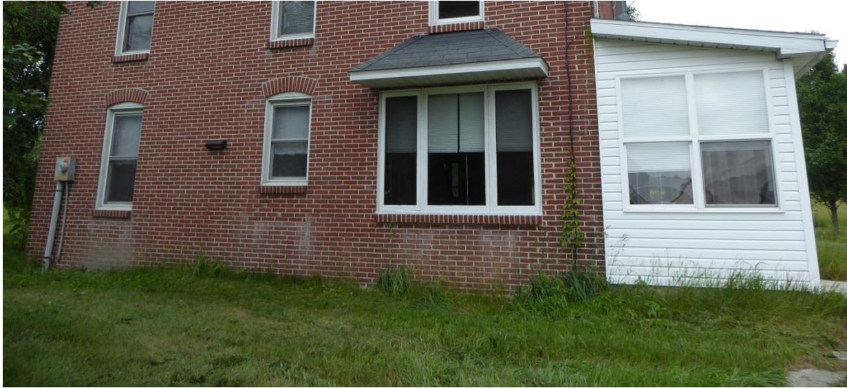
Most of the window openings on the west elevation first floor are not CDFs. From left: W107 is a CDF, modified window openings W106 and W105 are not CDFs, and modern opening W104 is not a CDF. None of the sash are CDFs. Photo: HPTC, 06/07/17.
