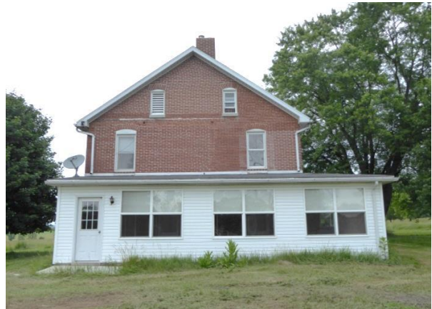
The south elevation. Photo: HPTC, 06/07/17.
