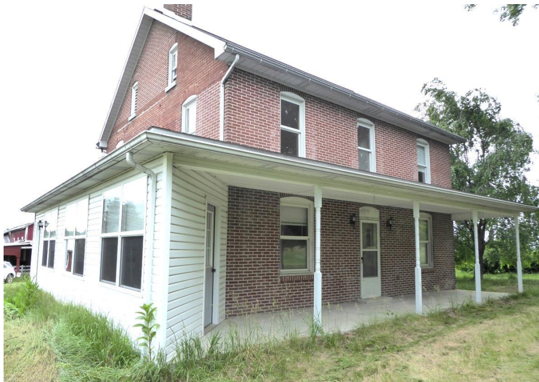
Brick on the main block, though not original to the house, is character defining because of its age. Modern vinyl trim on the sunroom/porch is not character defining. Photo: HPTC, 06/07/17.
