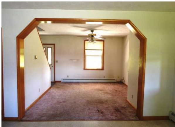
The loadbearing wall between rooms 102 and 105 has been largely removed. Photo: HPTC, 06/08/17.
