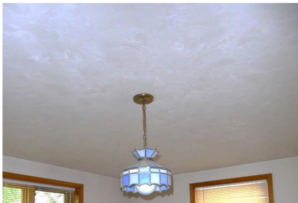
The majority of ceiling finishes are textured painted drywall, which is not a CDF. Photo: HPTC, 06/08/17.
