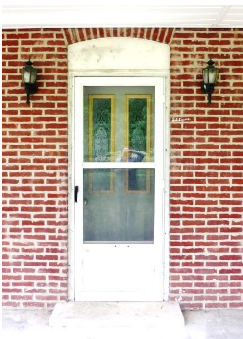
D103, exterior, with modern storm door. Photo: HPTC, 06/07/17.
