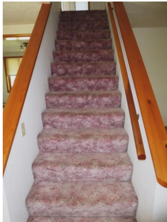
Load-bearing walls support the main stair. Photo: HPTC, 06/08/17.
