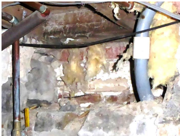
Former basement window opening on the west wall of Room 001 covered over with brick veneer. Photo: HPTC, 06/08/17.
