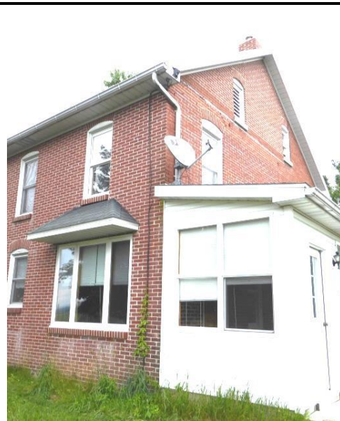
Eaves, soffits, and fascia—all modern—are not CDFs. Photo: HPTC, 06/07/17.
