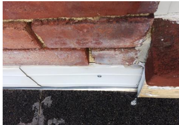
Sidewall flashing and trim, south elevation. Photo: HPTC, 06/21/17.
