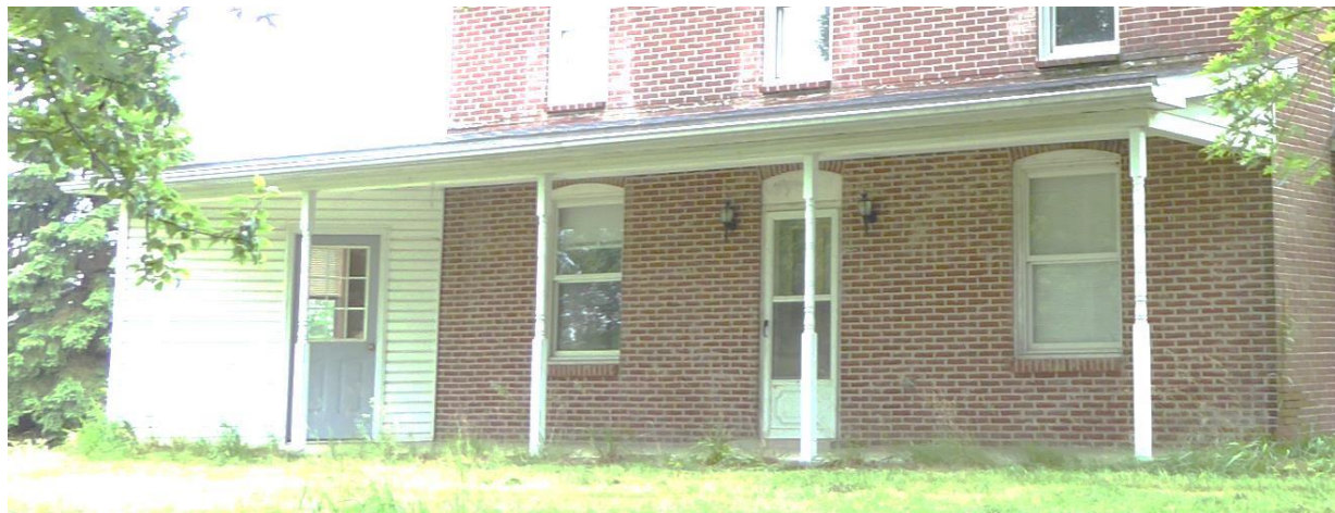
The east entry porch is modern and not a CDF. Photo: HPTC, 06/07/17.
