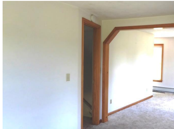
The majority of walls are painted drywall, which is not a CDF. Photo: HPTC, 06/08/17.
