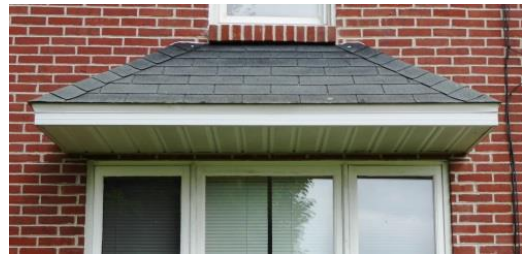
Roof projections over W105 (above) and W109 are not CDFs. Photo: HPTC, 06/07/17.
