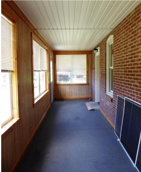
The first-floor south wall of the main block became an interior wall when the addition was constructed. The balloon-framed wall is veneered with brick. Photo: HPTC, 06/08/17.
