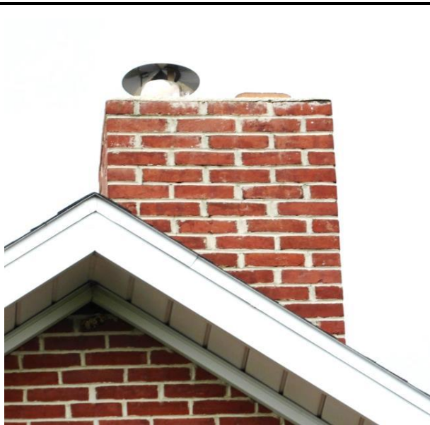
The main block chimney is not a CDF. Photo: HPTC, 06/07/17.
