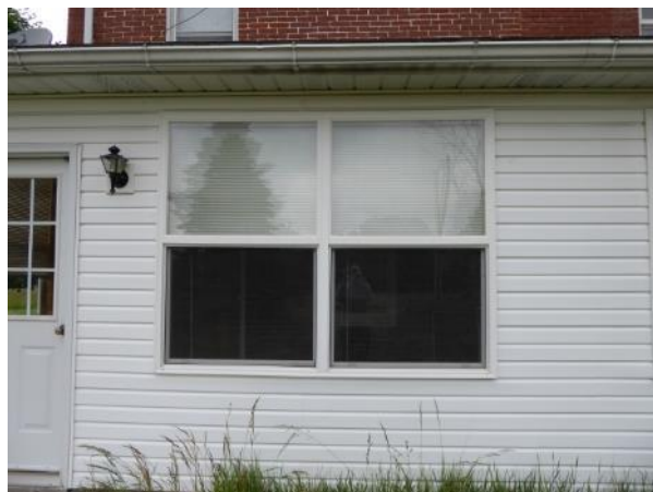
W103, exterior. Photo: HPTC, 06/07/17.
