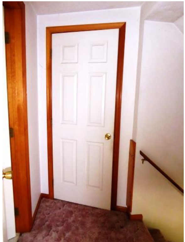
Interior doors are modern and not character defining. Photo: HPTC, 06/08/17.
