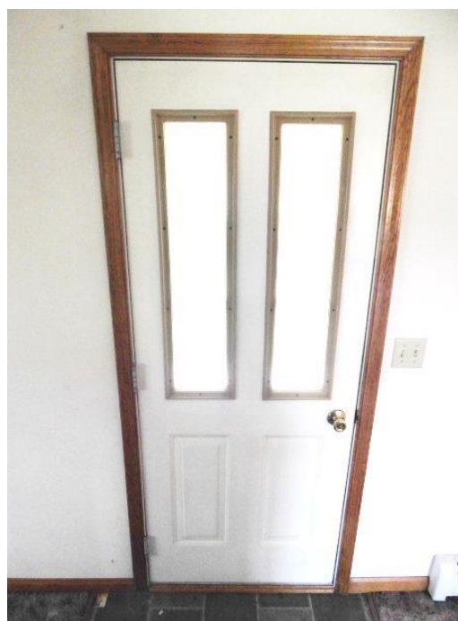
D103, interior. Photo: HPTC, 06/08/17.
