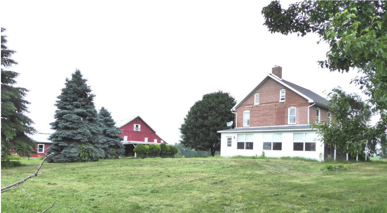
The house sits among agricultural fields, next to the historic bank barn. Photo: HPTC, 06/07/17.
