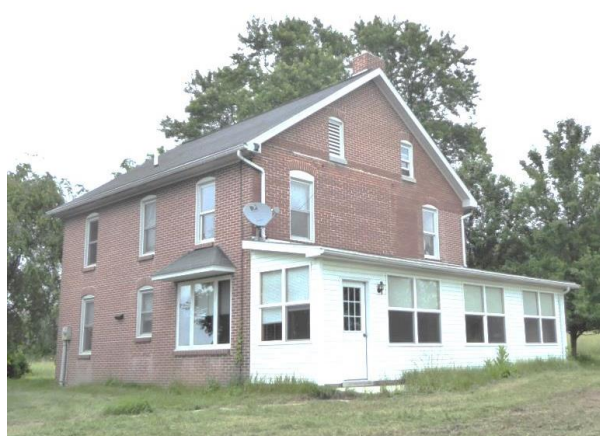
The west and north elevations. Modifications include roof covering, modern chimney, sunroom addition, modified window openings, and roof projection over W105. Photo: HPTC, 06/07/17.
