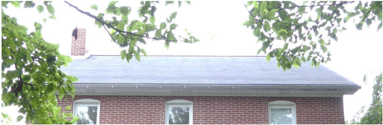
The main block's gable roof shape is character-defining. Asphalt shingle covering is not a CDF. Photo: HPTC, 06/07/17.
