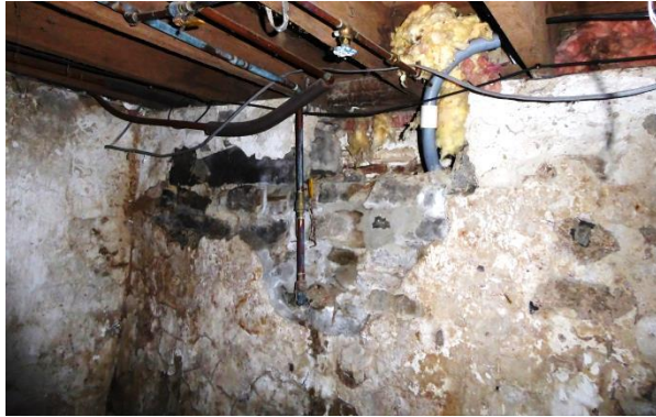
Foundation walls visible in Basement (Room 001) are a CDF. Concrete parging is likely historic. Photo: HPTC, 06/08/17.
