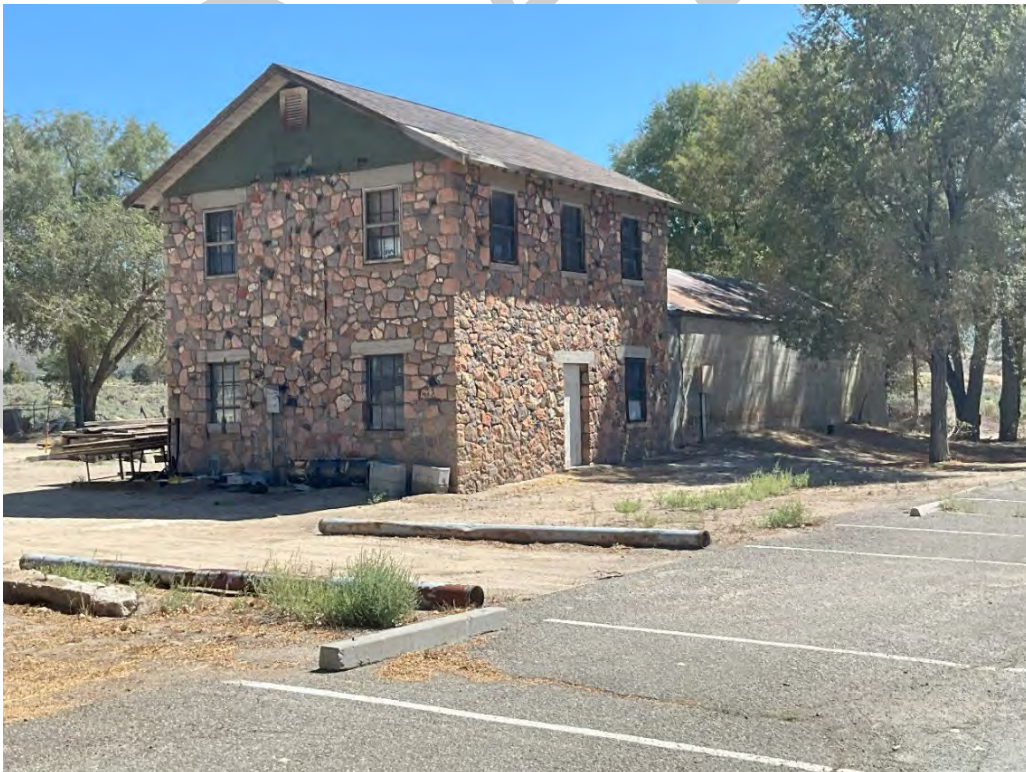
Photograph 54. Resource 96 (Filter Plant), oblique view, facing east. Nesta Anderson, August 2024.
