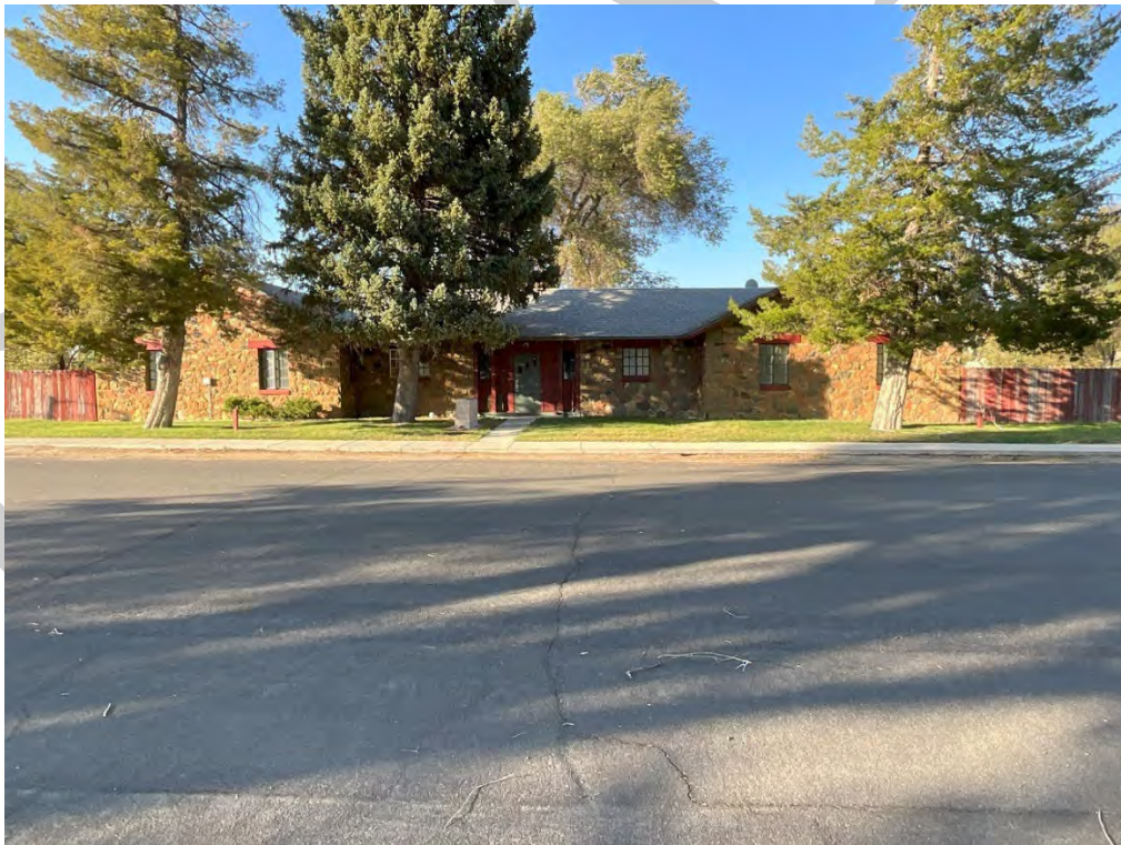
Photograph 40. Resource 57 (Quarters), view of northeast façade, facing southwest. Nesta Anderson, August 2024.
