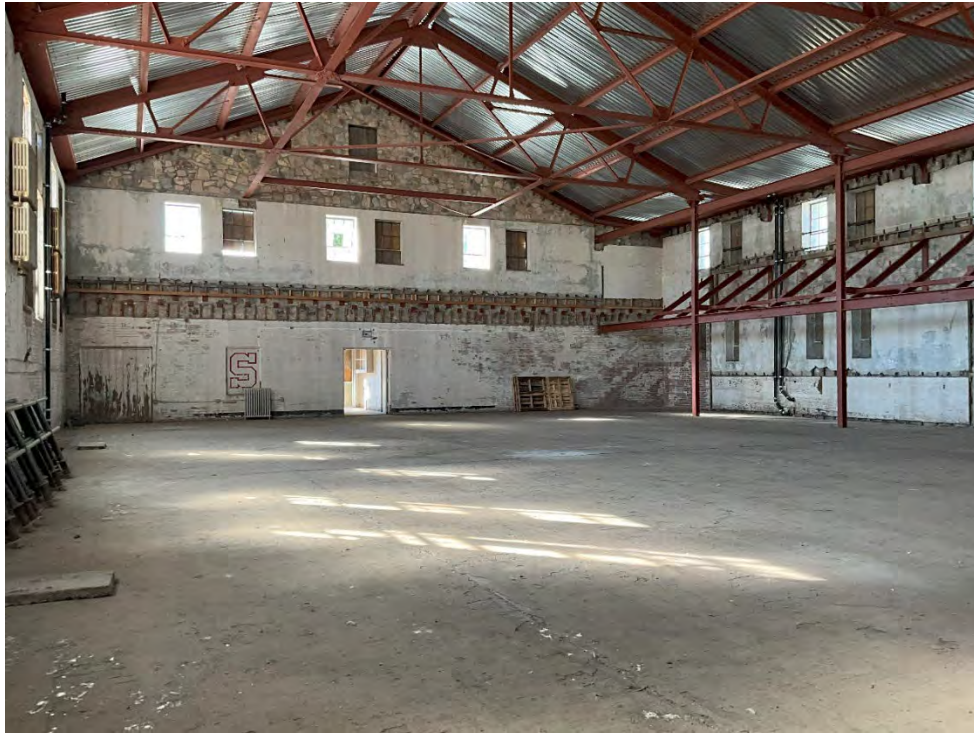
Photograph 23. Resource 20 (Gymnasium), interior overview of southeast end of building. Nesta Anderson, August 2024.
