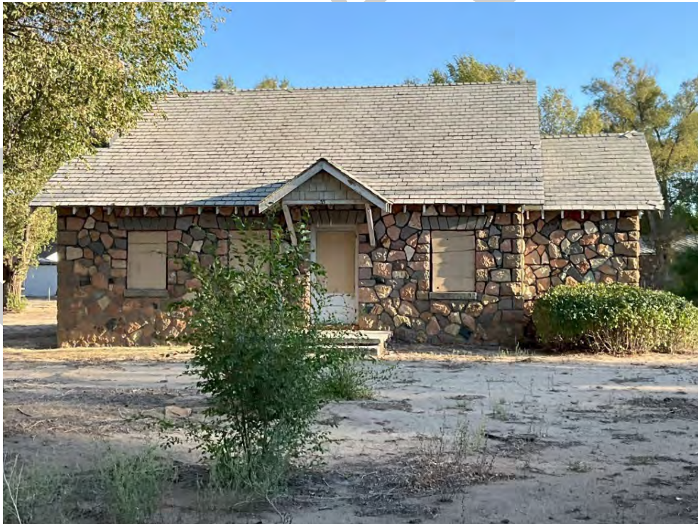
Photograph 32. Resource 35 (Cottage), view of north façade. Resource 36 (Cottage) is similar in appearance. Nesta Anderson, August 2024.
