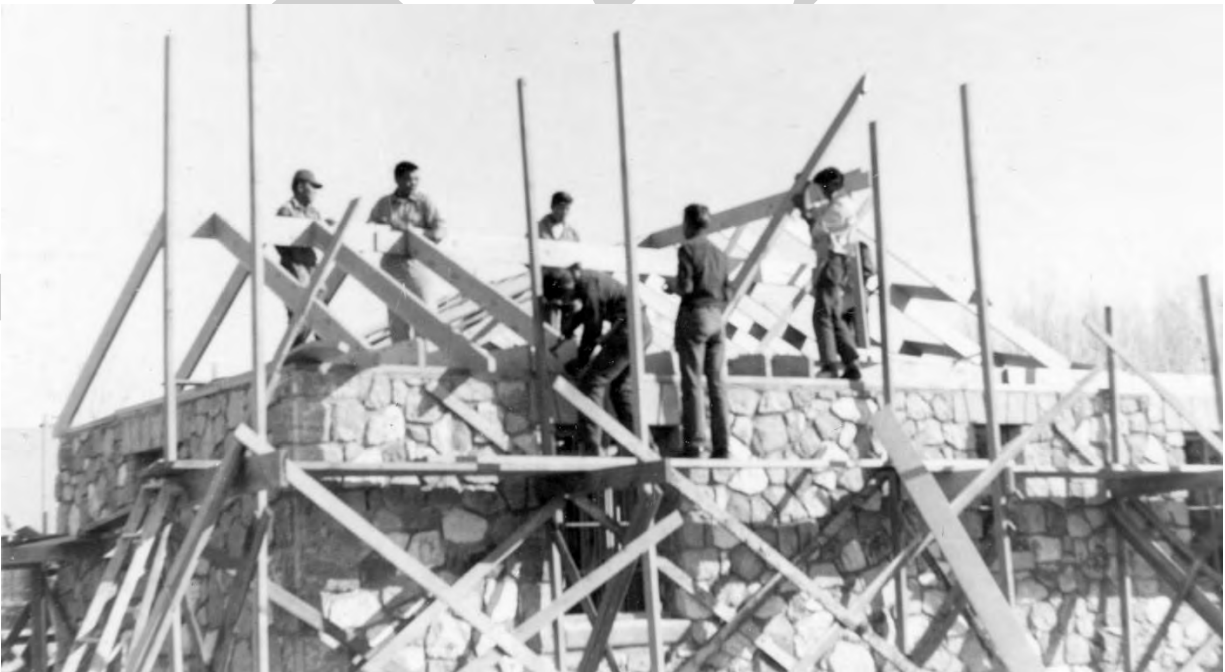
Figure 20. Students constructing stone cottage, 1956. Courtesy of Stewart Indian School Cultural Center & Museum (originally Hugh O. Tyler Collection).
