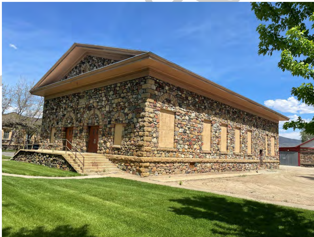
Photograph 50. Resource 90 (Auditorium), oblique view, facing northeast. Astrid Liverman, May 2026.
