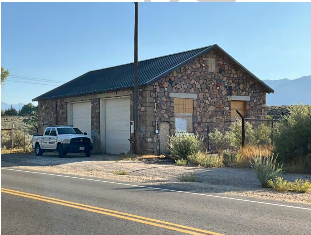
Photograph 75. Garage (outside nomination boundary), oblique view facing southwest, built 1940. Nesta Anderson, August 2024.
