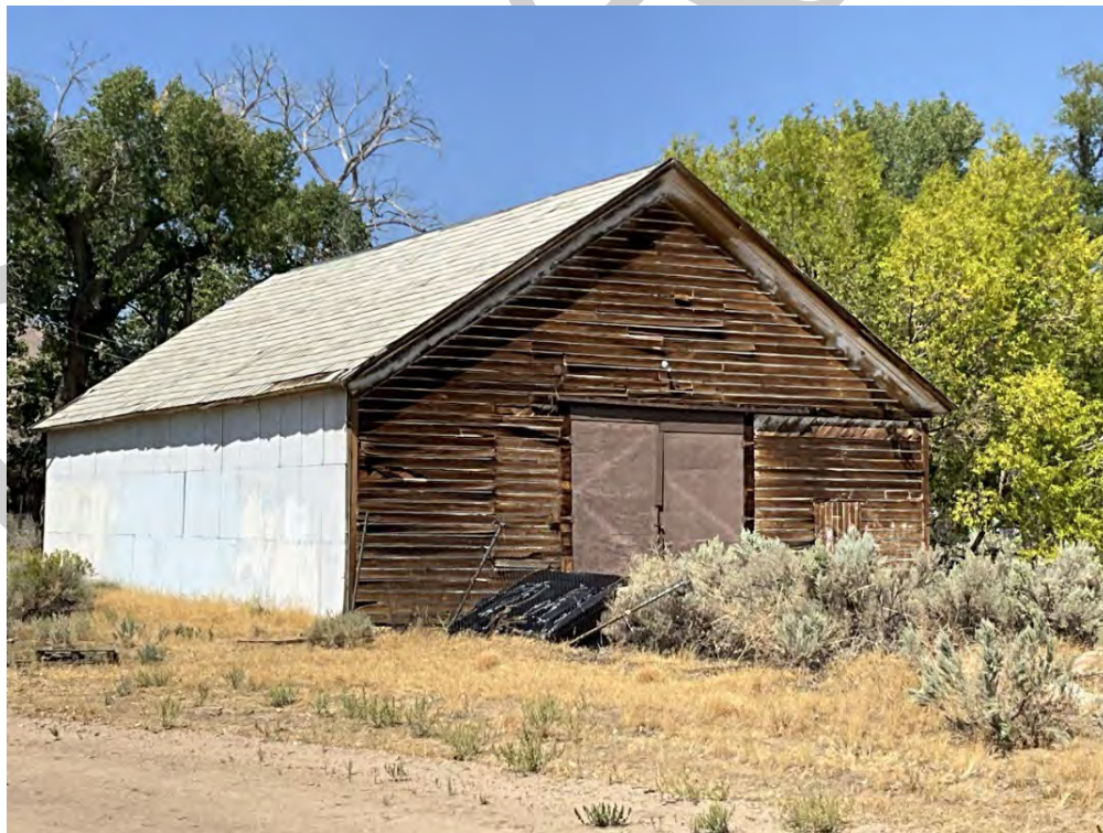
Photograph 46. Resource 70 (Blacksmith Shop), oblique view, facing northwest. Nesta Anderson, September 2025.
