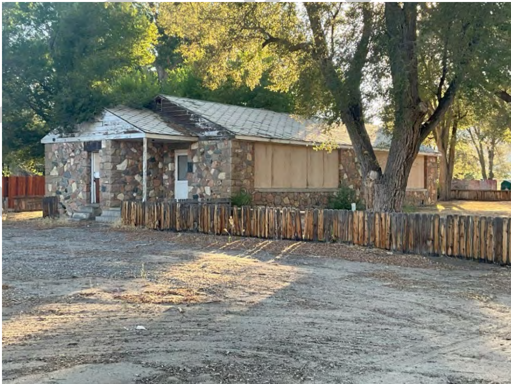
Photograph 42. Resource 61 (Duplex), oblique view, facing west. Nesta Anderson, August 2024.
