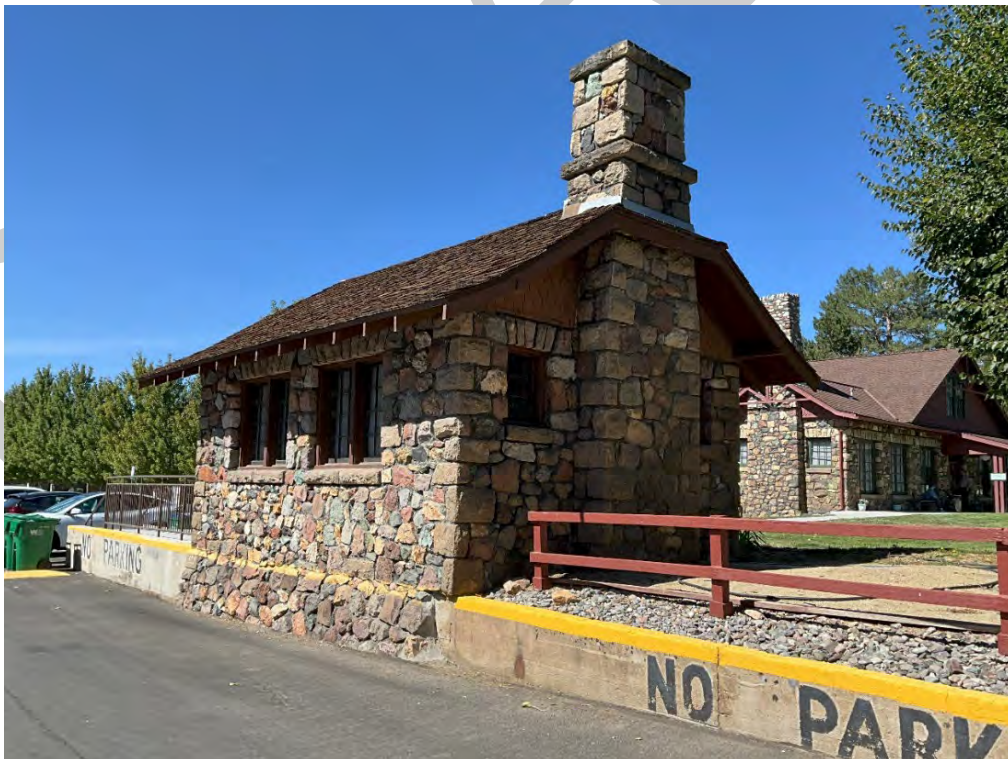
Photograph 6. Resource 2 (Post Office), oblique view, facing southwest. Nesta Anderson, August 2024.
