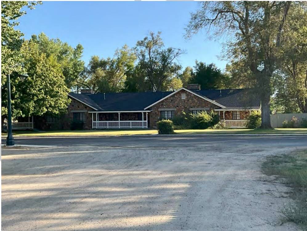
Photograph 44. Resource 67 (Four-plex), view of northeast façade, facing southwest. Nesta Anderson, August 2024.
