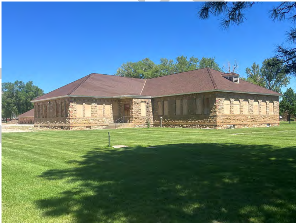
Photograph 16. Resource 15 (Kitchen and Dining Hall), oblique view, facing northwest. Lisa Davidson, May 2026.
