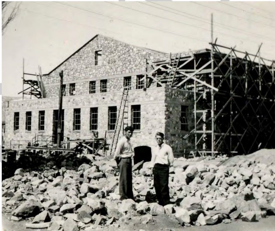
Figure 18. Resource 20 (Gymnasium) under construction, ca. 1938. Photo courtesy of Stewart Indian School Cultural Center & Museum.
