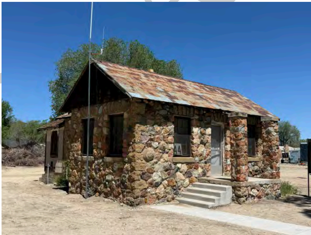
Photograph 34. Resource 44 (Cottage), view of east façade. Astrid Liverman, May 2024.
