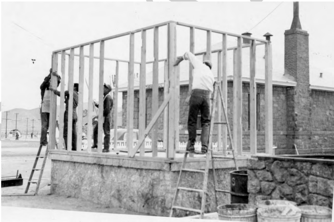
Figure 22. Students engaging in construction on the small foundation (still extant) located between the Bakery (Resource 19) and Kitchen and Dining Hall (Resource 15), undated photograph (post-1942). Note Quonset hut visible in the background located due south of Stewart Infirmary postdates 1941. Courtesy of Stewart Indian School Cultural Center & Museum.
