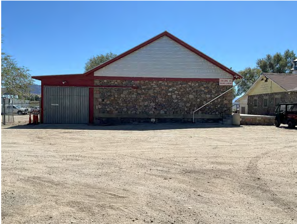
Photograph 47. Resource 84 (Shop Building), view of northwest side, facing southeast. Nesta Anderson, August 2024.
