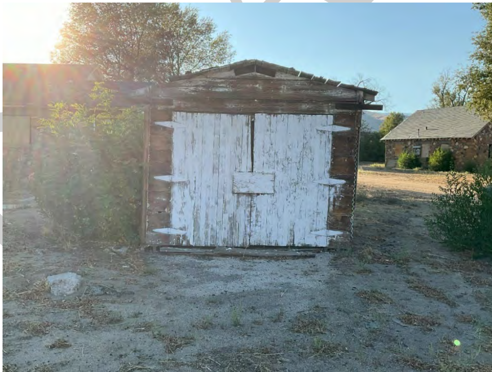
Photograph 62. Resource 165 (Shed/garage), view of east side, facing northwest. Nesta Anderson, August 2024.
