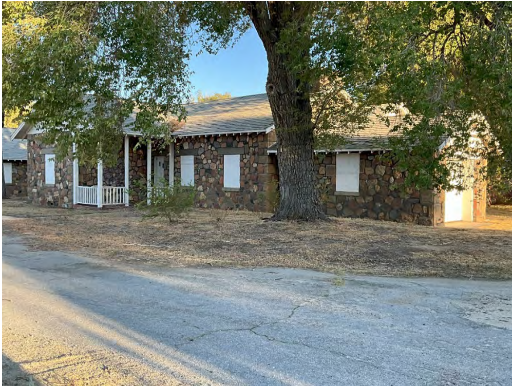
Photograph 29. Resource 31 (Cottage), oblique view, facing southeast. Nesta Anderson, August 2024.
