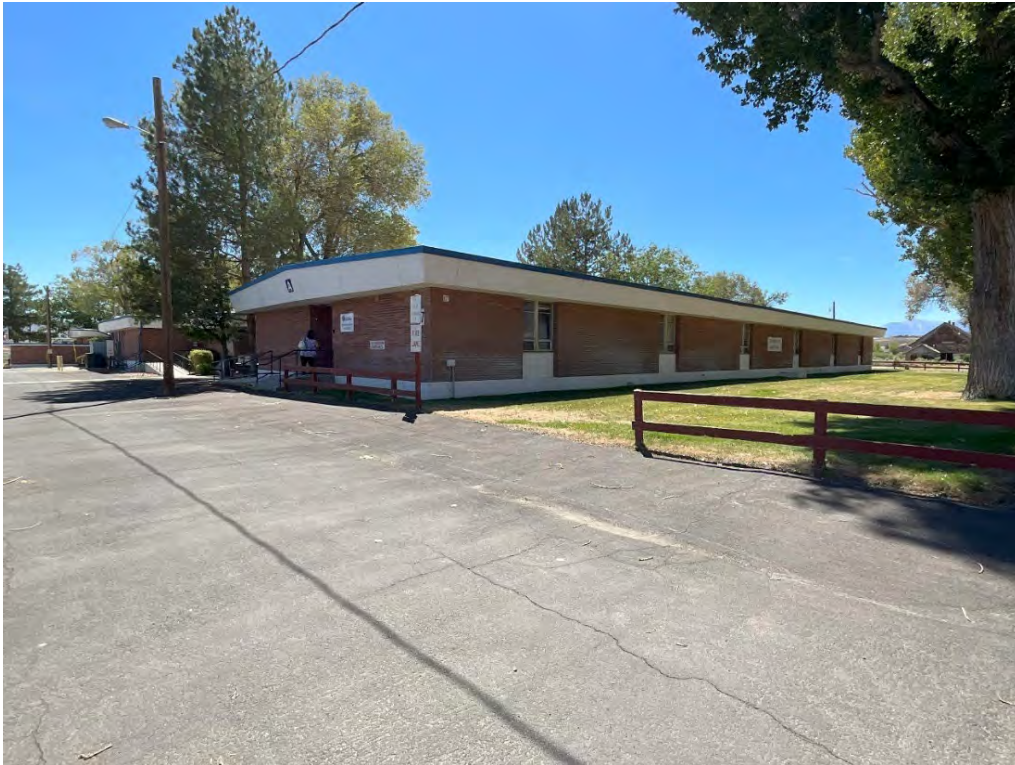
Photograph 55. Resource 107 (Nunez Lodge), oblique view, facing southeast. Nesta Anderson, August 2024.
