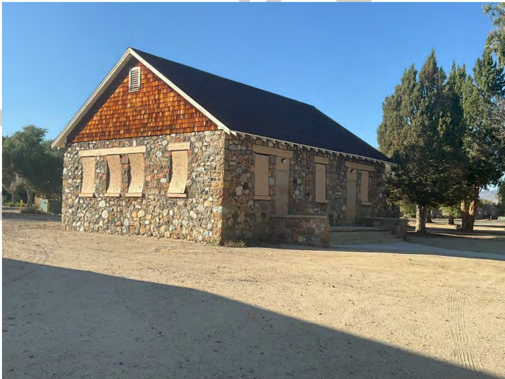
Photograph 36. Resource 46 (Sewing Room), view of east façade. Nesta Anderson, August 2024.
