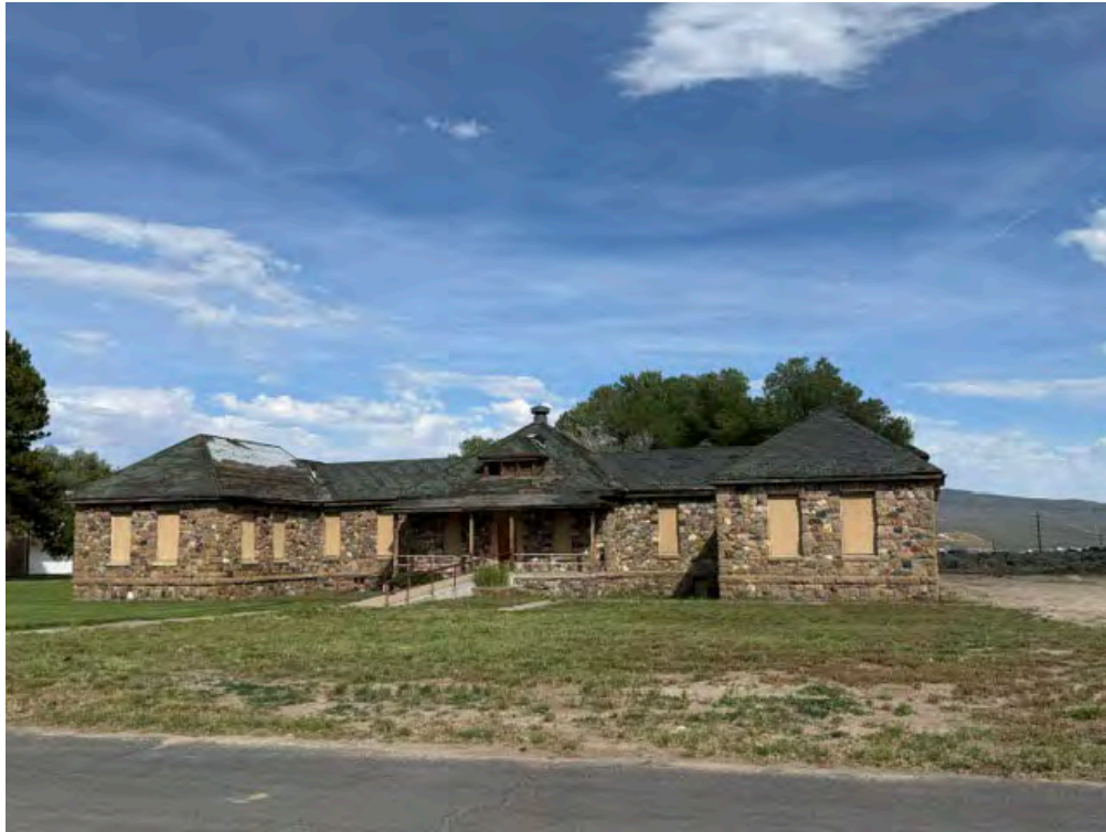
Photograph 61. Resource 162 (Student Infirmary), west façade along Jacobsen Way. Astrid Liverman, May 2026.
