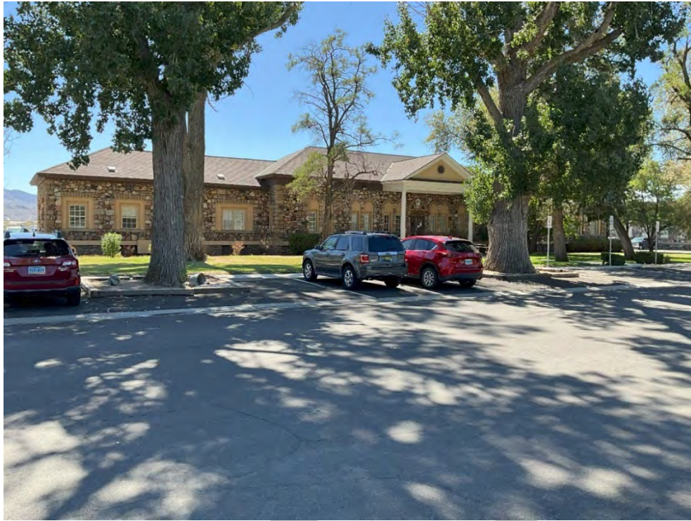
Photograph 49. Resource 89 (Boys' Dormitory), view of east façade, facing west. Nesta Anderson, August 2024.
