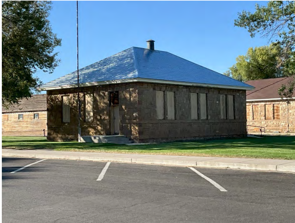
Photograph 21. Resource 19 (Bakery), oblique view, facing northwest. Nesta Anderson, August 2024.
