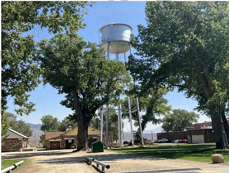
Photograph 48. Resource 87 (Water Tank), overall view facing southeast. Nesta Anderson, September 2025.
