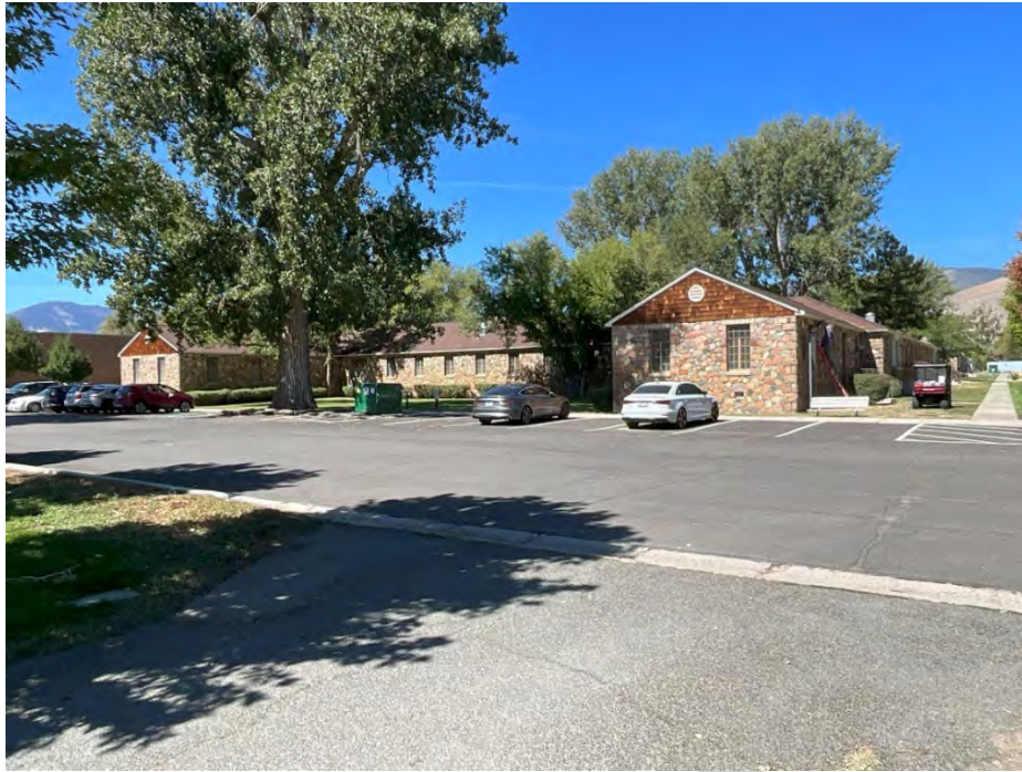
Photograph 13. Resource 13 (Girls' Dormitory), oblique view, facing southwest. Resource 12 (Girls' Dormitory, "La Manzanita," is similar in appearance. Nesta Anderson, August 2024.
