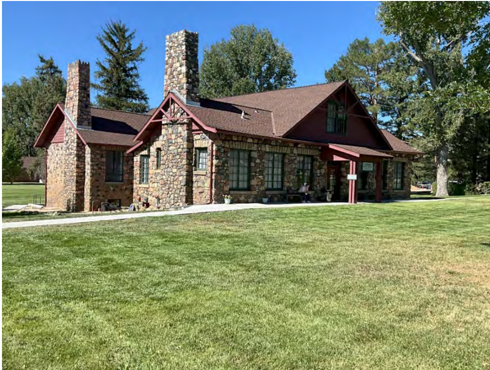
Photograph 5. Resource 1 (Administration Building), oblique view facing southwest. Nesta Anderson, August 2024.
