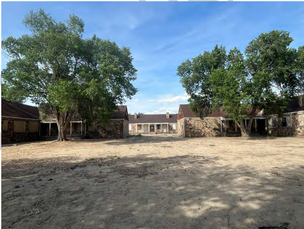
Photograph 24. Overview, Resources 22-25 (Sierra Lodge Dormitories) from interior courtyard, facing northeast. Lisa Davidson, May August 2026.
