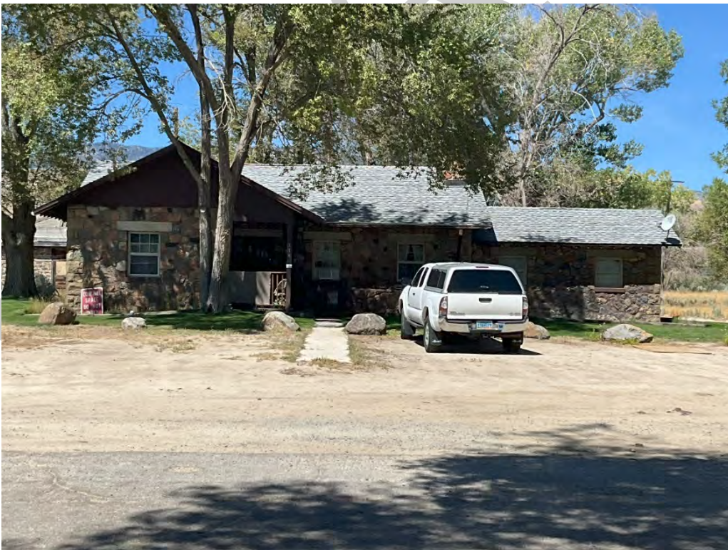
Photograph 56. Resource 110 (Cottage), view of east façade, facing northwest. Nesta Anderson, August 2024.
