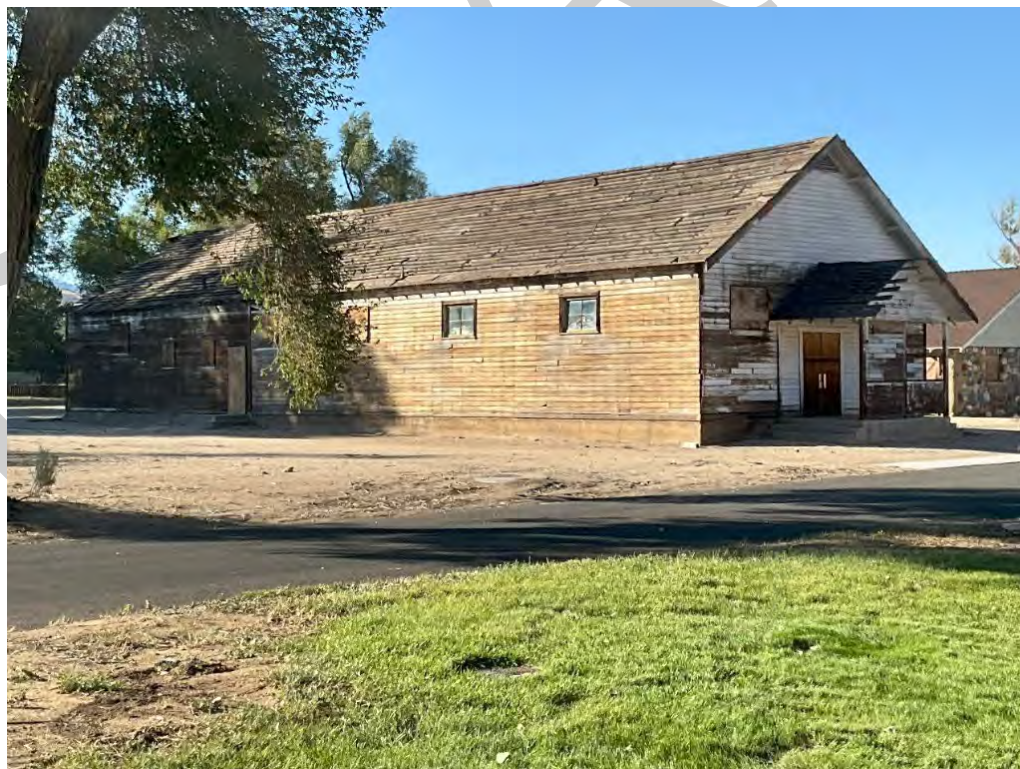
Photograph 38. Resource 48 (Commissary), oblique view of east façade. Nesta Anderson, August 2024.
