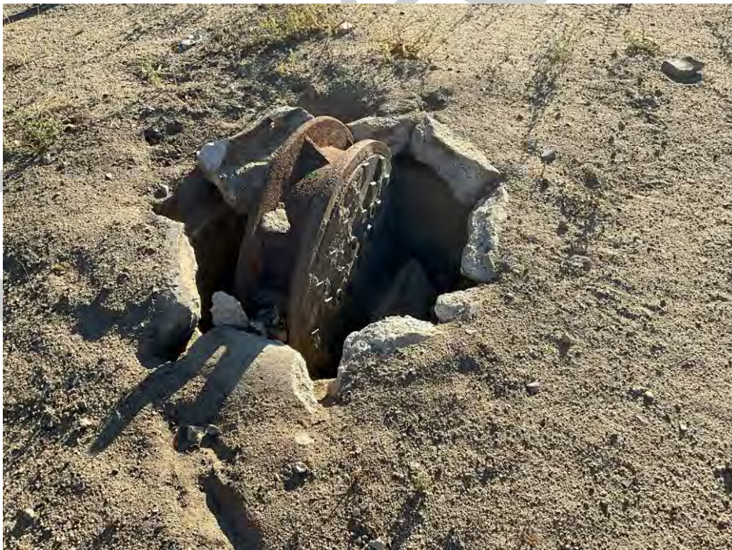
Photograph 70. Steam Tunnels, representative aboveground feature. Nesta Anderson, August 2024.
