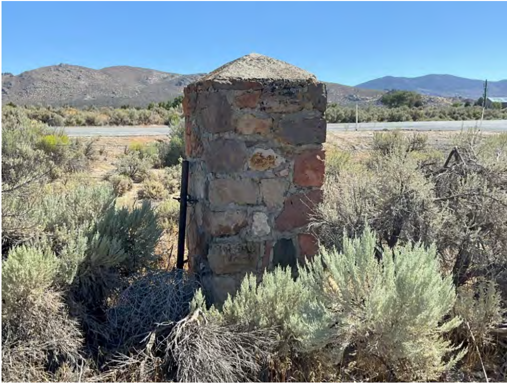
Photograph 65. Resource 169 (Fence Posts), northeast edge of property, facing northeast. Other individual piers on the campus perimeter are comparable in appearance. Nesta Anderson, August 2024.
