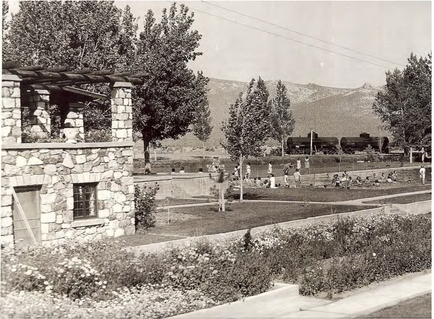
Figure 15. View of swimming pool originally north of the Administration Building (Resource 1) and formal plantings, with Superintendent's Cottage (Resource 3) at left, undated photograph (ca. 1935). View also shows Virginia & Truckee rail line in background running at the approximate location of Snyder Avenue and Bigelow Drive. Courtesy of Stewart Indian School Cultural Center & Museum.
