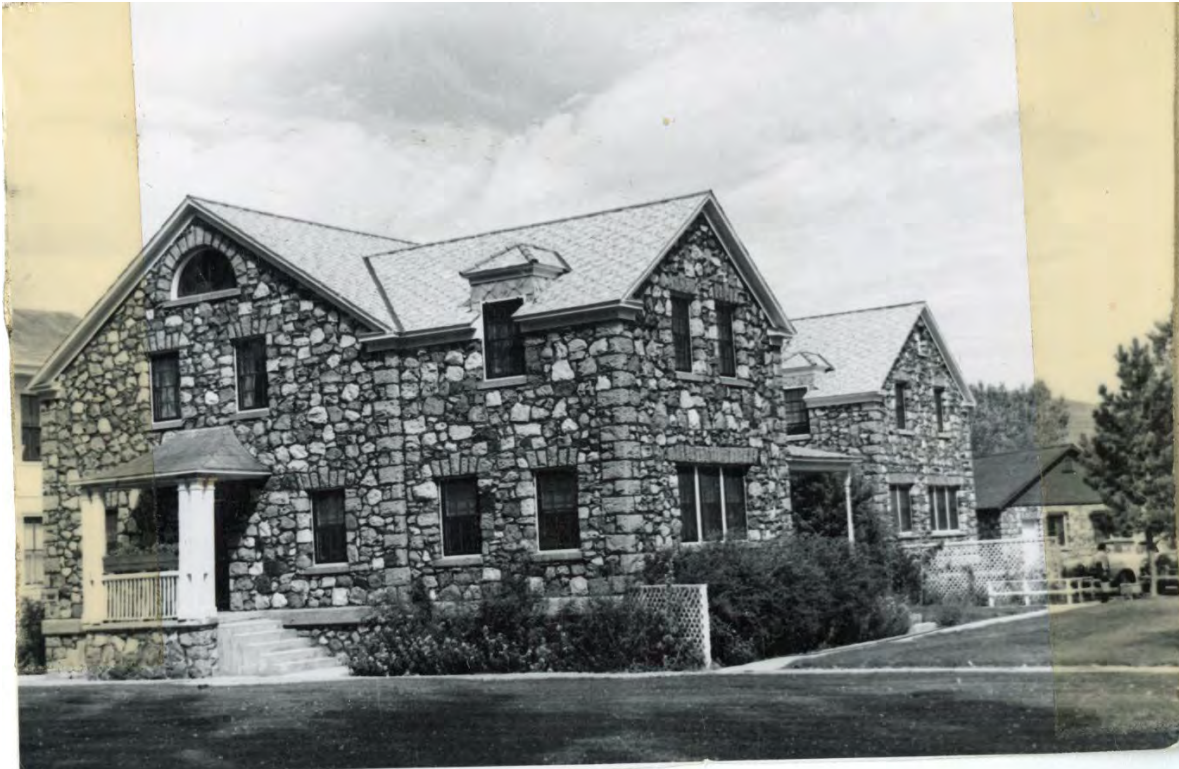
Figure 28. Home Economics Building, Jacobsen Way (demolished ca. 1972), undated photograph. Courtesy of Stewart Indian School Cultural Center & Museum.
