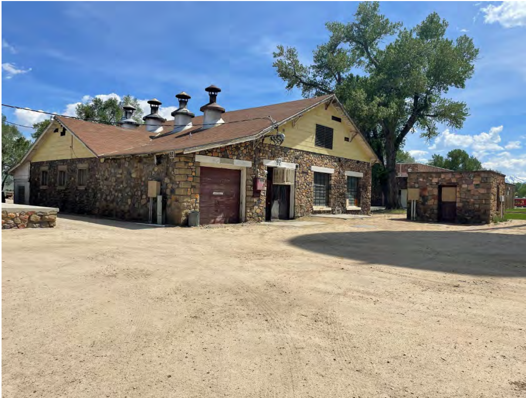
Photograph 53. Resource 92 (Boiler House) and Resource 94 (Pump House) (at right), facing southeast. Astrid Liverman, May 2026.
