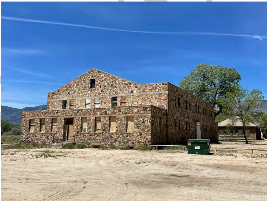
Photograph 22. Resource 20 (Gymnasium), oblique view, facing southwest. Astrid Liverman, May 2026.
