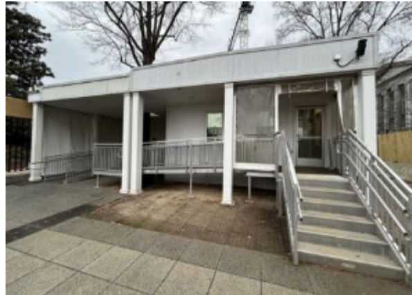
Figure 3: View of a Temporary Visitor Screening Trailer Entrance on East Executive Avenue
