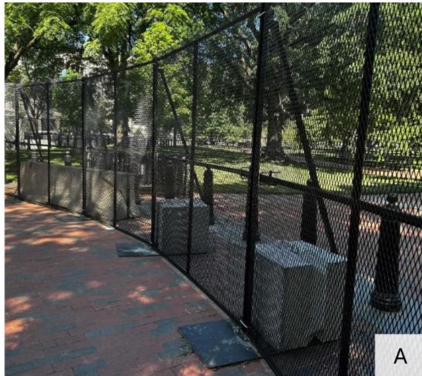
Anti-scale fencing on H Street NW, June 2026
