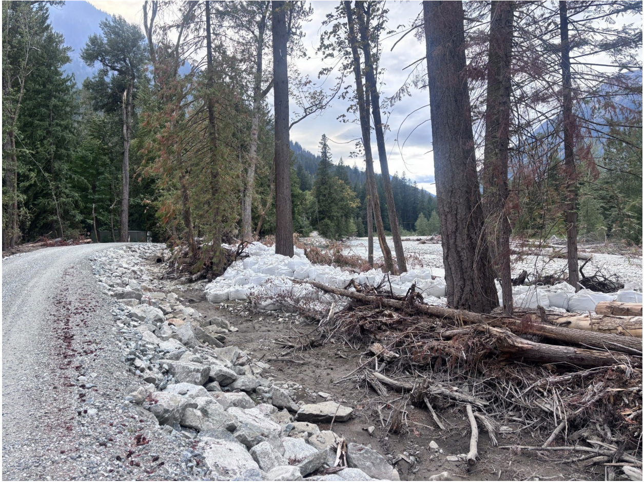
Figure 6. Approximate location where proposed Chelan County Road segment will tie in with the existing NPS temporary road (looking west). Note Supersacks.
