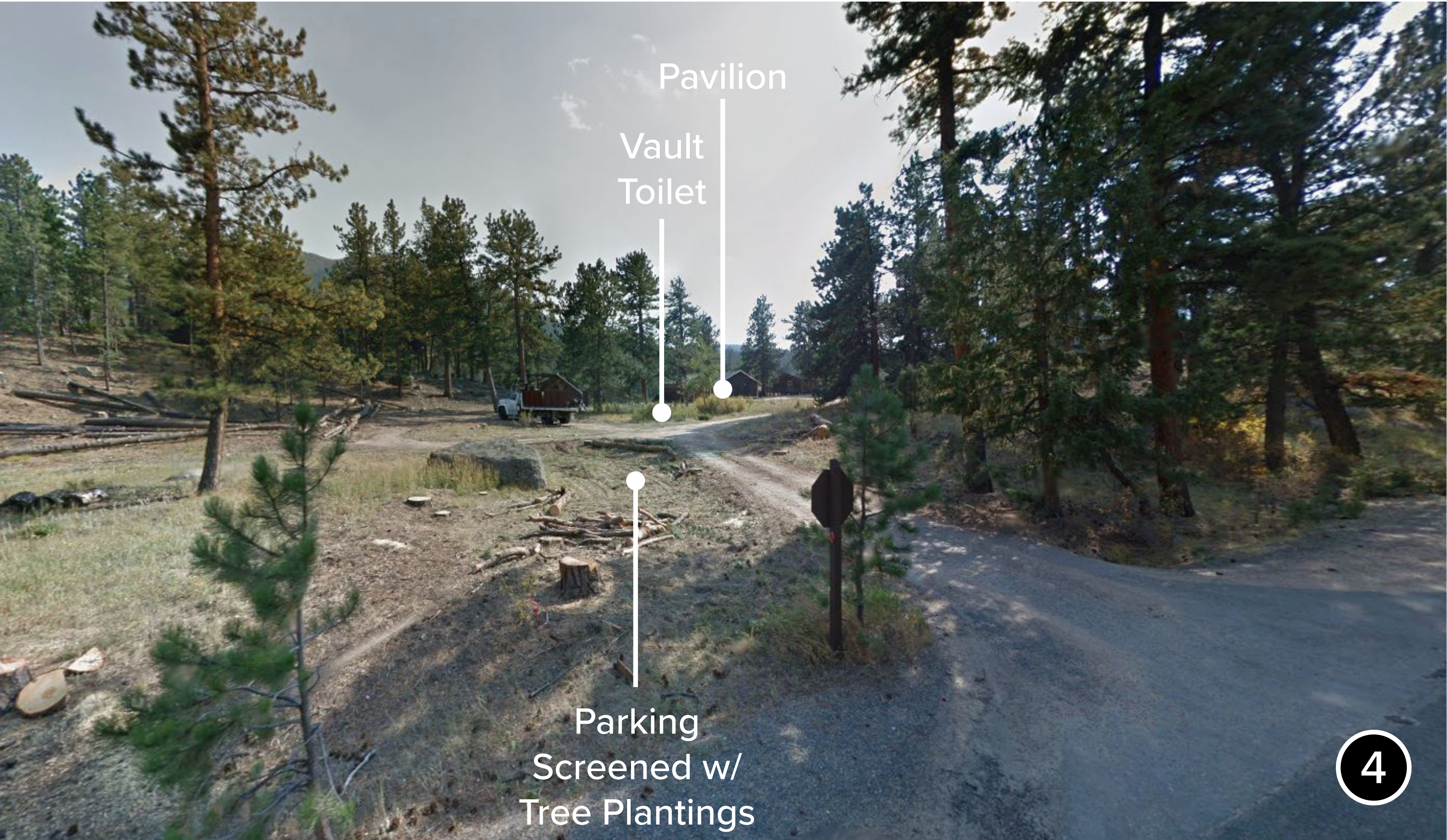
East Entrance - Looking West
