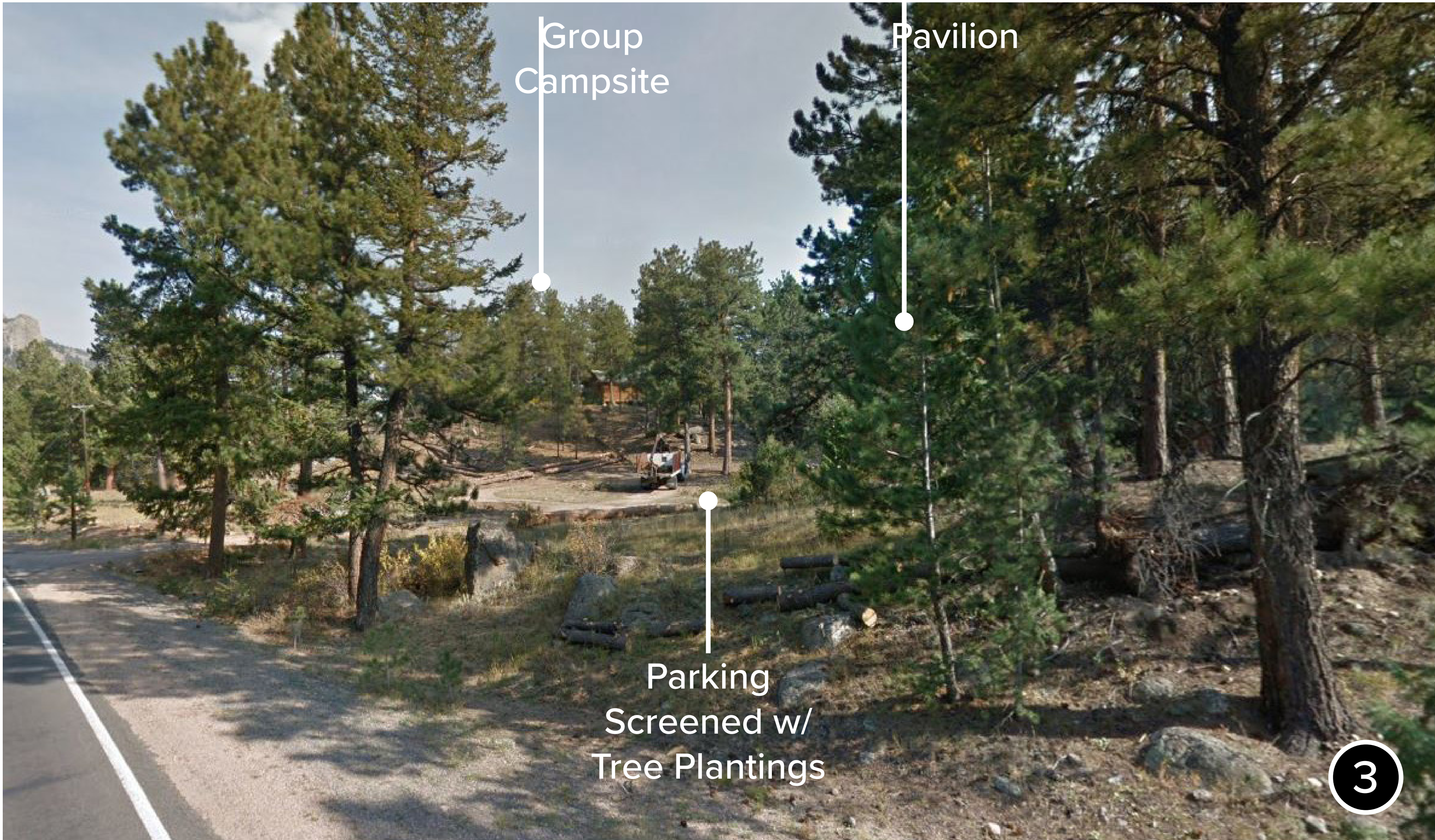
East Entrance - Looking East
