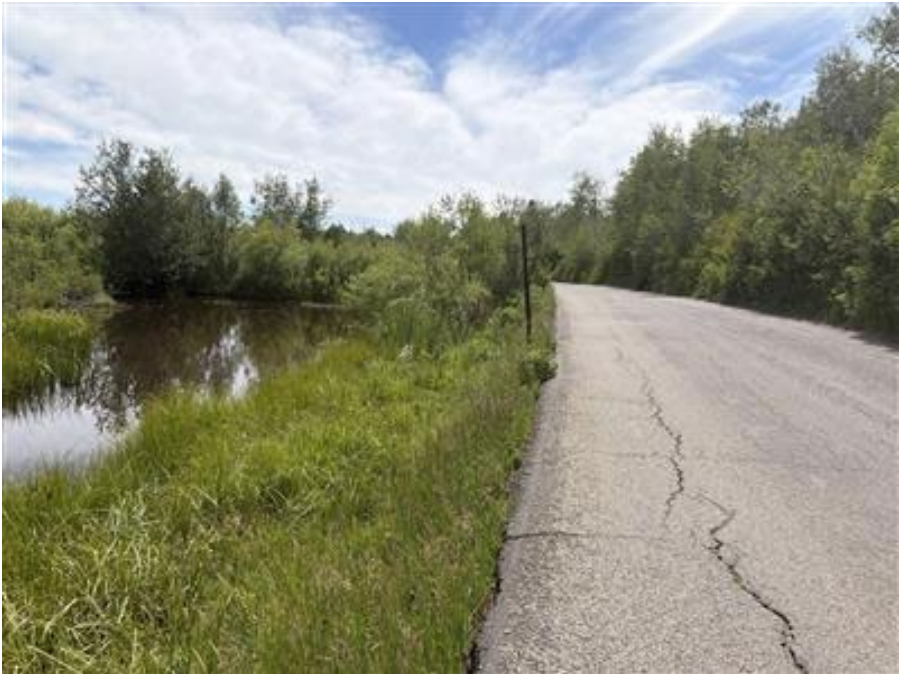
Photo B-1. Existing road and wetland complex boundary in the vicinity of Cross-Section 1, view is to the southwest.
