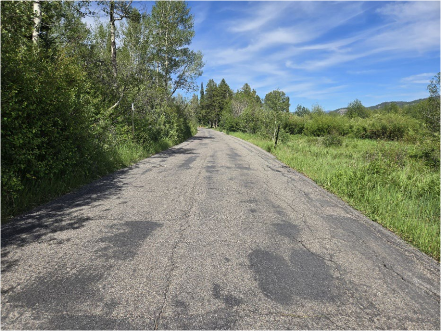
Photo B-2. Existing road and wetland complex boundary in the vicinity of Cross-Section 2, view is to the northeast.
