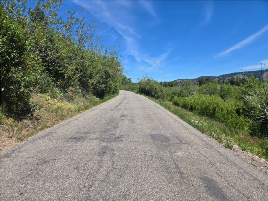
Photo B-3. Existing road and wetland complex boundary in the vicinity of Cross-Section 3, view is to the northeast.
