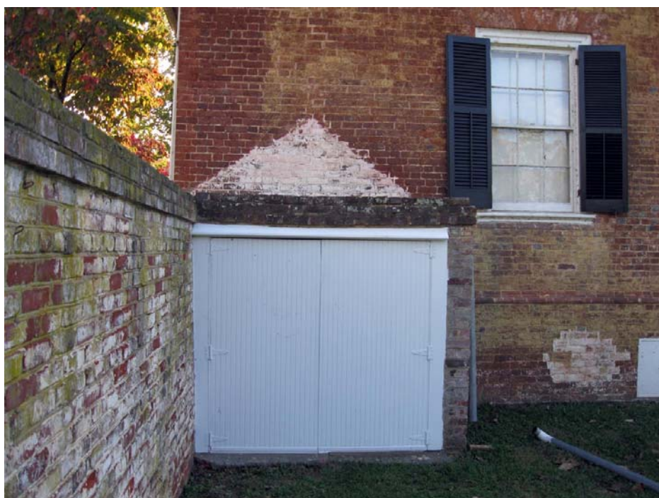
Current view of northern basement stairway entrance. Garden wall added in 1920s. Note ghost lines for pitched roof on wall of the house. The park proposes to reconstruct the missing roof.
