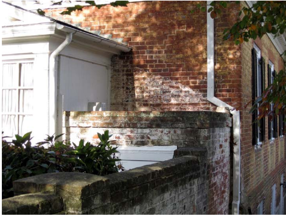
Current view northern basement stairway entrance. Garden wall added in 1920s. Note ghost lines for pitched roof on wall of the house. The park proposes to reconstruct the missing roof.
