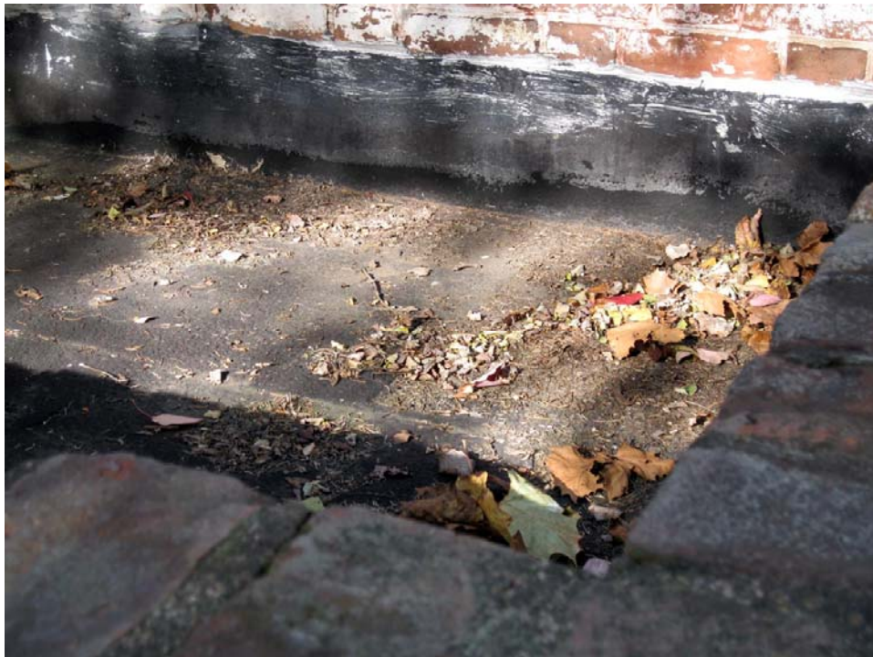
Current view of the flat roof on the southern basement stairway entrance. This area fills with rainwater that eventually seeps into the basement.
