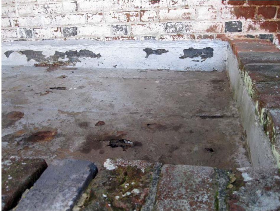
Current view of the flat roof on the northern basement stairway entrance. This area fills with rainwater that eventually seeps into the basement.
