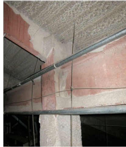
Deteriorated condition of fireproofing at column/beam in the hotel attic space. Hornberger + Worstell Photo
