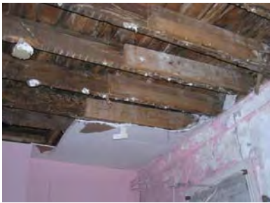
Figure 4-047: Sistered floor joists visible from first floor. (RSA, 2006)
