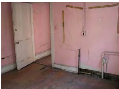
Figure 4-055: Room 208 - Floor sagging below east wall. (RSA, 2006)
