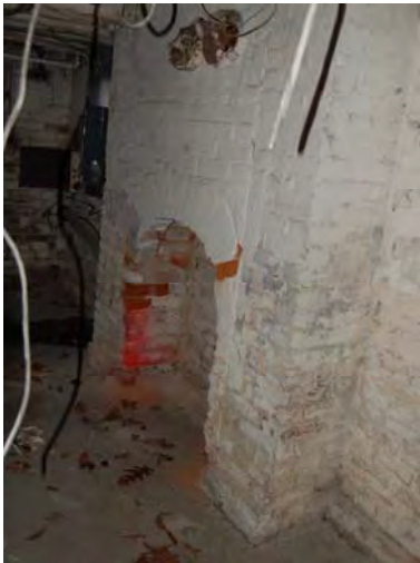
Figure 3-114: East fireplace piers at south wall. (Photo: BBB, 2007)
