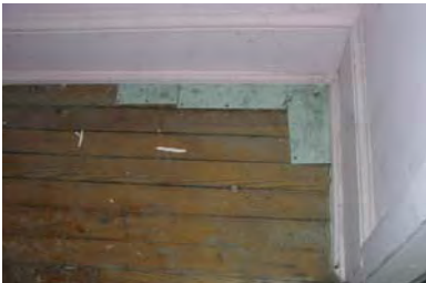
Figure 3-406: 2 1/4 Strip flooring and floor patches. (Photo: BBB, 2007)
