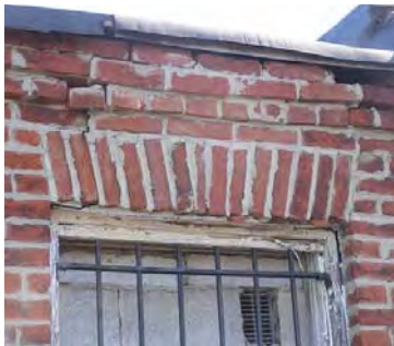
Figure 4-031: Brick masonry shifting above flat arch and interior lintel of window W304. (RSA, 2006)
