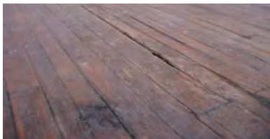
Figure 3-466: Separating at wood floor. (Photo: BBB, 2007)
