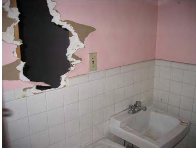
Figure 3-227: Hold in GWB at west wall. (Photo: BBB, 2007)
