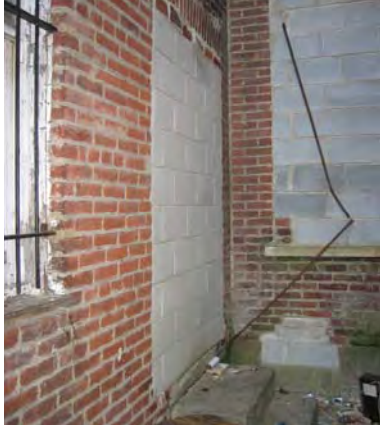
Figure 3-060: Door D103A with CMU infill. (Photo: BBB, 2007)
