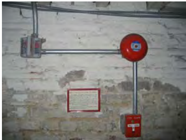
Figure 4-094: Fire alarm system. (Photo: GHT, 2006)
