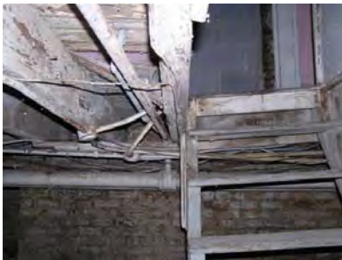
Figure 4-041: Sagging at stairs. (RSA, 2006)
