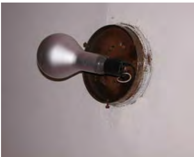
Figure 3-153: Incandescent ceiling light fixtures. (Photos: BBB 2006)
