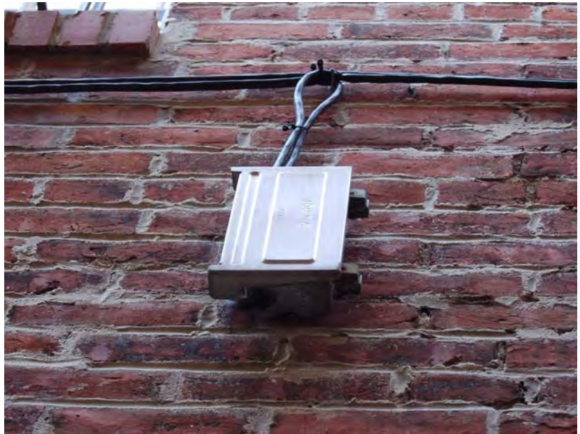
Figure 3-066: Surface mounted telephone box and cable. (Photo: BBB, 2007)
