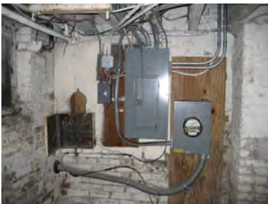
Figure 4-081: Electrical panels and electric meter in the basement. (Photo: GHT, 2006)
