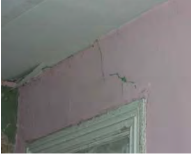
Figure 3-420: Plaster damage above W210. (Photo: BBB, 2007)
