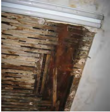
Figure 3-192: Break in lath at ceiling showing where north wing wall once was. (Photo: BBB, 2006)
