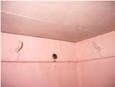
Figure 3-487: Underside of shelf with missing hook exposing stained finish. (Photo: BBB, 2007)
