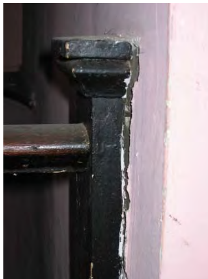
Figure 3-523: Pilaster detail showing cut nail anchor. (Photo: BBB, 2006)
