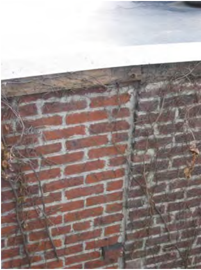
Figure 2-020: View of joint showing end of Period 1 two-story structure on the left and beginning of Period 2 two-story structure on right. (Photo: BBB, 2006)
