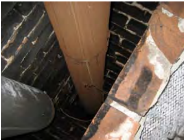
Figure 4-077: Metal tubes in flue as evidence of early duct work. (Photo: GHT, 2007)
