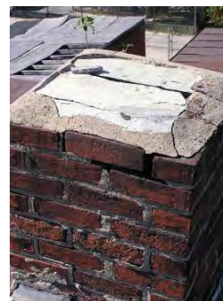
Figure 4-033: Masonry deterioration at chimneys. (RSA, 2006)
