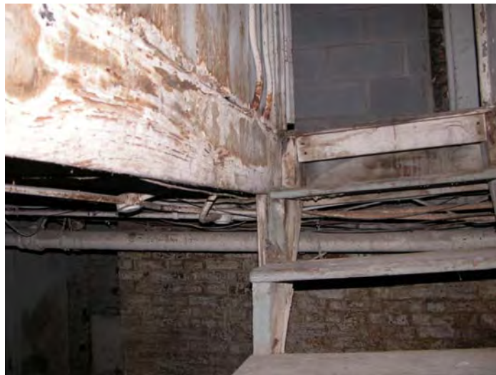
Figure 3-129: Termite damage at stair opening framing. (Photo: BBB, 2007)
