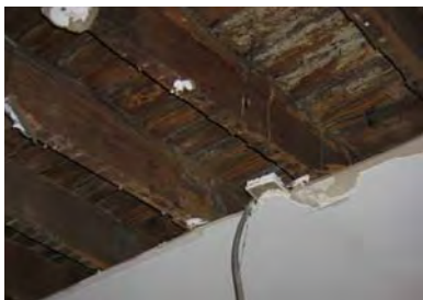
Figure 3-271: Second floor joists with exposed underside of original tongue and groove flooring. (Photo: BBB, 2007)
