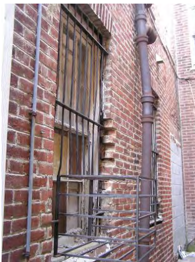
Figure 4-027: Spalling brick at first floor south wall window. (RSA, 2006)
