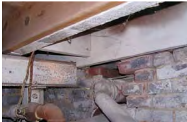
Figure 4-035: Steel beam not bearing on brick as it should. (RSA, 2006)
