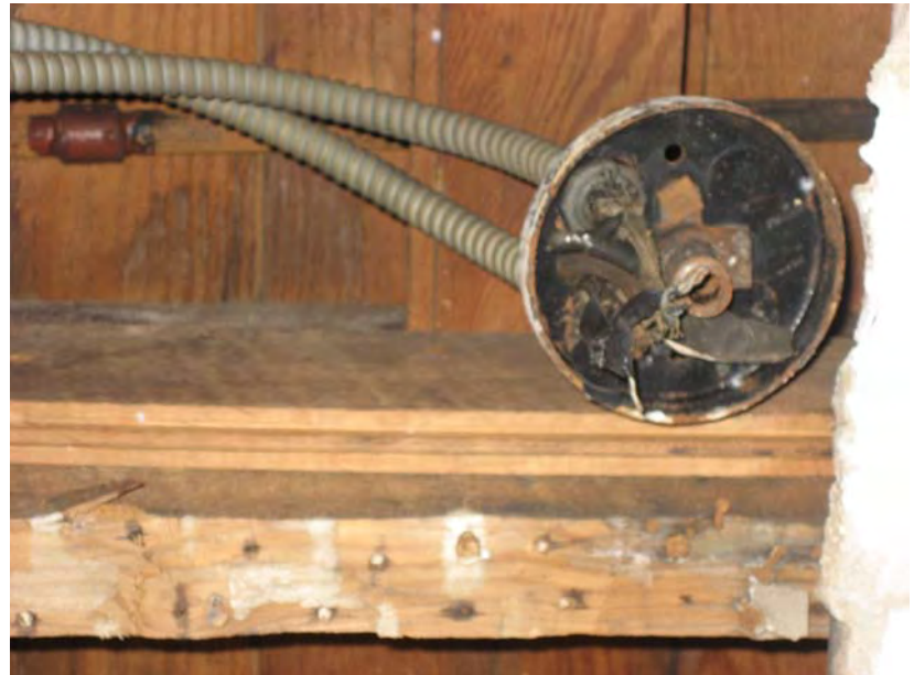
Figure 4-086: Retrofitted junction box at ceiling of second floor. (Photo: GHT, 2007)
