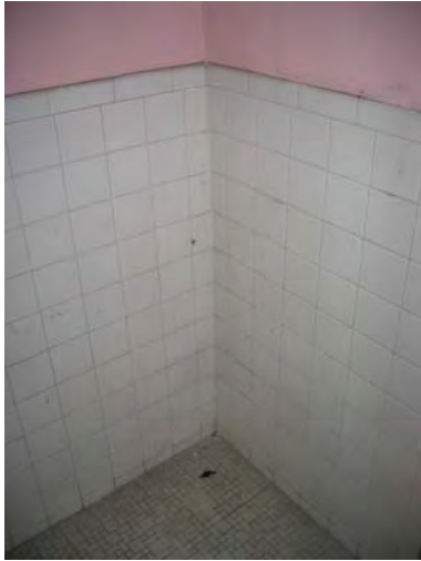
Figure 3-226: Ceramic wall tile. (Photo: BBB, 2007)
