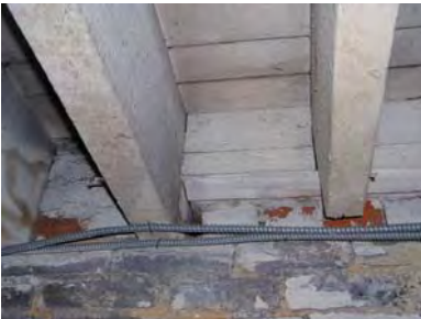
Figure 4-044: Header corresponding to party wall chimneys – splitting at north wall header. (RSA, 2006)
