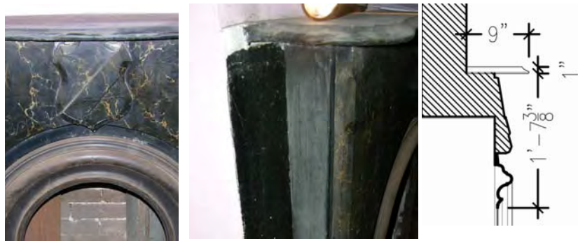
Figure 3-202: Fireplace mantel and face detail and side elevation photos and profile. (Photos: BBB, 2006)
