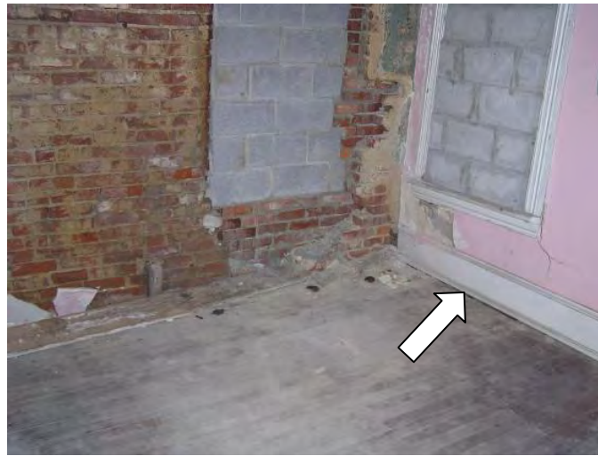
Figure 4-053: Room 210 - Floor sagging. (RSA, 2006)
