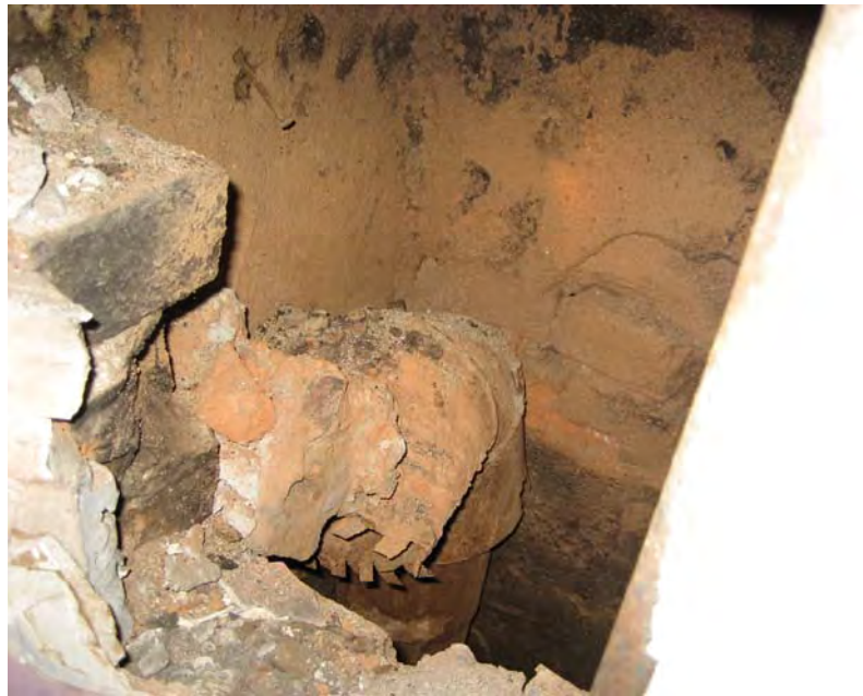
Figure 4-078: Elbow of metal tube in flue at third floor. (Photo: GHT, 2007)
