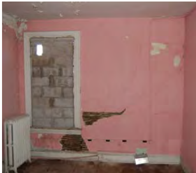
Figure 3-500: Plaster loss at west wall. (Photo: BBB, 2007)
