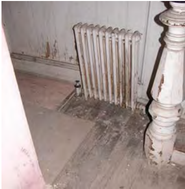
Figure 3-164: View looking west with cast iron radiator in front of painted bead board at stair. (Photo: BBB, 2006)
