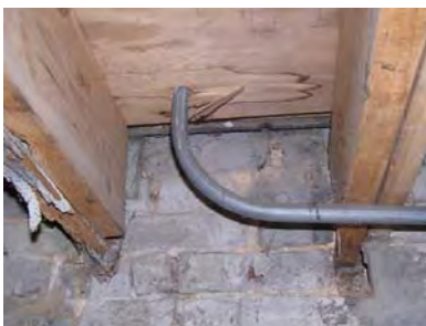
Figure 4-037: Insufficient Joist Bearing at north wall. (RSA, 2006)
