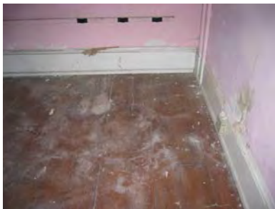
Figure 3-259: Five-inch wood plank flooring. (Photo: BBB, 2007)
