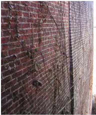
Figure 4-024: Bulging of north elevation. (RSA, 2006)
