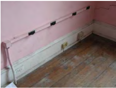
Figure 3-182: Surface mounted electrical outlets (Photo: BBB, 2006)
