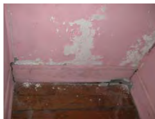
Figure 3-410: Water damage at south wall. (Photo: BBB, 2007)
