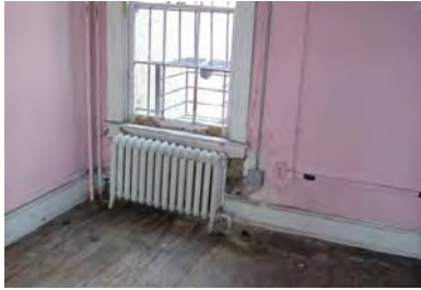
Figure 4-056: Photo 44. Room 205 - Cracking at window along west wall, original construction. (RSA, 2006)
