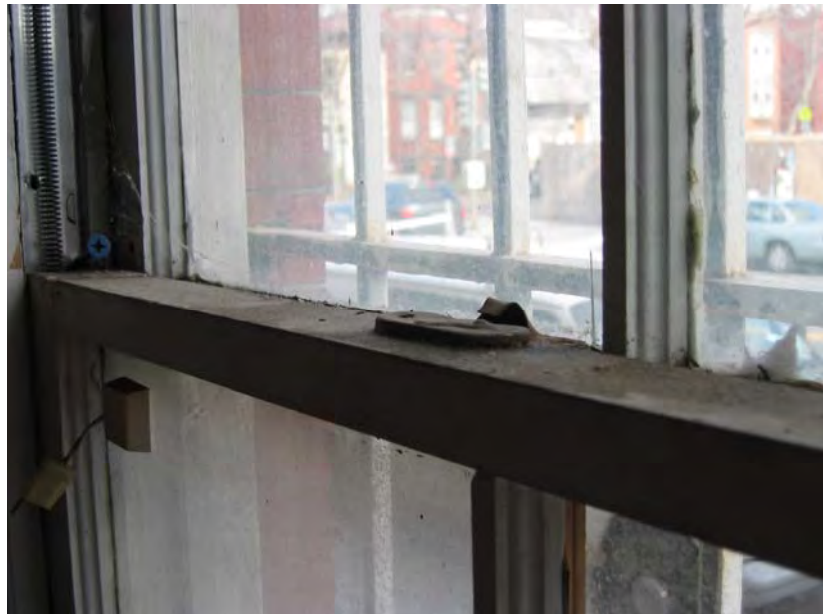
Figure 3-180: W101 sash, showing muntin, hardware and aluminum spring operated track. (Photo: BBB, 2006)
