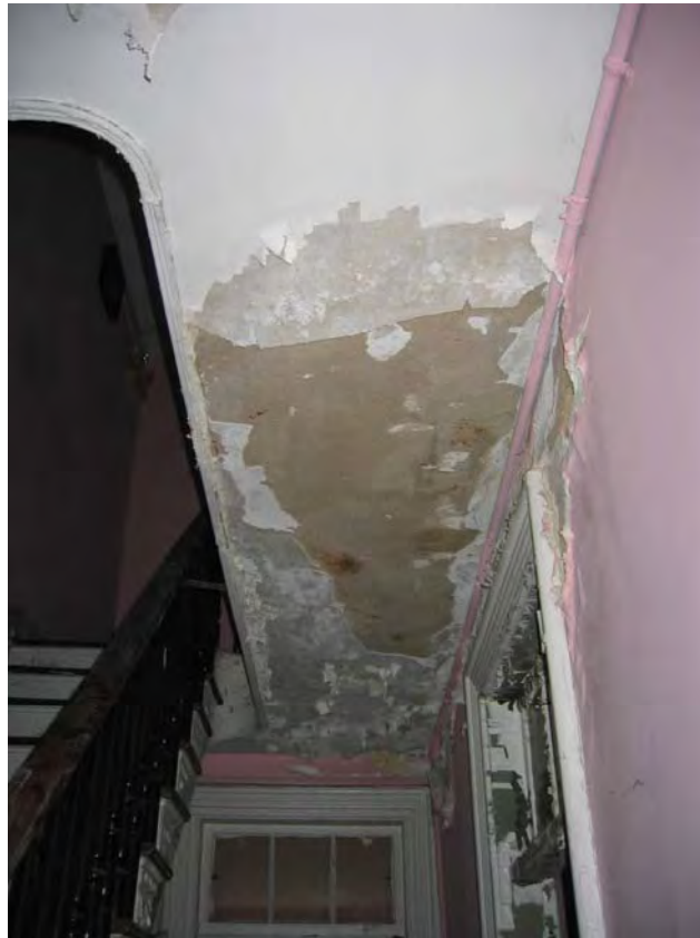
Figure 3-301: Plaster ceiling damage. (Photo: BBB, 2007)
