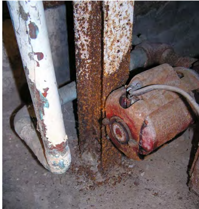
Figure 4-040. Rust and delamination at base of steel column. (RSA, 2006)
