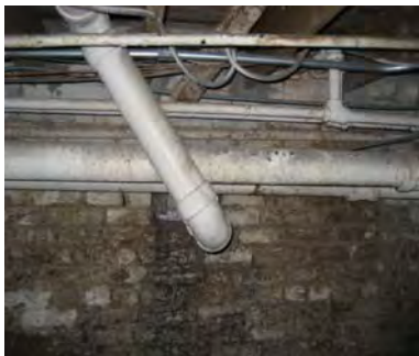
Figure 4-090: PVC sanitary waste pipe. (Photo: GHT, 2006)
