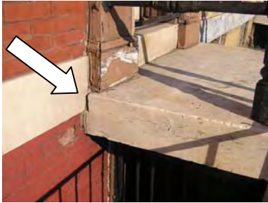
Figure 4-018: Spalling at front door. (RSA, 2006)
