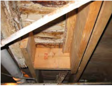
Figure 3-126: Sistering of joists. (Photo: BBB, 2007)
