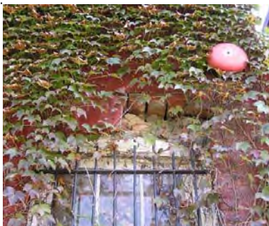
Figure 4-022: Loose and missing bricks at top of window W107. (RSA, 2006)
