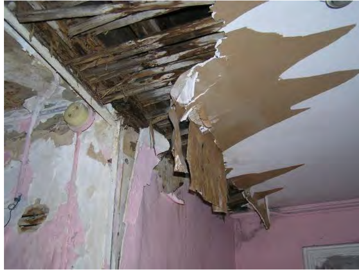
Figure 4-057: Room 201 - Fallen plaster ceiling and framing damage. (RSA, 2006)
