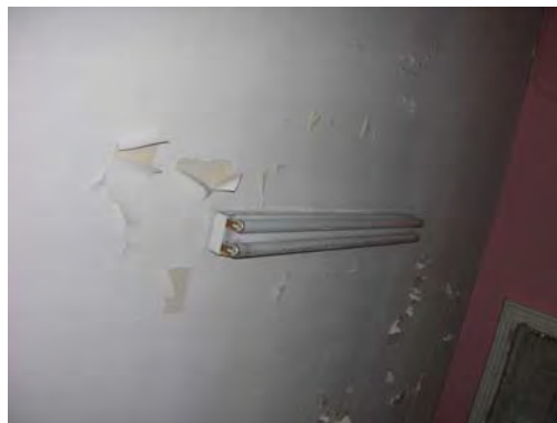
Figure 3-506: Ceiling showing light fixture and paint loss. (Photo: BBB, 2007)
