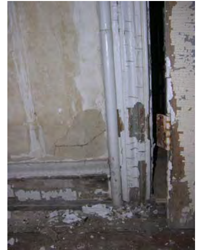
Figure 3-498: Water damage at wood base on north wall. (Photo: BBB, 2007)
