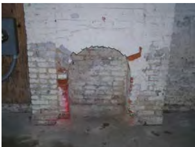
Figure 4-042: Fireplace, deterioration – southeast end. (RSA, 2006)
