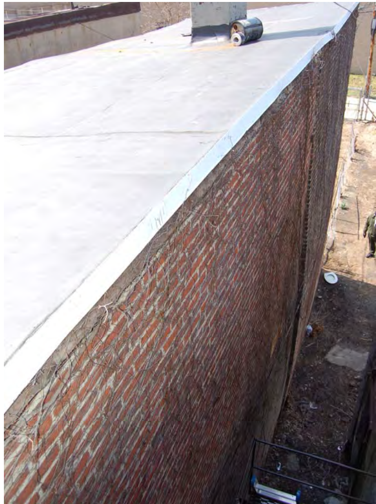
Figure 3-088: PVC flashing and wood fascia at lower roof. (Photo: BBB, 2007)
