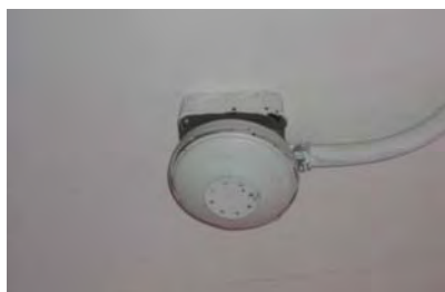
Figure 3-212: Smoke detector and conduit. (Photo: BBB, 2007)
