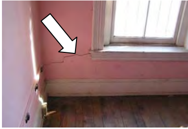
Figure 4-051: Room 104 - Crack at bottom lintel of window. (RSA, 2006)
