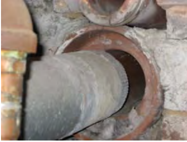
Figure 4-076: Boiler exhaust connection to flue. (Photo: GHT, 2007)
