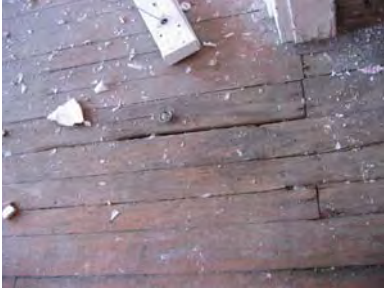
Figure 3-306: Floor damage at Door D203. (Photo: BBB, 2006)
