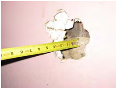
Figure 2-044: Gypsum wall board furred out at room 109 south wall. (Photo: BBB, 2006)
