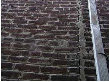
Figure 4-028: Separation of mortar at joint, between Period I and Period II construction. (RSA, 2006)
