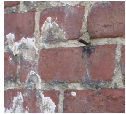
Figure 3-072: One of three ferrous metal anchors. (Photo: BBB, 2007)
