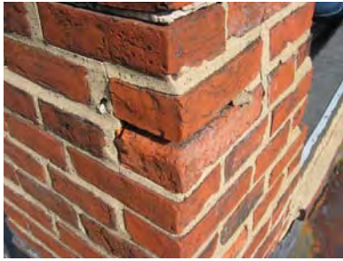
Figure 3-084: Open joints at chimney 1. (Photo: BBB, 2007)
