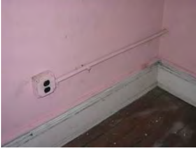
Figure 3-297: Typical base with surface mounted conduit above. (Photo: BBB, 2007)
