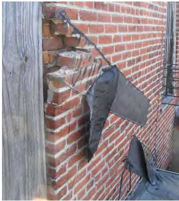
Figure 4-029: Cracking and bulging of west wall. (RSA, 2006)
