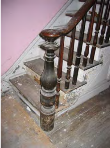
Figure 3-524: Newel post at second floor. (Photo: BBB, 2006)
