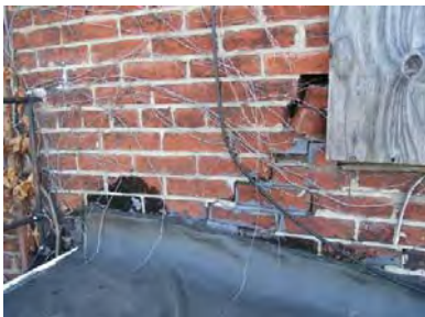
Figure 4-032: Photo 18. Diagonal cracking below window W303 at west wall. (RSA, 2006)
