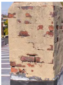
Figure 4-033: Masonry deterioration at chimneys. (RSA, 2006)
