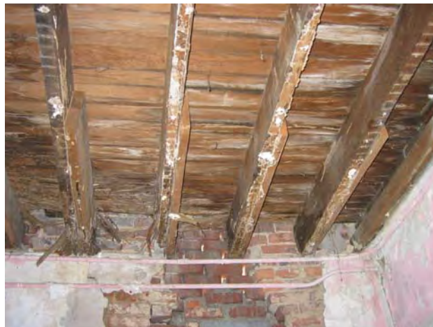
Figure 3-261: Exposed joists with shadowing of lath. (Photo: BBB, 2007)
