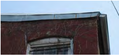
Figure 3-045: Aluminum flashing. (Photo: BBB, 2007)
