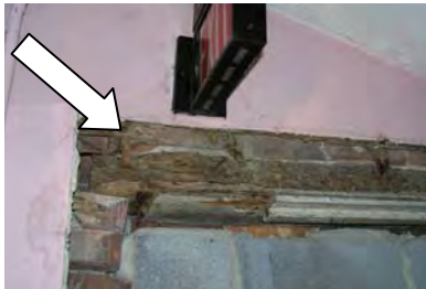
Figure 4-048: Deterioration at lintel of door D103A. (RSA, 2006)
