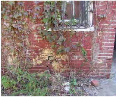
Figure 4-023: Loose bricks and rotting wood sill at window W107. (RSA, 2006)
