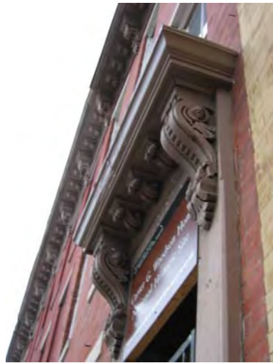
Figure 3-005: Bracketed and modillioned cornice. (Photo: BBB, 2006)
