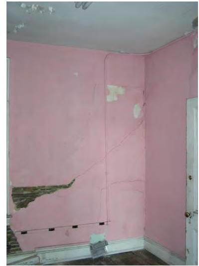
Figure 4-061: Room 305 - Diagonal cracks, west wall. (RSA, 2006)
