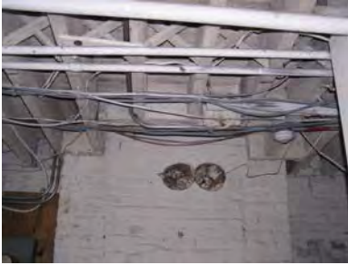
Figure 4-043: South chimney with insufficient trimmer support. (RSA, 2006)
