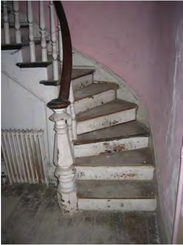
Figure 3-515: First floor newel post. (Photo: BBB, 2006)
