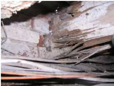
Figure 4-039: Rotted bearing end of stair framing. (RSA, 2006)
