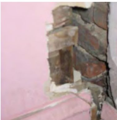
Figure 3-409: Opening at east wall corner along south wall exposing timber stud. (Photo: BBB, 2007)
