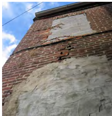
Figure 3-054: CMU infill and cementitious coating at W209 and D110A – note dislocated brick. (Photo: BBB, 2007)
