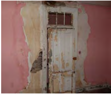
Figure 3-496: Plaster damage at north wall by door D305. (Photo: BBB, 2007)
