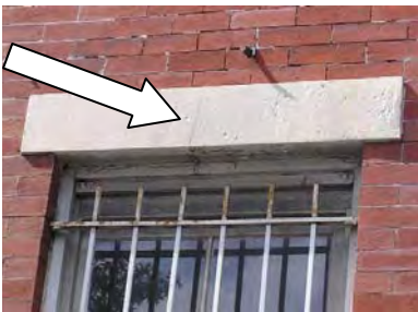
Figure 4-016: Crack in lintel at window W101. (RSA, 2006)
