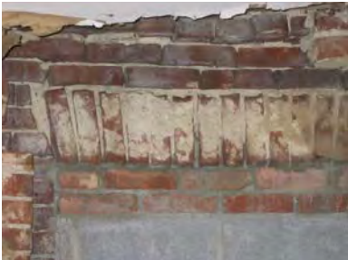
Figure 3-421: Failing flat arch at window W209. (Photo: BBB, 2007)
