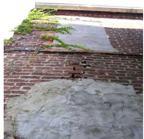
Figure 4-026: Cracking below second floor window W209. (RSA, 2006)
