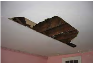
Figure 3-308: Loss of plaster wall board ceiling. (Photo: BBB, 2006)
