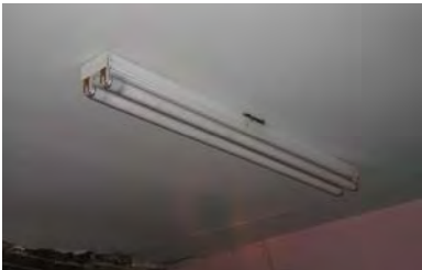
Figure 3-422: GWB ceiling with florescent light fixture. (Photo: BBB, 2007)
