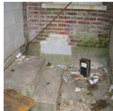
Figure 3-041: Concrete steps and CMU infill below W103. (Photo: BBB, 2007)
