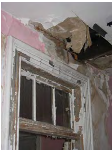
Figure 3-440: Transom damage at door D305. (Photo: BBB, 2007)
