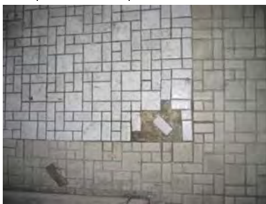
Figure 3-363: Patch at tile flooring. (Photo: BBB, 2007)
