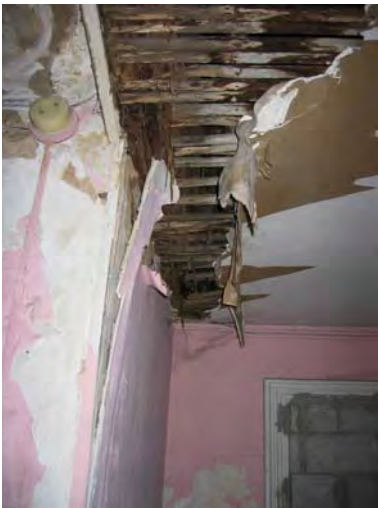
Figure 3-289: GWB and wood lath separating from structure. (Photo: BBB, 2007)
