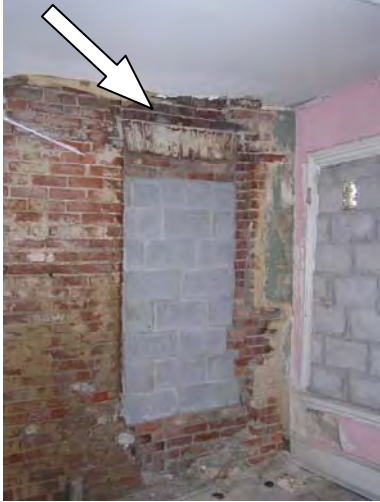
Figure 4-052: Room 210 - Brick failure at window. (RSA, 2006)
