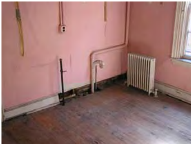
Figure 4-054: Room 208 - Floor sagging below east wall. (RSA, 2006)
