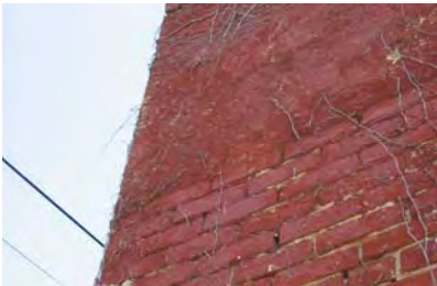
Figure 3-038: Cementitious coating and painted brick. (Photo: BBB, 2007)
