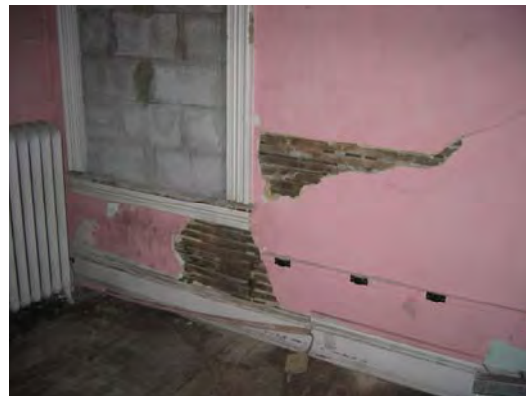
Figure 3-502: Loss of plaster and major cracks at west wall by window W304. (Photo: BBB, 2007)
