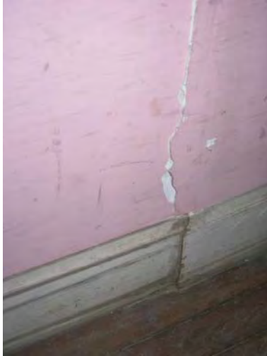
Figure 2-043: Joint showing line of infill for opening to room 105. (Photo: BBB, 2006)
