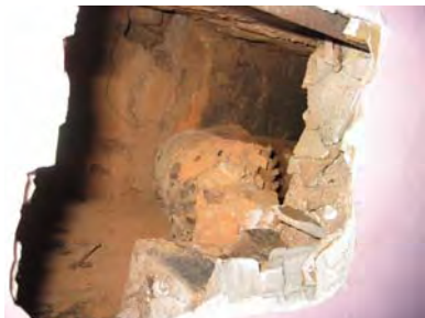
Figure 3-470: Probe at south wall chimney chase. (Photo: BBB, 2007)
