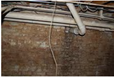
Figure 3-121: PVC pipe penetration with radiator pipes and conduit. (Photo: BBB, 2007)
