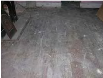
Figure 3-190: Flooring patch in front of fireplace with metal patch. (Photo: BBB, 2006)
