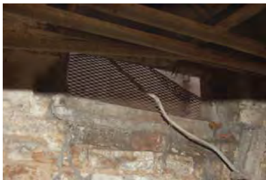
Figure 3-123: Opening W003 with wood frame and rusting wire grille. (Photo: BBB, 2007)
