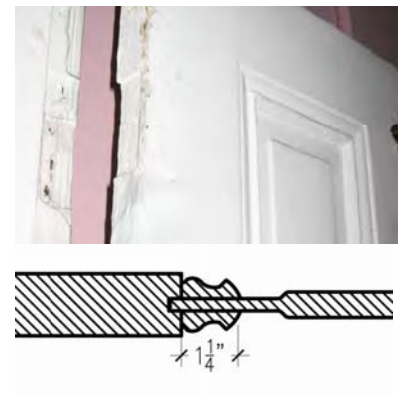
Figure 3-393: Door D210 molding type-7 photo and profile. (Photo: BBB, 2007)
