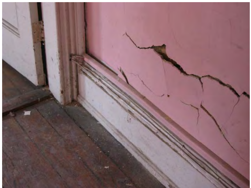
Figure 3-278: Plaster separating from substrate at north wall. (Photo: BBB, 2007)
