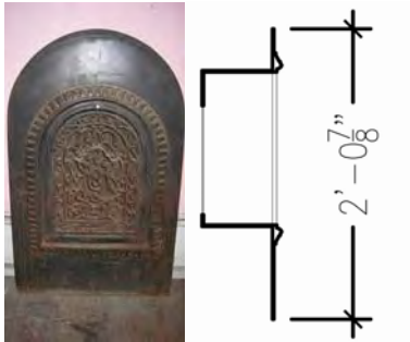
Figure 3-197: Fireplace grille photo and profile. (Photo: BBB, 2006)
