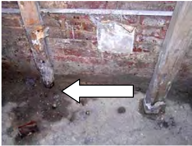
Figure 4-038: Base of column severely deteriorated. (RSA, 2006)
