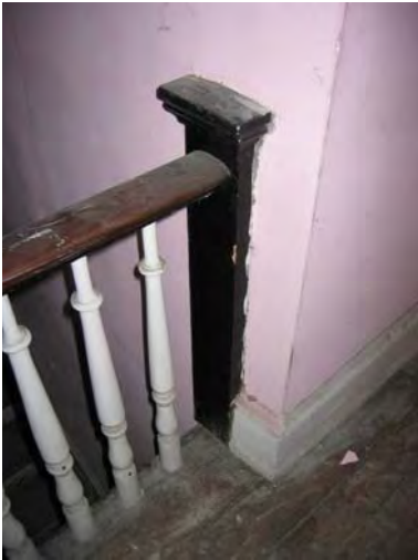
Figure 3-522: Pilaster at railing return at second floor. (Photo: BBB, 2006)
