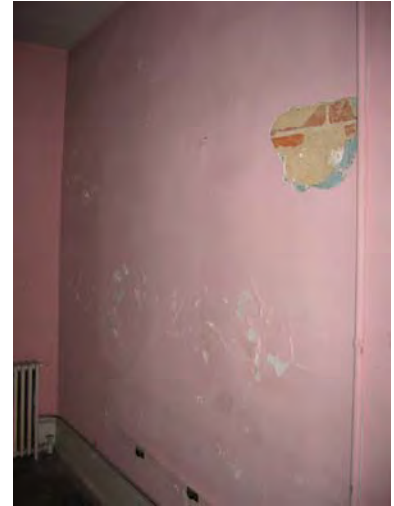
Figure 3-418: North elevation showing water damage to plaster. (Photo: BBB, 2007)
