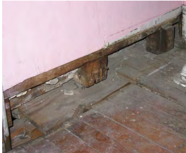
Figure 3-383: Missing base board at east wall exposing timber studs and cut nails.
