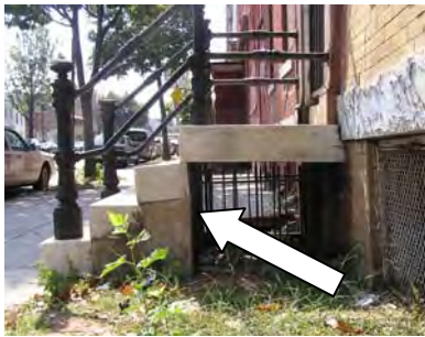
Figure 4-019: Stone rotation at front stoop, facing south. (RSA, 2006)
