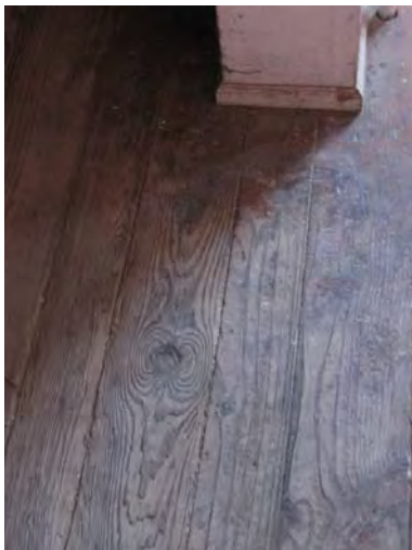
Figure 3-089: Pine tongue and groove flooring at Room 104. (Photo: BBB, 2006)
