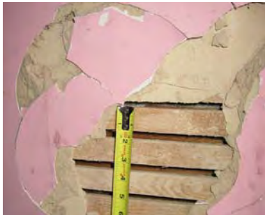
Figure 3-468: Loss of plaster at north wall exposing wood lath. (Photo: BBB, 2007)
