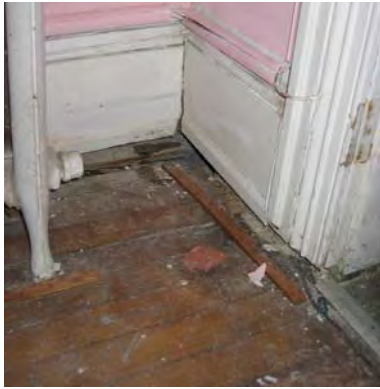
Figure 3-243: Sagging of floor in south west corner. (Photo: BBB, 2007)
