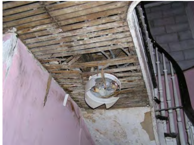
Figure 4-049: Room 103 - Fallen plaster at stairwell. (RSA, 2006)
