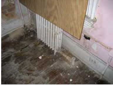
Figure 4-072: View of typical radiator and surface mounted conduit. (Photo: GHT, 2006)
