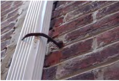
Figure 3-063: Flat cut nail and hook anchor for rain leader. (Photo: BBB, 2007)
