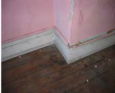
Figure 3-467: Wood base at south wall with surface mounted conduit. (Photo: BBB, 2007)
