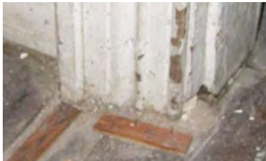
Figure 3-243: Sagging of floor in south west corner. (Photo: BBB, 2007)
