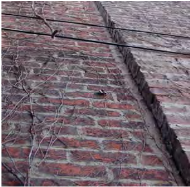
Figure 3-070: Joint on brick between 1872-74 and 1880 construction. (Photo: BBB, 2007)
