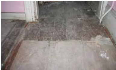
Figure 3-239: Tongue and groove and plywood flooring at door D109. (Photo: BBB, 2007)
