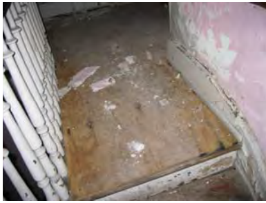
Figure 3-276: Plywood patch at top of stairs. (Photo: BBB, 2007)
