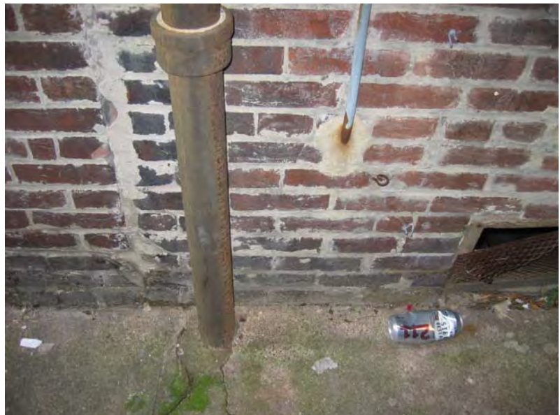
Figure 3-062: Three-inch cast iron storm drain, surface mounted conduit and miscellaneous ferrous anchors. (Photo: BBB, 2007)
