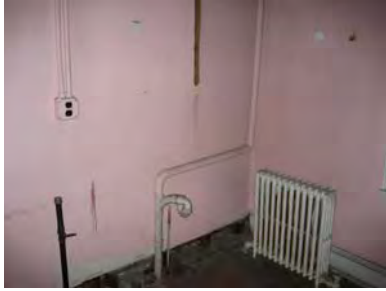
Figure 4-087: Radiator, radiator piping, sink and gas piping (Photo: GHT, 2006)
