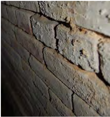
Figure 3-104: Open joists at north wall. (Photo: BBB, 2007)
