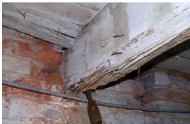
Figure 4-036: Rotted bearing condition. (RSA, 2006)
