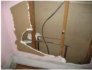
Figure 4-088: Remaining piping that has been cut. (Photo: GHT, 2006)
