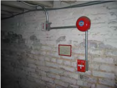
Figure 3-107: Fire alarm equipment on north wall. (Photo: BBB, 2007)
