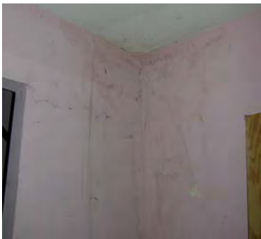
Figure 3-193: Water damage at northwest corner. (Photo: BBB, 2006)
