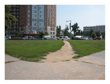
Res. 72- Section of fence on east edge of reservation (left of photo) to be removed and replaced along new pathway alignment. Center pathway to be straightened and nose of both grass panels to be reduced and edged with new quarter-round curb and end posts (see historic quarter-round curb detail). Brick DC sidewalks to remain. Reservation pathways to be replaced with new concrete/asphalt walkways.
