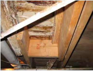
Figure 3-126: Sistering of joists. (Photo: BBB, 2007)
