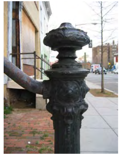
Figure 3-031: Cast iron railing detail. (Photo: BBB, 2007)
