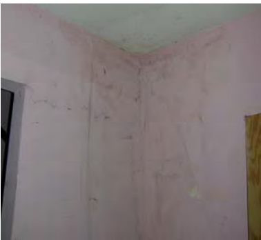
Figure 3-193: Water damage at northwest corner. (Photo: BBB, 2006)
