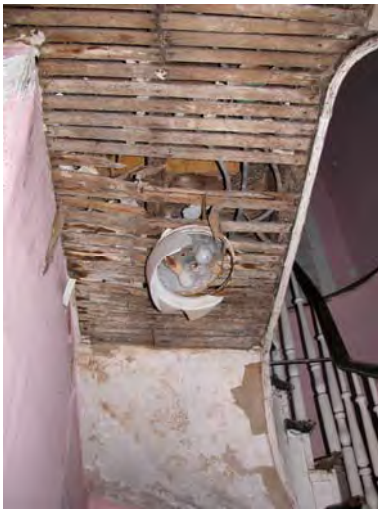
Figure 3-160: Room 103 ceiling damage and incandescent light fixture. (Photo: BBB, 2006)
