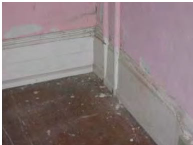
Figure 3-260: Wood base at radiator pipes. (Photo: BBB, 2007)
