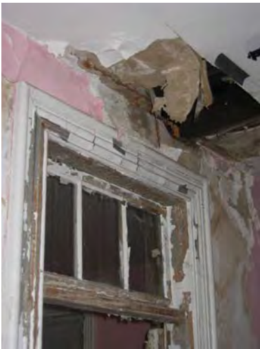
Figure 3-440: Transom damage at door D305. (Photo: BBB, 2007)
