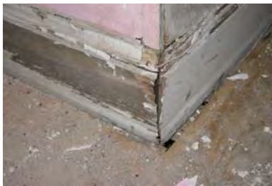
Figure 3-277: Deterioration of wood base. (Photo: BBB, 2007)
