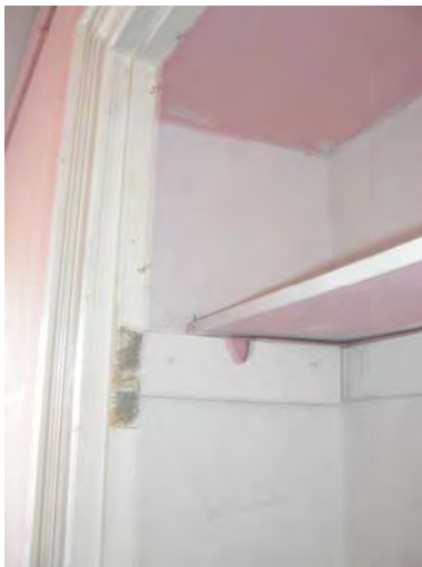
Figure 3-330: Shelf support with notch for clothing rod. (Photo: BBB, 2007)
