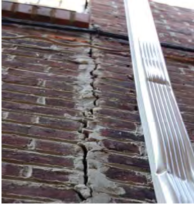
Figure 3-051: Joint between 1872-74 addition & 1880 addition. (Photo: BBB, 2007)
