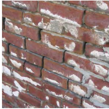
Figure 3-071: Cementitious coating and open joints. (Photo: BBB, 2007)
