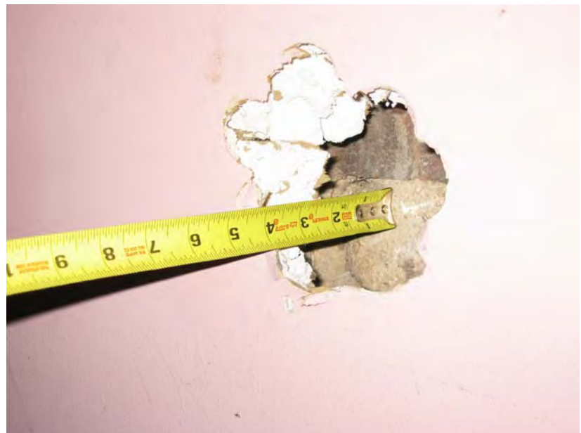
Figure 3-246: Furr-out at south wall. (Photo: BBB, 2007)
