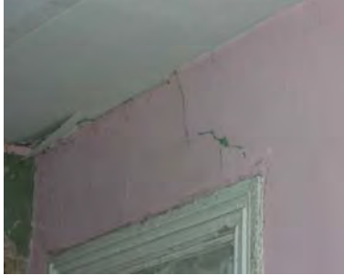
Figure 3-420: Plaster damage above W210. (Photo: BBB, 2007)
