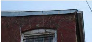
Figure 3-045: Aluminum flashing. (Photo: BBB, 2007)
