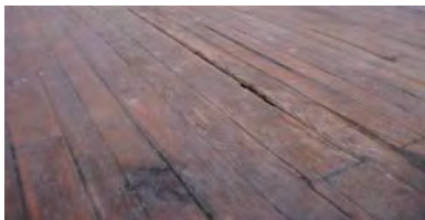
Figure 3-466: Separating at wood floor. (Photo: BBB, 2007)
