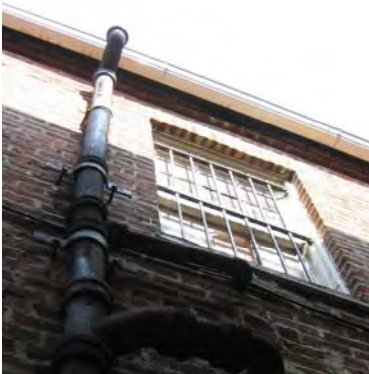
Figure 3-061: Four-inch cast iron sanitary pipe with bolted anchor brackets and nail and hook anchors. (Photo: BBB, 2007)
