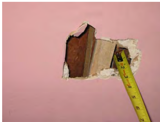
Figure 3-407: Probe at west wall showing GWB with wood lath beyond. (Photo: BBB, 2007)
