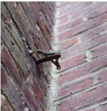
Figure 3-065: Miscellaneous metal anchor. (Photo: BBB, 2007)
