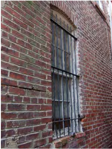
Figure 3-052: Window W106 with curved brick arch and replacement sill. (Photo: BBB, 2007)
