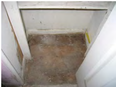
Figure 3-217: Plywood flooring with wood base. (Photo: BBB, 2007)
