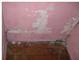
Figure 3-410: Water damage at south wall. (Photo: BBB, 2007)
