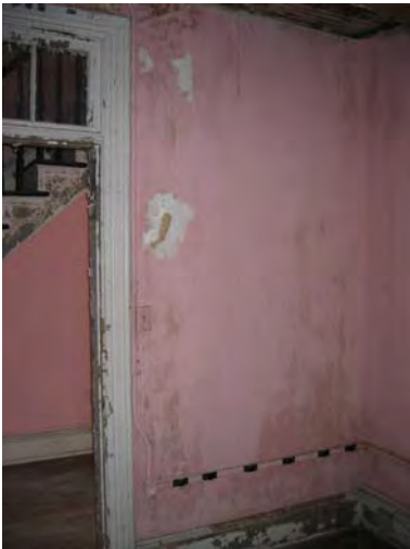
Figure 3-338: Water damage at north wall. (Photo: BBB, 2007)
