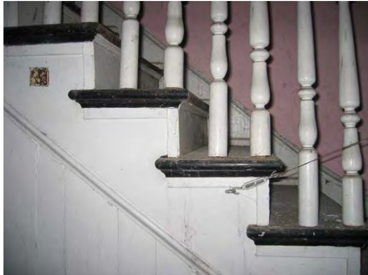
Figure 3-521: Stringer at first floor stair. (Photo: BBB, 2007)
