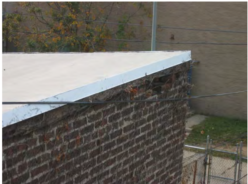
Figure 3-074: 3 ½" PVC flashing over 6" wood fascia. (Photo: BBB, 2007)
