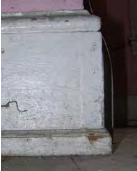
Figure 3-172: Base molding type-1, photo and profile. (Photo: BBB, 2006)
