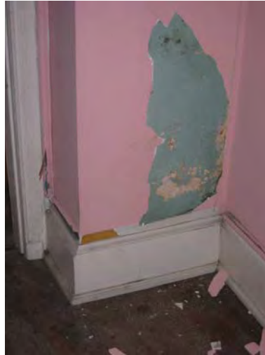
Figure 3-417: Wood base and plaster damage at chimney flue. (Photo: BBB, 2007)
