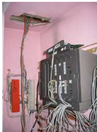
Figure 3-356: Telephone distribution box on south wall. (Photo: BBB, 2007)
