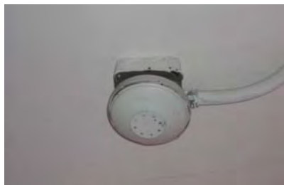
Figure 3-212: Smoke detector and conduit. (Photo: BBB, 2007)
