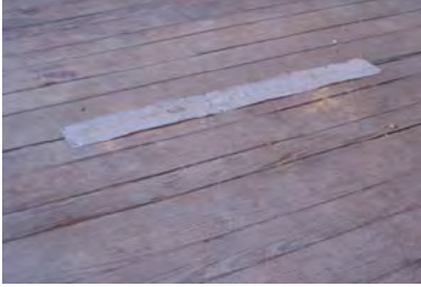
Figure 3-171: Room 104 pine wood flooring patch. (Photo: BBB, 2005)
