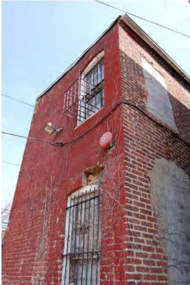
Figure 3-046: Surface mounted light fixture and fire alarm bell. (Photo: BBB, 2007)
