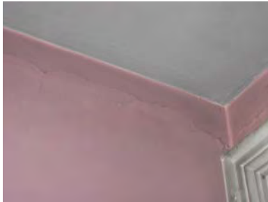
Figure 3-458: Hairline cracks on walls close to ceiling. (Photo: BBB, 2007)
