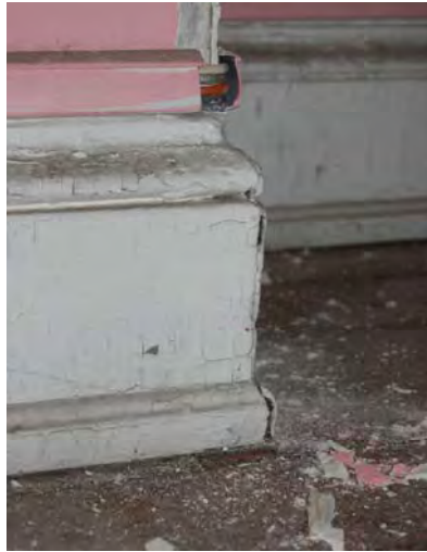
Figure 3-497: Base showing surface mounted telephone conduit. (Photo: BBB, 2007)
