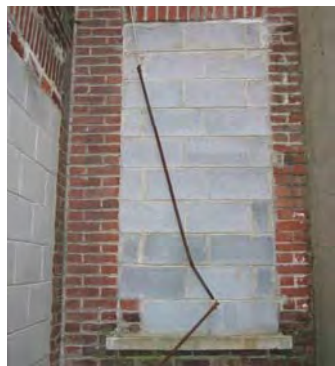
Figure 3-040: CMU infill and concrete sill at W103. (Photo: BBB, 2007)
