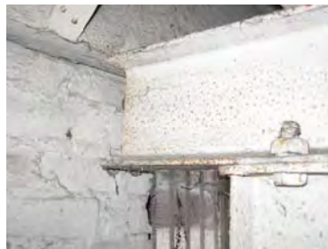
Figure 3-115: Phoenix steel beam. (Photo: BBB, 2007)
