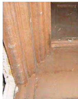
Figure 3-141: Door D101 transom type-1 photo and profile. (Photo: BBB, 2006)
