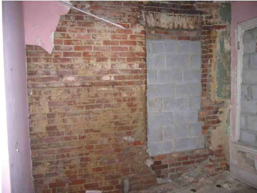
Figure 3-412: South elevation with window opening W209 showing complete loss of plaster. (Photo: BBB, 2007)
