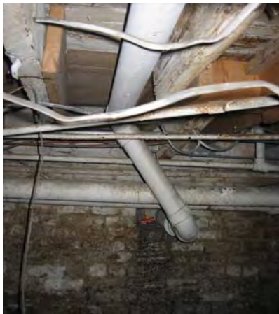
Figure 3-122: PVC piping at ceiling. (Photo: BBB, 2007)
