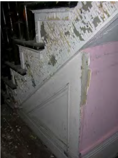
Figure 3-300: West wall with evidence of skim coat below stair. (Photo: BBB, 2007)
