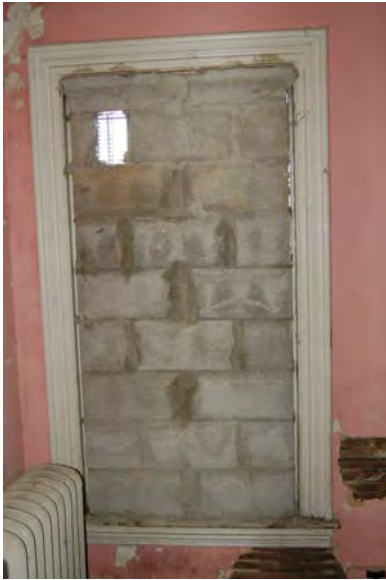
Figure 3-503: CMU infill at window W304. (Photo: BBB, 2007)
