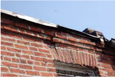
Figure 3-037: Corbelled cornice at third story elevation. (Photo: BBB, 2007)
