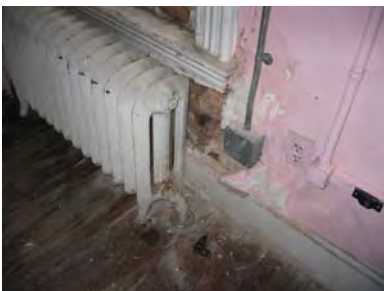
Figure 3-340: Plaster damage below window W204. (Photo: BBB, 2007)
