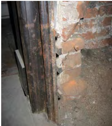
Figure 3-199: Fireplace attachment to masonry. (Photo: BBB, 2006)
