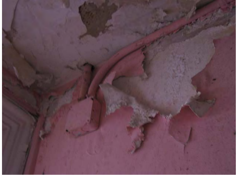
Figure 3-298: South wall – east corner water damage and surface mounted conduit. (Photo: BBB, 2007)
