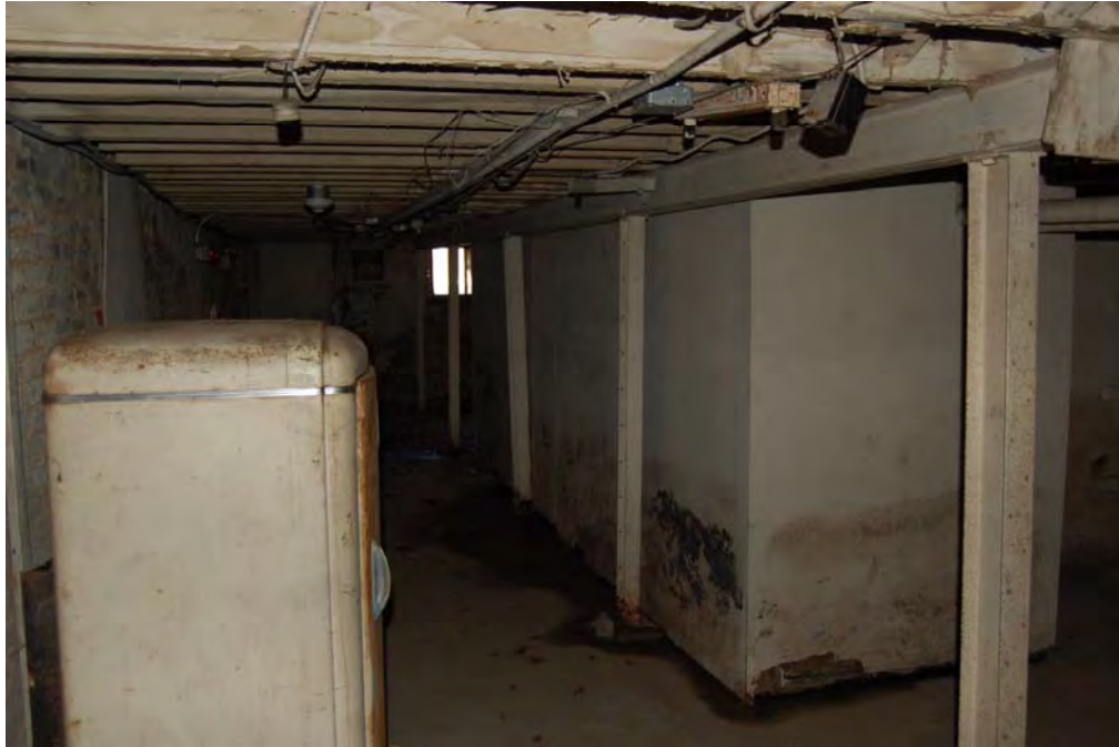
Figure 3-100: View looking east with Phoenix steel columns on right. (Photo: BBB, 2007)
