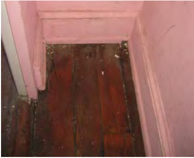
Figure 3-486: Flooring with evidence of a floor finish. (Photo: BBB, 2007)
