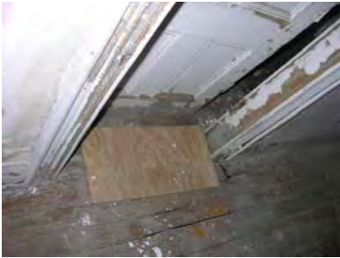
Figure 3-427: Plywood patch at floor of door D305. (Photo: BBB, 2007)
