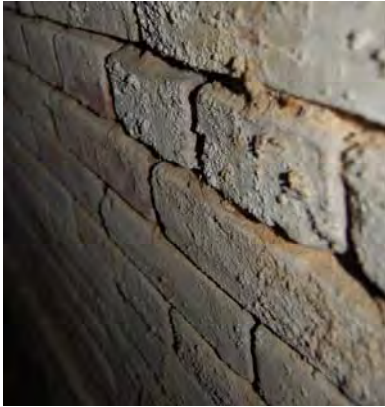
Figure 3-104: Open joists at north wall. (Photo: BBB, 2007)
