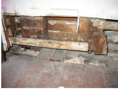
Figure 3-382: Exposed studs and lath at east wall. (Photo: BBB, 2007)
