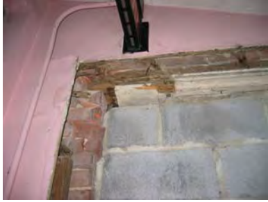
Figure 3-163: Door 103A head detail – not shadow of removed mullion. (Photo: BBB, 2006)
