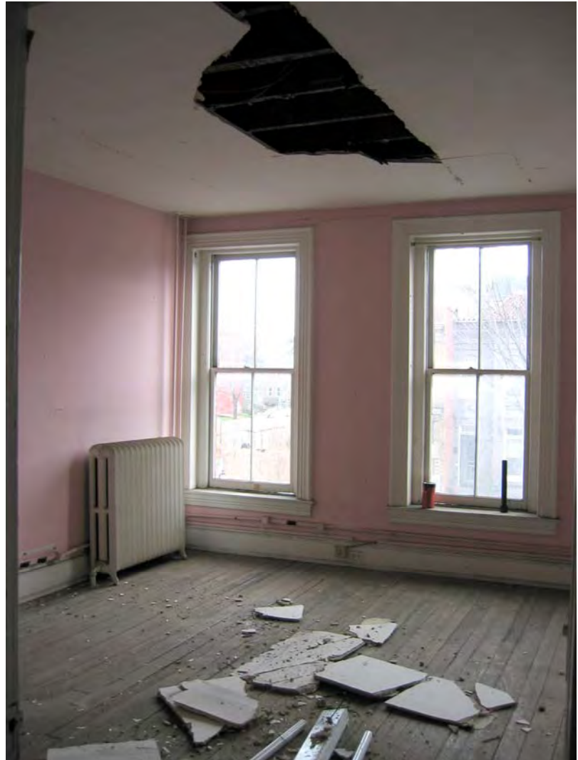
Figure 3-325: Room 203 ceiling failure. (Photo: BBB, 2006)
