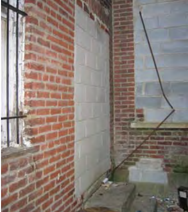
Figure 3-060: Door D103A with CMU infill. (Photo: BBB, 2007)
