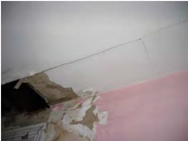
Figure 3-449: Cracks at rock lath ceiling panels. (Photo: BBB, 2007)
