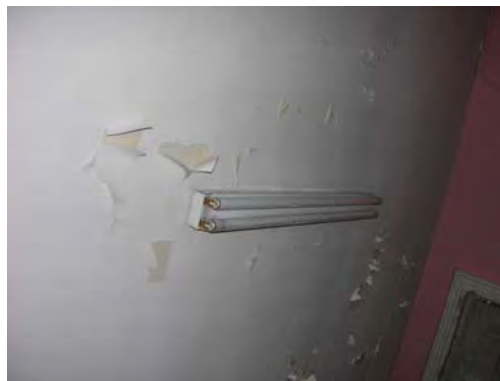
Figure 3-506: Ceiling showing light fixture and paint loss. (Photo: BBB, 2007)
