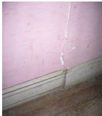
Figure 3-150: Line of infill patch at south wall. (Photo: BBB 2005)
