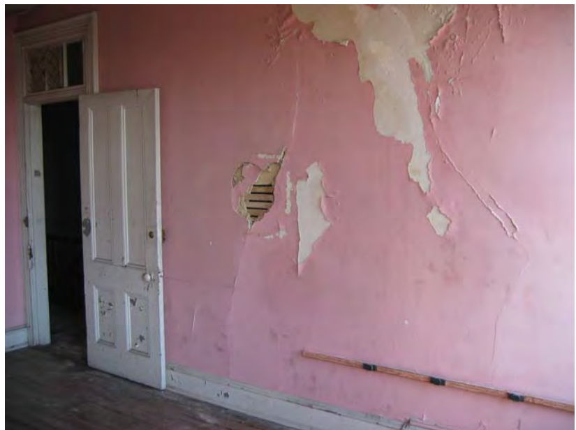
Figure 3-469: North wall showing water damage and loss of plaster. (Photo: BBB, 2007)
