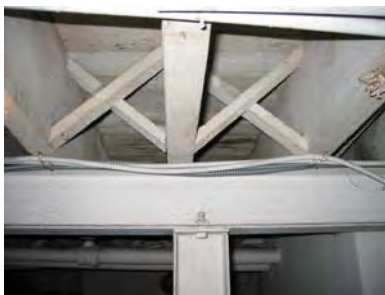
Figure 3-013: Phoenix steel beams at basement. (Photo: BBB, 2006)
