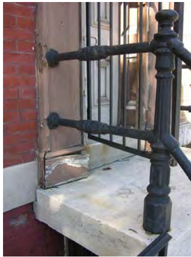
Figure 3-030: Cast iron guard railing detail. (Photo: BBB, 2007)
