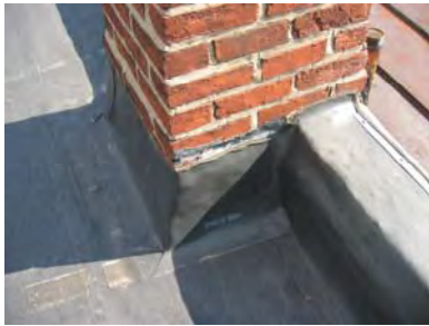
Figure 3-085: Roof flashing at party wall; chimney 1 joint. (Photo: BBB, 2007)
