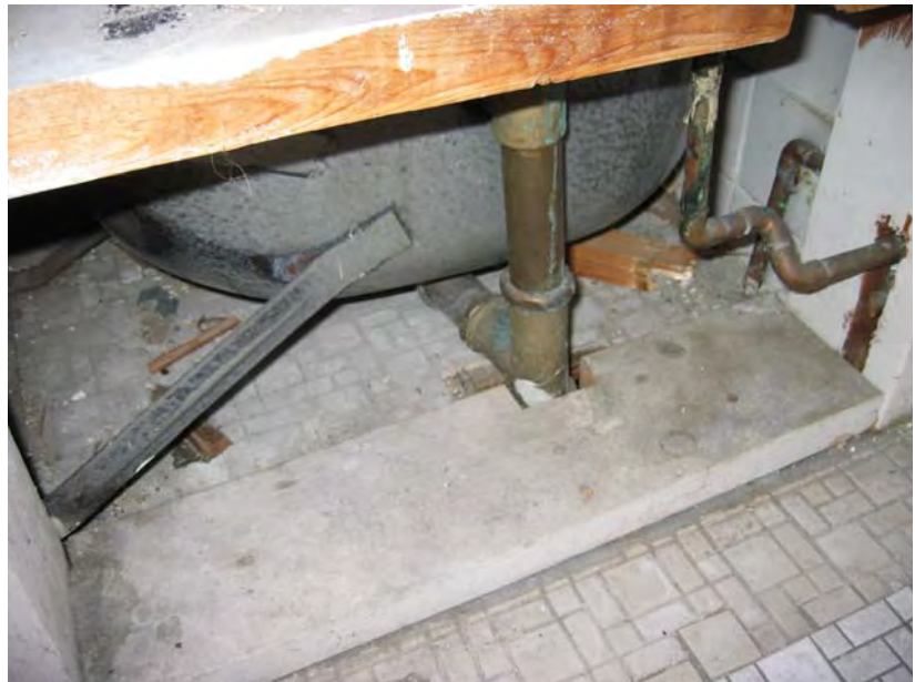
Figure 3-365: Tile extending below tub. (Photo: BBB, 2007)
