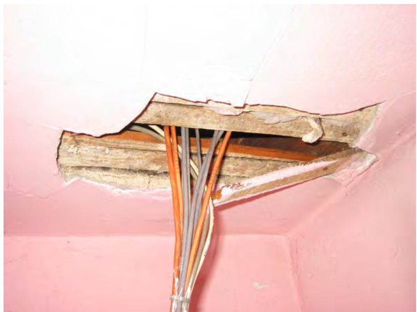
Figure 3-358: Hole in plaster at ceiling. (Photo: BBB, 2007)
