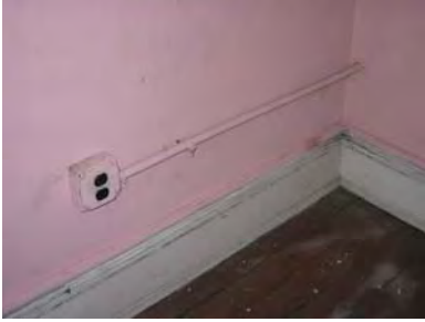
Figure 3-297: Typical base with surface mounted conduit above. (Photo: BBB, 2007)
