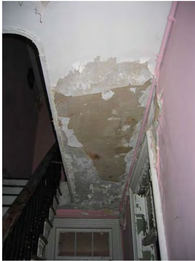
Figure 3-301: Plaster ceiling damage. (Photo: BBB, 2007)
