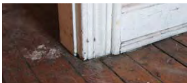
Figure 3-457: Base detail showing evidence of floor finish. (Photo: BBB, 2007)
