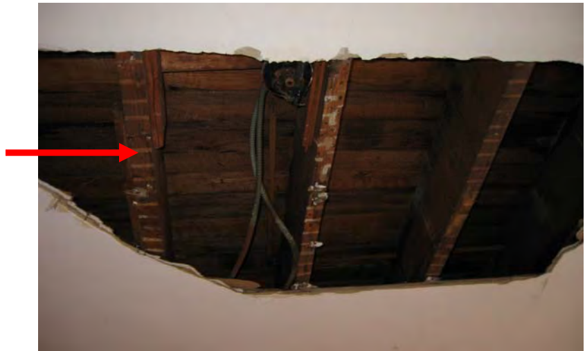
Figure 8-XXX: Ghosting from plaster keys on ceiling joists behind plaster board. (Photo: BBB, 2006)
