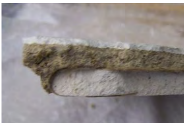
Figure 8-004: Cross-section of rock lath with keyed plaster brown coat and finish coats. (Photo: JB, 2007)
