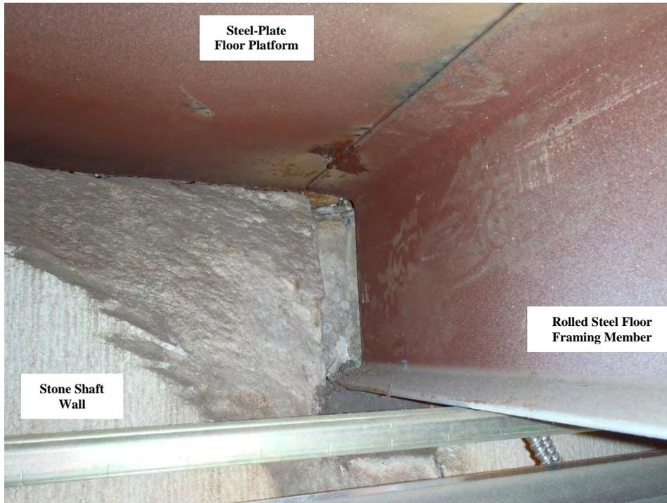
Figure 21. Photograph of bearing-type connection between floor framing and stone wall
