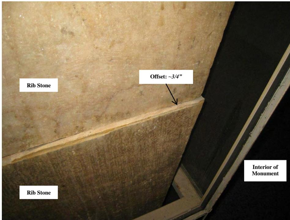
Figure 24. Horizontal offset between rib stones documented at the observation level
