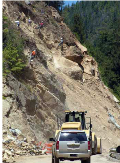
FIGURE 7. MANUAL ROCK SCALING
