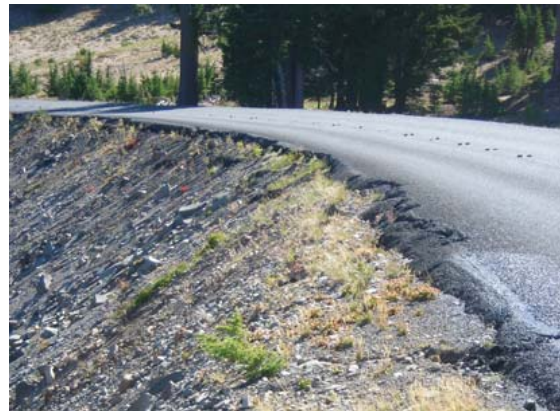
FIGURE 15. BENCH EROSION AND UNRAVELING PAVEMENT EDGE
