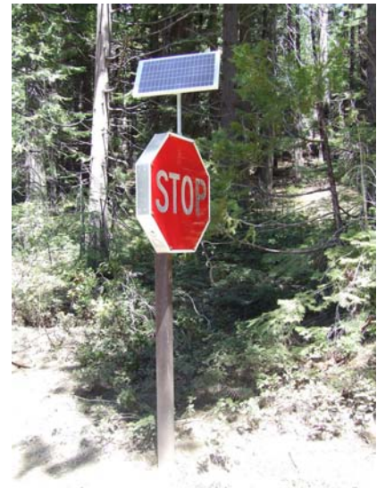
Figure 3-38 – Solar-powered Sign at South Entrance
