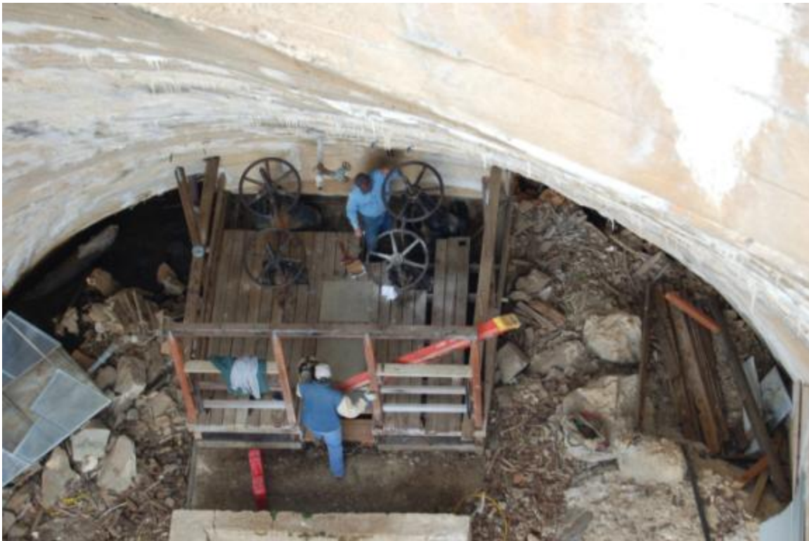
Picture 4. The lower valves at Lake Eleanor.
