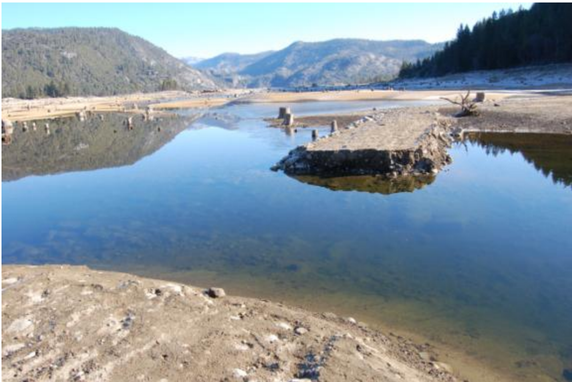
Picture 3. The breached section of the coffer dam
