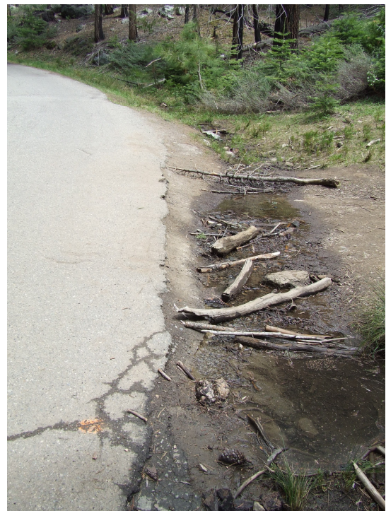
Figure 3-16 – Drainage Channel along the Mariposa Grove Road within the Grove
