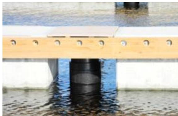
Figure 6: Example of Telescoping Piles
