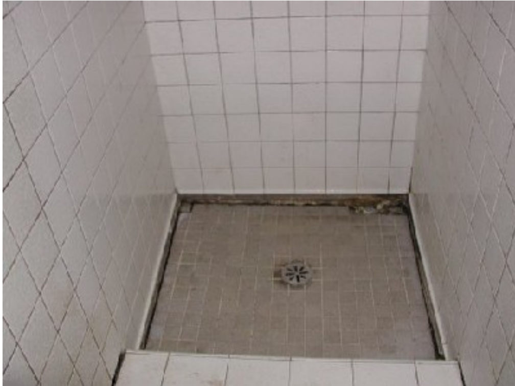
Photo 7 Shower Tile Damage-Sinking Floor
