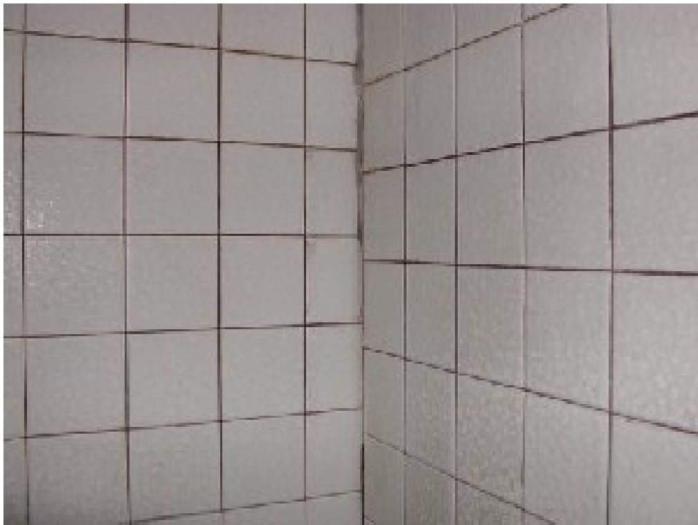
Photo 6 Shower Tile Offset Damage
