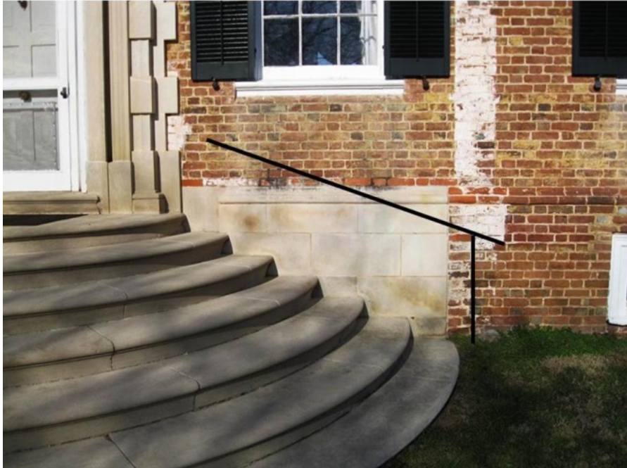
Close up of west entrance to Chatham Manor. Black lines to the left of the door represent proposed railing attached to the exterior wall.
