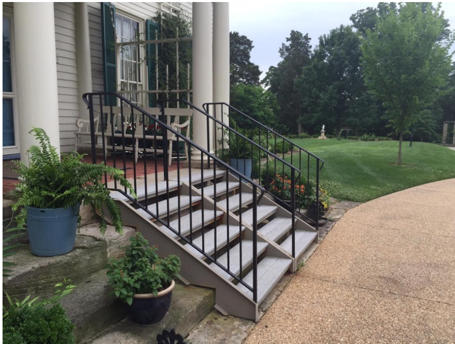
The removable slip-over steps in use at the Gari Melchers Home and Studio Belmont. This alternative would create additional safety concerns at Chatham Manor, plus it is not compatible with the elliptical steps at Chatham.
