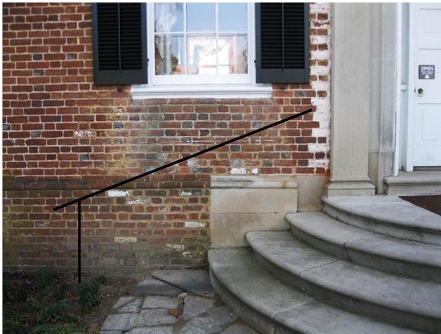
Close up of east entrance to Chatham Manor. Black lines to the left of the door represent proposed railing attached to the exterior wall.
