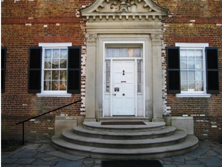
East entrance to Chatham Manor. Black lines to the left of the door represent proposed railing attached to the exterior wall.
