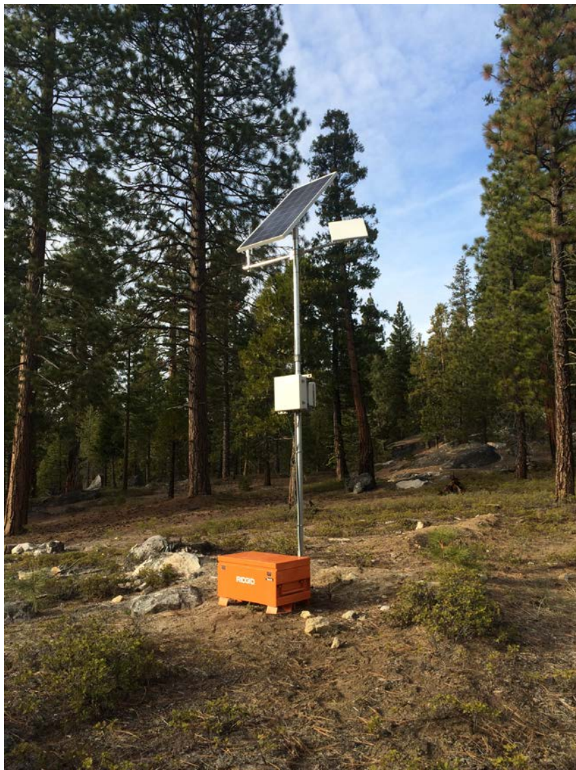
Figure 2. Telemetry pole installation. The proposed installation would use a solar panel that is approximately \frac{1}{2} the size illustrated here with the battery box mounted on the pole (not on the ground as pictured here).
