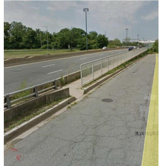
The existing bridge approach from the east shows the narrow sidewalk on the north side of the bridge. The break in the guardrail provides a narrow connection to the adjacent neighborhood.
