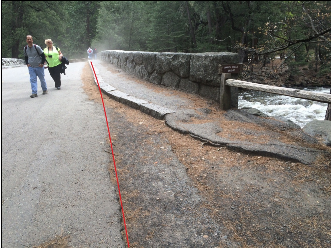
Figure 7. The shoulder of the road connects to Happy Isles Vehicle Bridge. This project includes making a continuous line from the stone curb on the bridge to the proposed formalized path.
