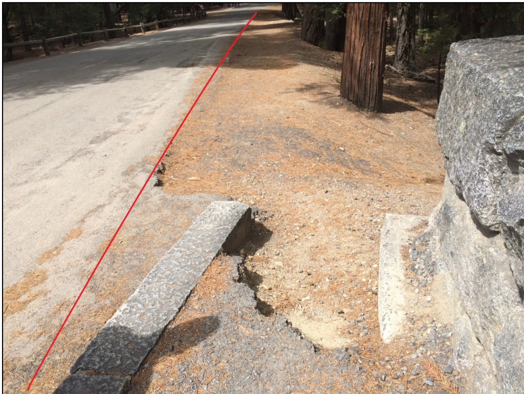
Figure 8. The shoulder-bridge connection on the other side of the road is severely eroded by stock use.
