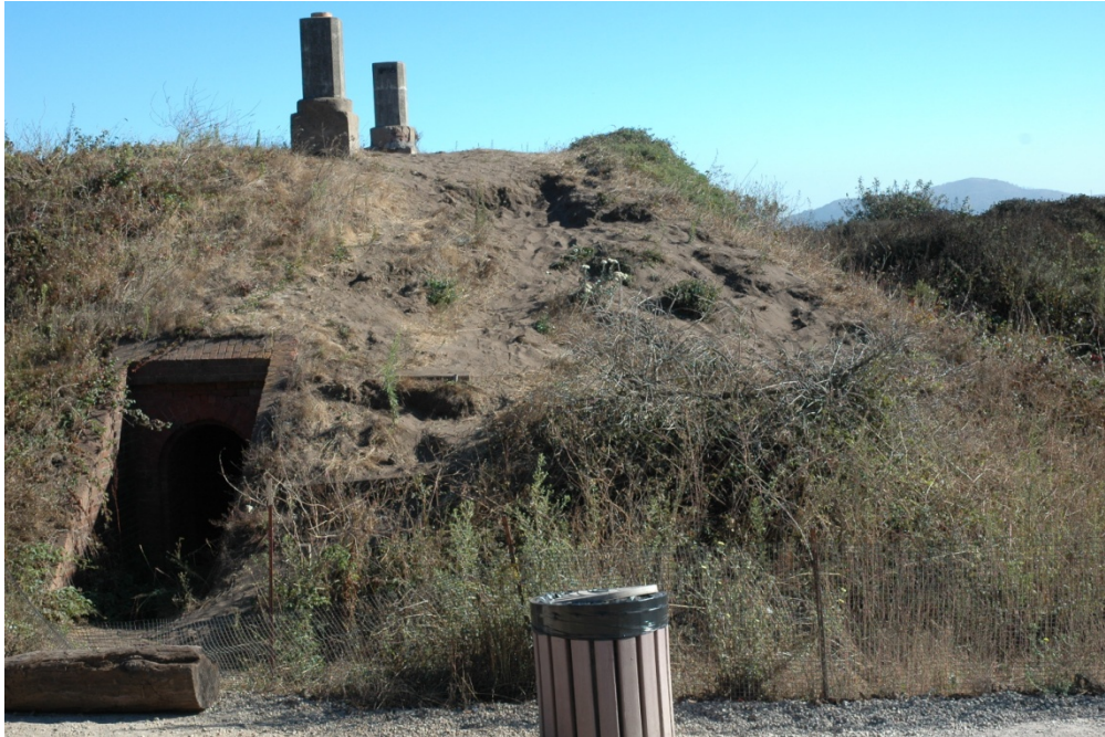
FIGURE 3. BATTERY EAST, WITH EROSION OF EARTHWORKS EVIDENT
