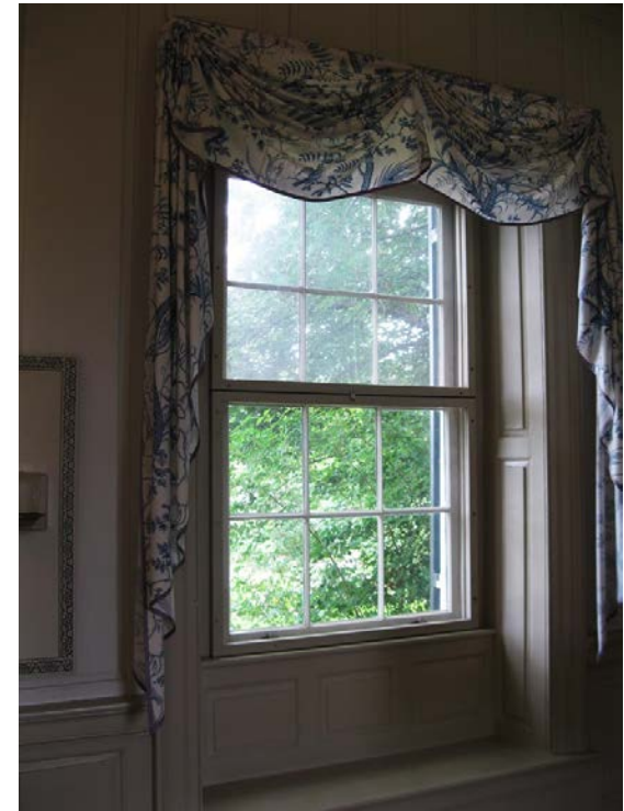
Typical double hung sash window in Chatham Manor FRSP proposes to install an interior storm window. In the exhibits rooms, the windows will be tinted to reduce penetration of UV light.
