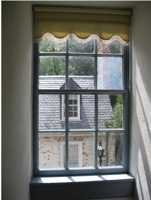
Typical double hung sash window in Chatham Kitchen. FRSP proposes to install an interior storm window.
