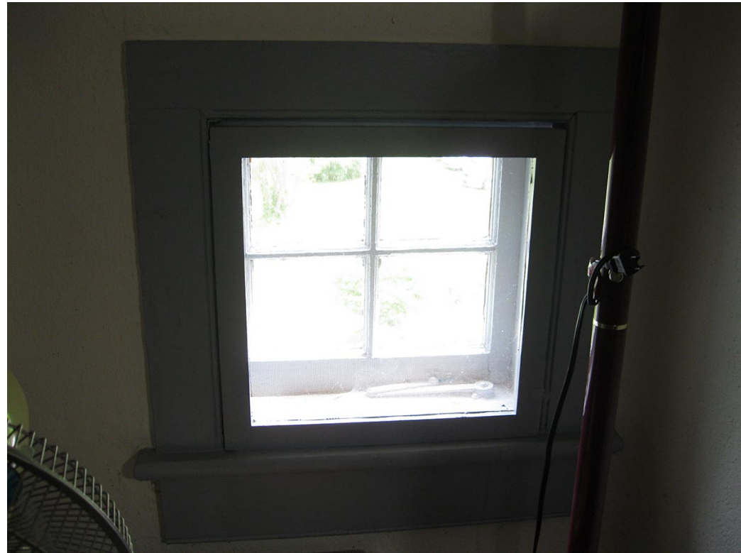
Typical casement window in Chatham Kitchen. FRSP proposes to install an interior storm window.
