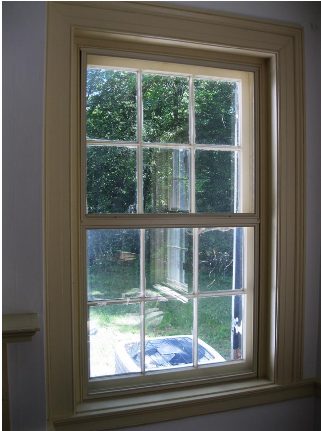
Interior storm window in the Superintendent's House (Quarters #2). The park proposes to use this same style of interior storm window. Two pane for the second floor of Chatham Manor, and single pane for the first floor, as well as the Laundry and Kitchen.
