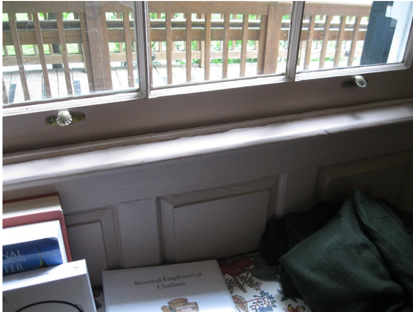
Detail of typical double hung sash window in Chatham Manor. The decorative brass handles will be removed, bagged, tagged, and stored.
