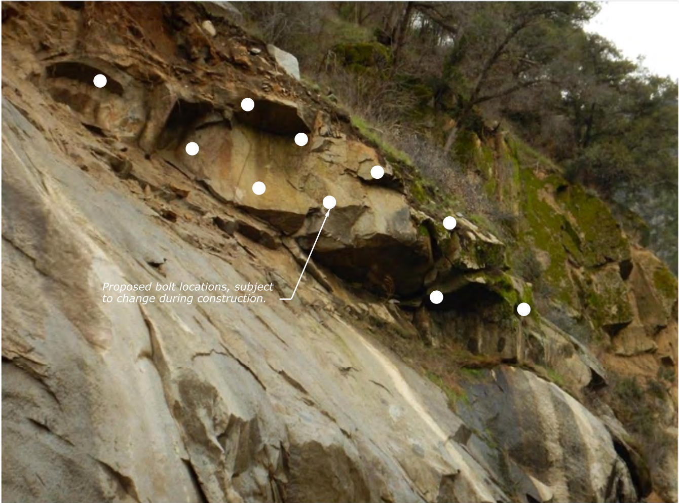
Photo 2: El Portal rock bolt location
