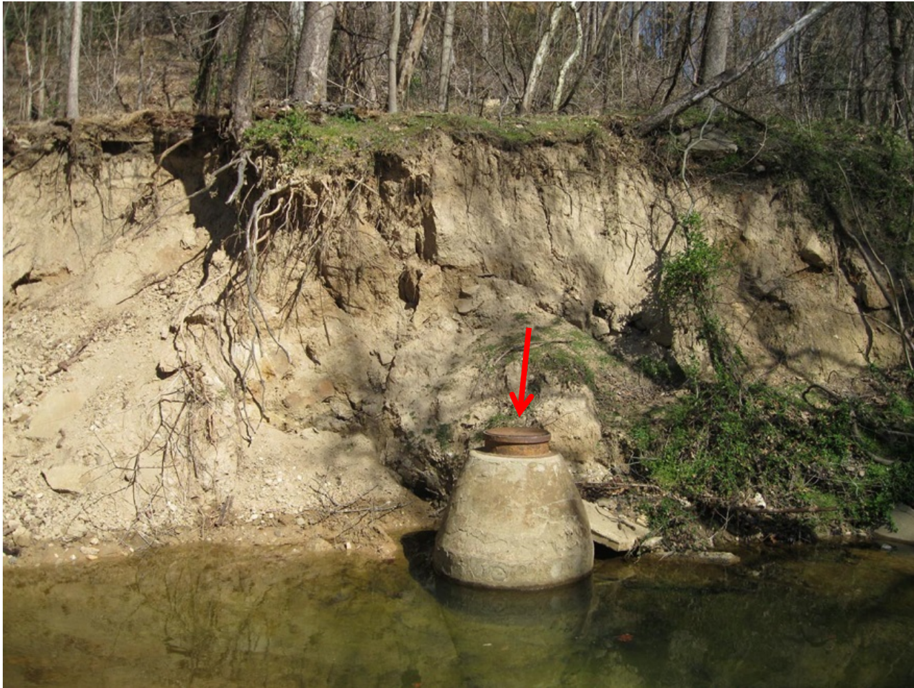
A view of the exposed manhole, indicated by the arrow. Gabions and clean backfill will protect the manhole.
