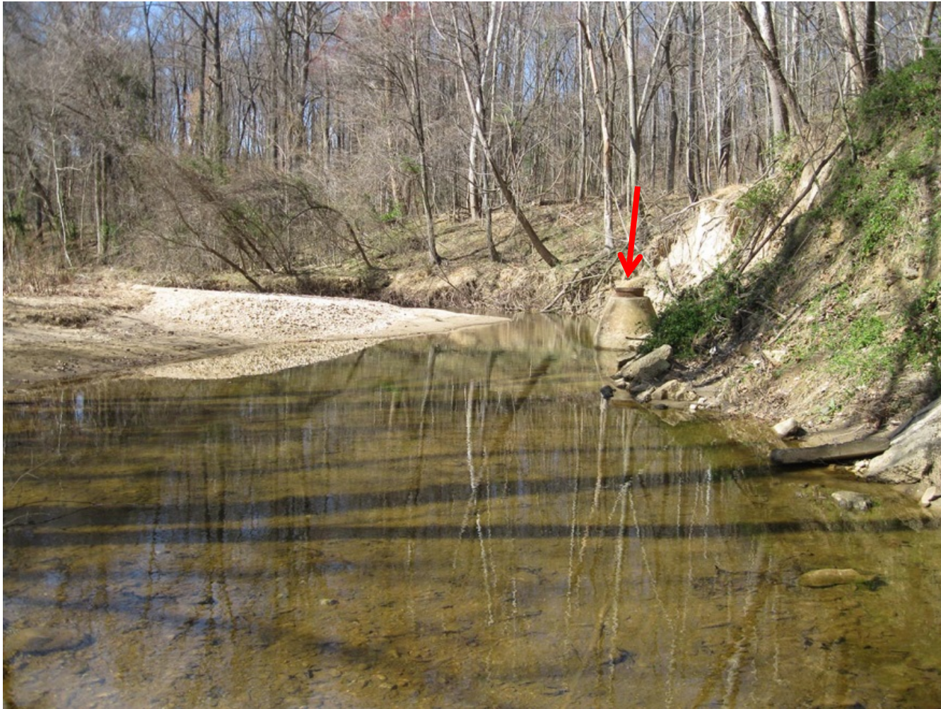
A view upstream along Hazel Run – note the dominant channel to the right, which is eroding the left bank in the distance. The exposed manhole is indicated by the arrow. Rock toe revetment will reinforce the left bank, while gabions and clean backfill will protect the manhole. Two log vanes will be installed in the stream to the left background.
