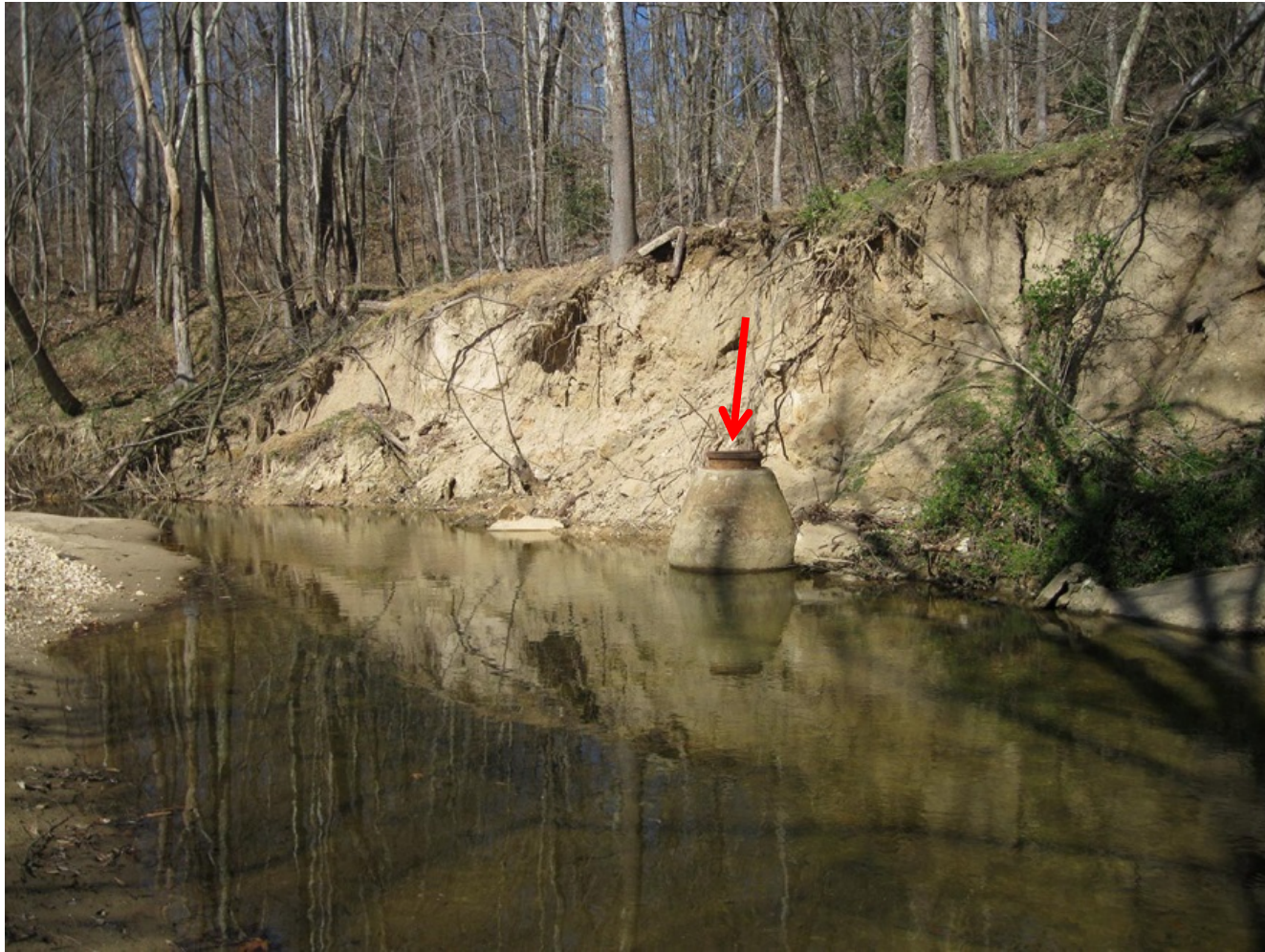
A view upstream along Hazel Run – note the dominant channel to the right, which is eroding the left bank. The exposed manhole is indicated by the arrow. Rock toe revetment will reinforce the left bank, while gabions and clean backfill will protect the manhole. Two log vanes will be installed in the stream out of sight to the left background.
