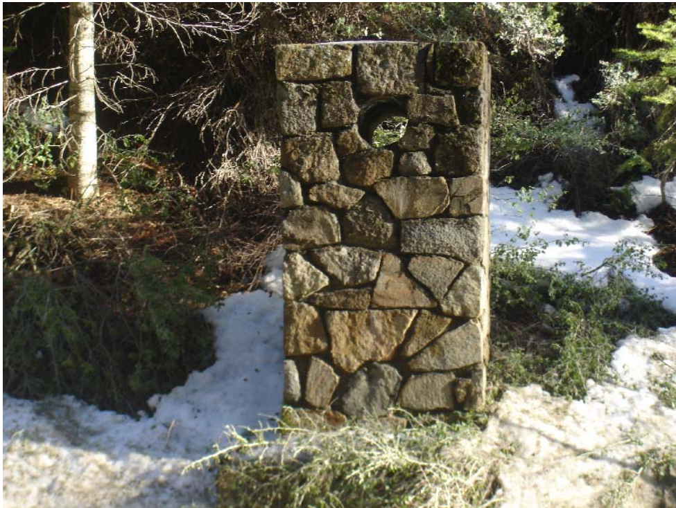
Photo 1 South Entrance Boundary Marker showing hole for the missing log that holds the entrance sign
