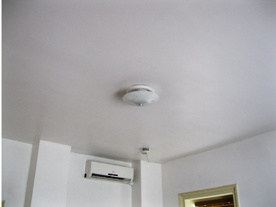
Gypsum ceiling in the first floor bedroom (Room #102). The gypsum ceiling will be removed and the piping run to sprinkler heads in the ceiling. A new gypsum ceiling will be installed.
