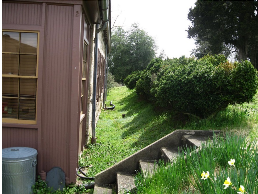
Looking south along the west face of the cemetery lodge. A 2" water line along the side of the building, about three feet from the structure. The waterline will be excavated, removed and replaced with a 4" line within the same trench. The boxwoods may be removed in order to access the waterline. They will be replaced with new boxwoods.
