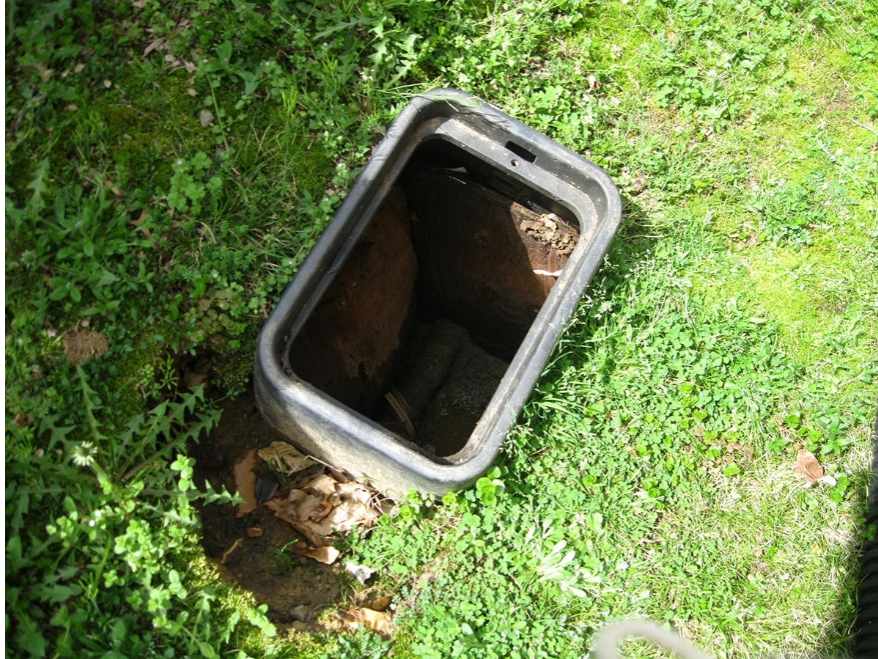
A hand hole from a previous repair of the 2" waterline on the west face of the cemetery lodge. The waterline will be excavated, removed and replaced with a 4" line within the same trench.
