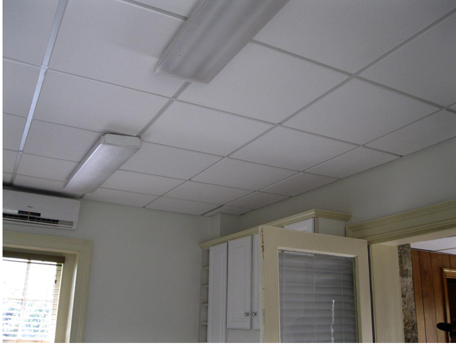
Acoustical tile ceiling in the Kitchen (Room #104). The tile will be removed and the piping run to sprinkler heads in the ceiling. A new tile ceiling will be installed.
