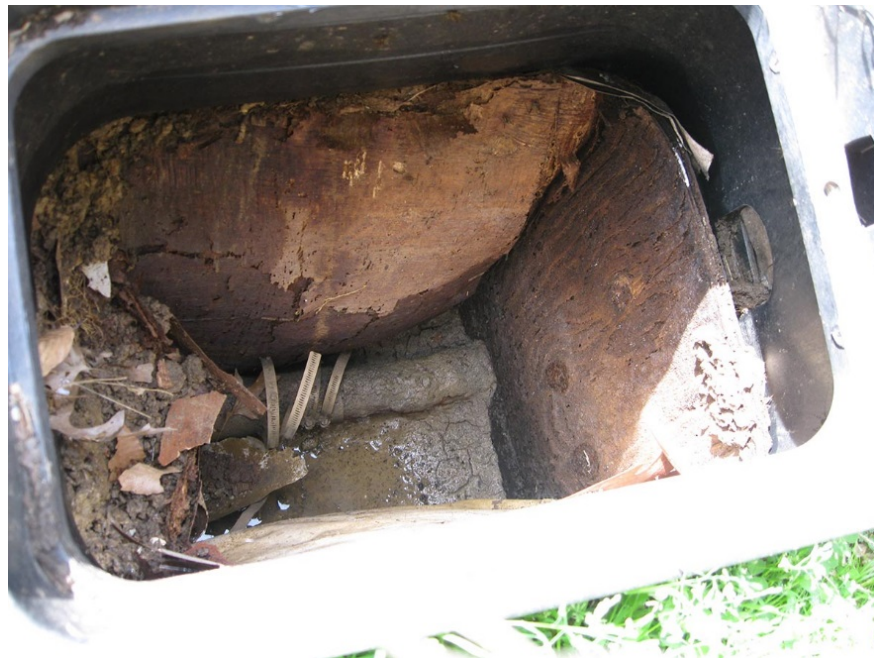
A close-up of the handhole shows the 2" waterline about three feet below the surface. The waterline will be excavated, removed and replaced with a 4" line within the same trench.
