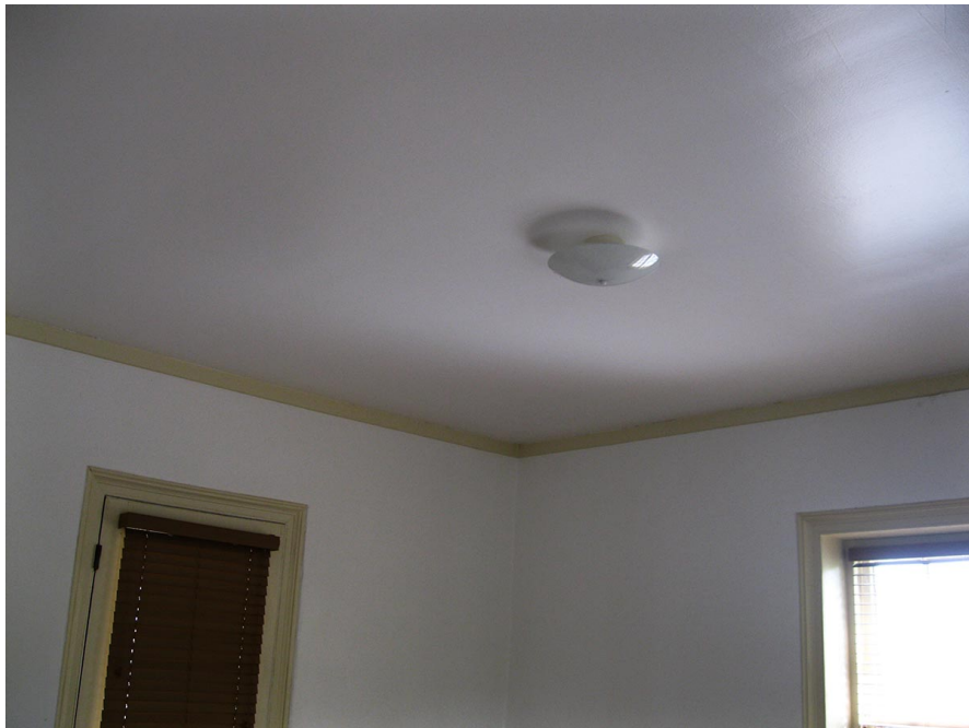
Gypsum ceiling in the Living Room (Room #101). The gypsum ceiling will be removed and the piping run to sprinkler heads in the ceiling. A new gypsum ceiling will be installed.
