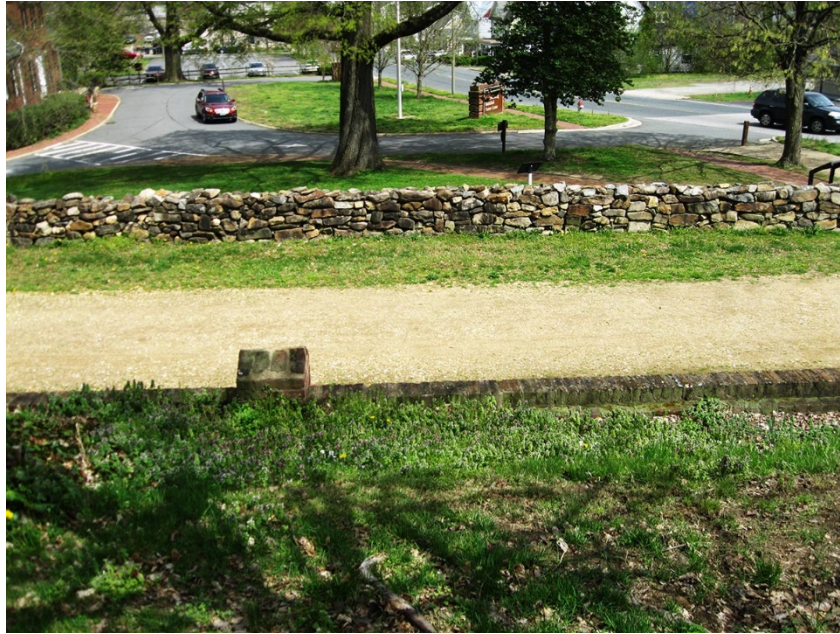
Looking east across the cemetery lodge lawn, the brick cemetery wall, Sunken Road to 1930s reconstructed stone wall. A 2" water line runs across the front of the lodge, under the brick cemetery wall, across the road and to the stone wall. The waterline will be excavated, removed and replaced with a 4" line within the same trench.
