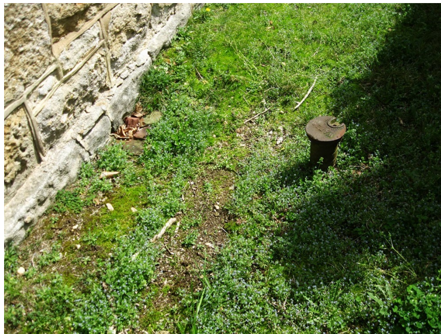
Part of the waterline infrastructure shows the proximity of the 2" waterline on the west face of the cemetery lodge. At this point the waterline enters the lodge to the left. The waterline will be excavated, removed and replaced with a 4" line within the same trench.
