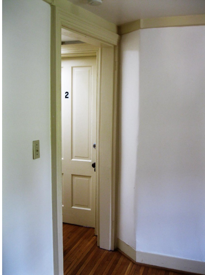
Looking into the southeast corner of the second floor Hall (Room #203). A small chase will be built near the door to house the sprinkler piping that will run to a sprinkler head mounted on the wall in Room 201.
