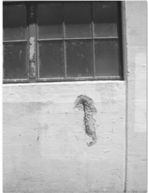
Another example of spalling concrete on Fort Mason Center building exterior
