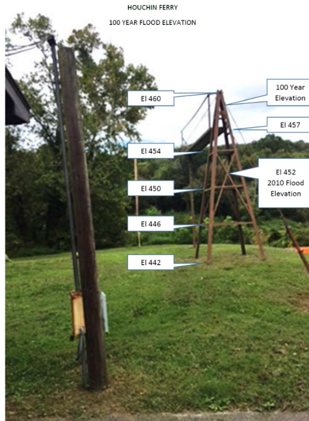
FIGURE B-4. FLOOD ELEVATIONS, SOUTH SIDE OF HOUCHIN FERRY SITE, AS MEASURED AGAINST FORMER FERRY TOWER. THE TOWER IS ON A CONTOURED BENCH ABOVE RIVER, WHICH FLOWS PAST THE TOWER IN THE BACKGROUND. THE PEDESTRIAN SUSPENSION BRIDGE WOULD BE AT THE 450-FOOT ELEVATION, WHICH IS BELOW THE 100-YEAR FLOOD ELEVATION.
