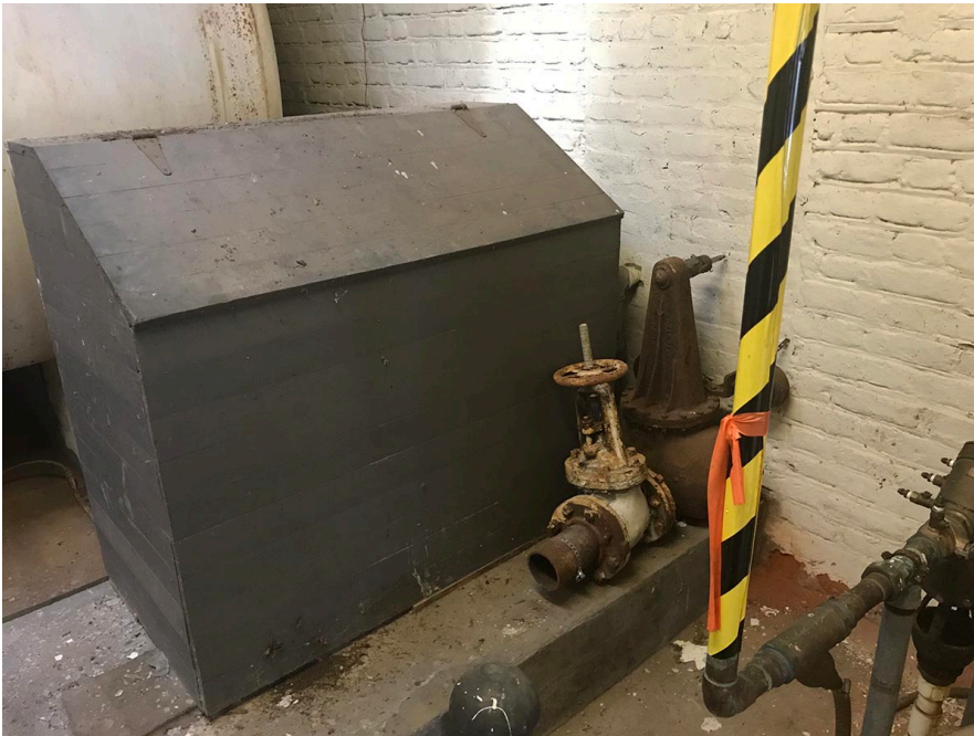
The room adjacent to the IT Server Room. The wood box will be removed and the heat pump will be installed in its place. The chase that will provide access for the lineset and power to the heat pump is located behind the box,
