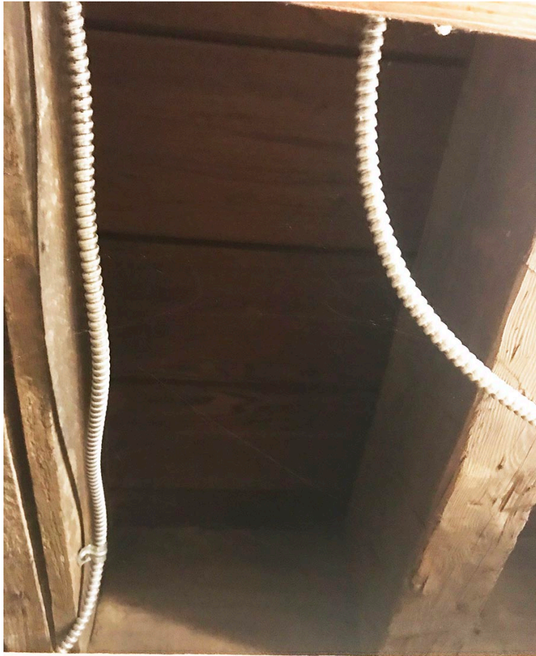
A view of the IT Server Room floor from the room below. Two 3/4" holes will be drilled in the wood floor to facilitate access of the lineset, power and condensate lines.
