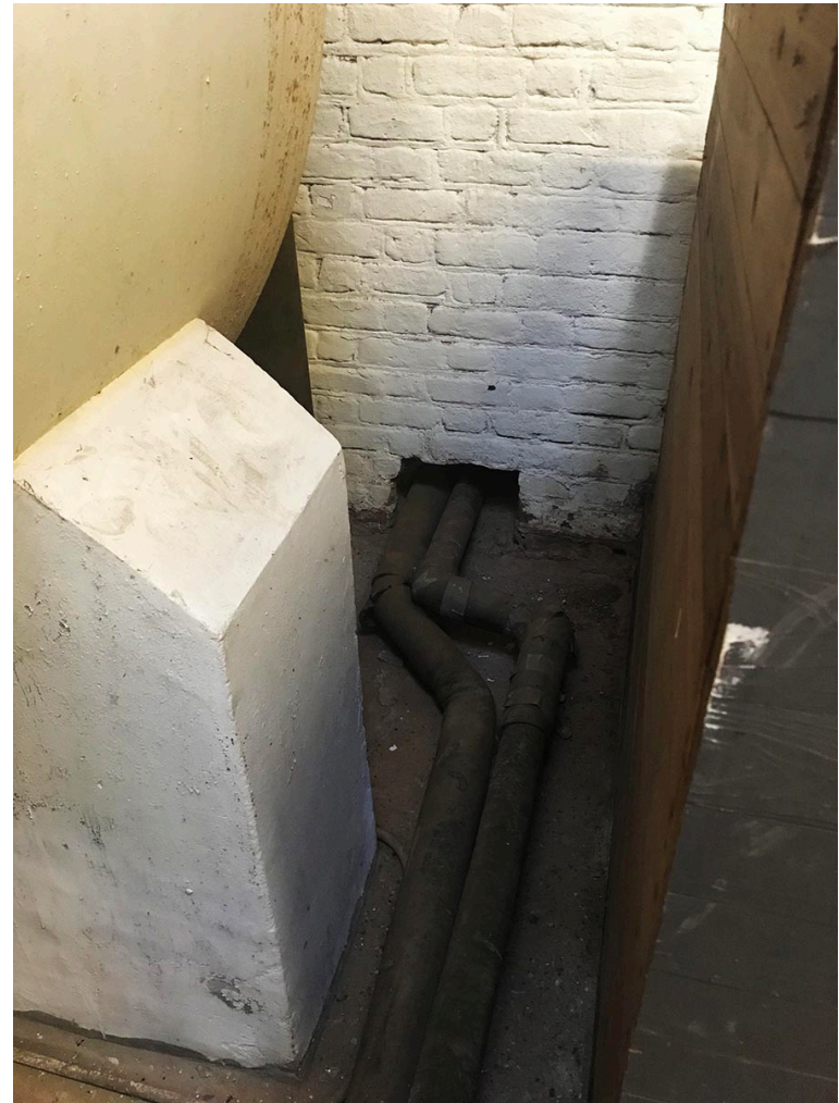
The chase that will provide access for the lineset and power to the heat pump.
