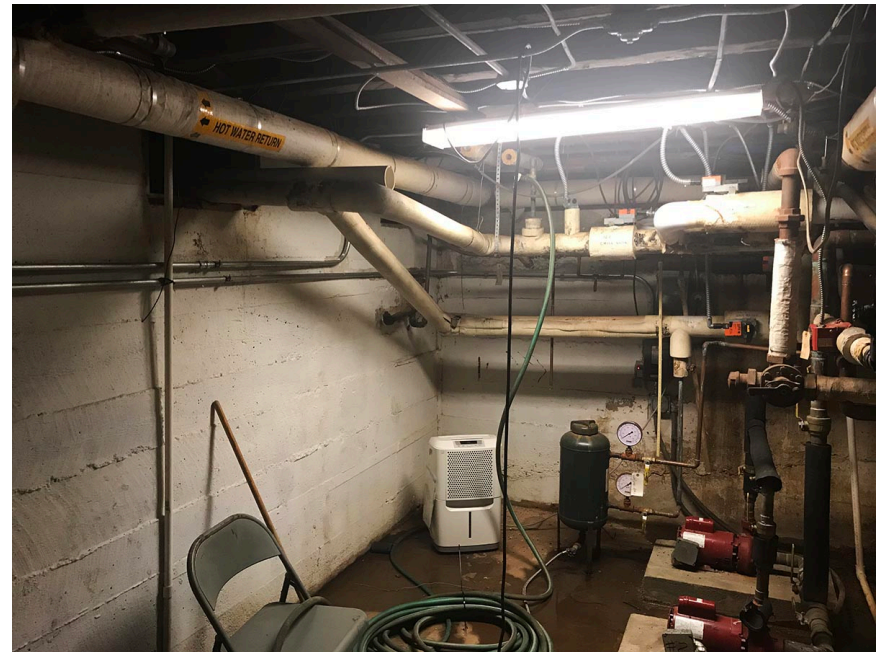
The room beneath the IT Server Room. The condensate line from the new HVAC unit will penetrate the ceiling of this room and empty into the sump in the floor.
