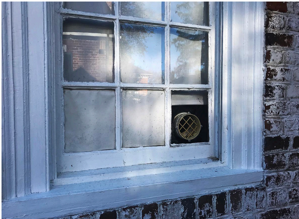
Exhaust from current floor air conditioner used in the IT Server Room
