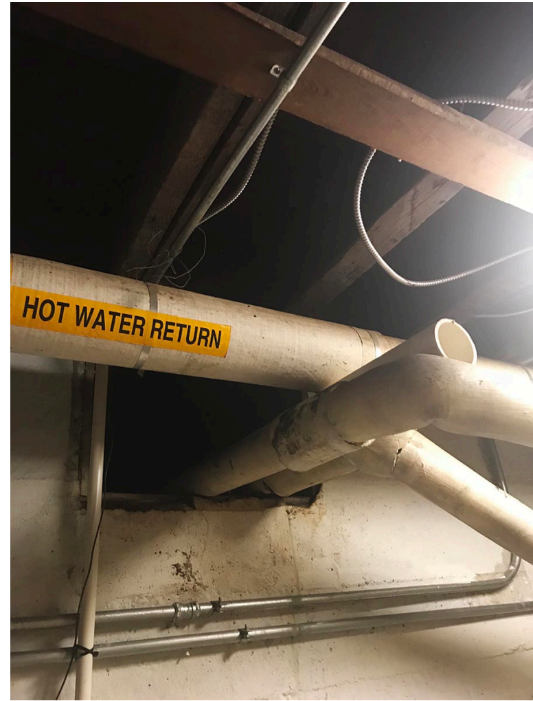
The lineset and power lines will run through this existing chase into the adjacent room where the heat pump will be installed.
