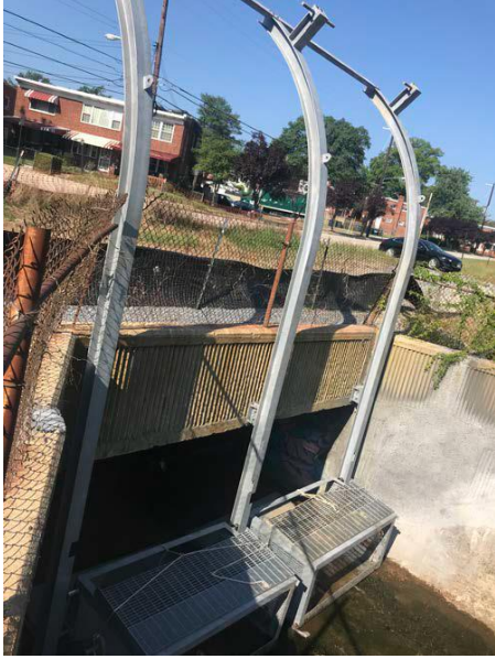
Figure 3. Photo of Outfall #999 Stormwater Trash Cage, Washington, DC (Living Classrooms, 2015).
