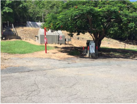
Photoplate 7. Area 2: Gasoline (lower) and diesel (upper) tanks, fuel pump.
