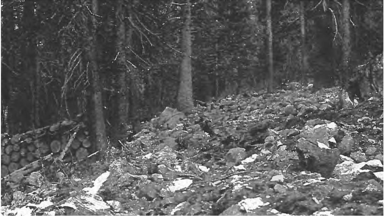
Figure 2-20. Electric blasting was used in rocky sections as in construction of Campground Road D in 1932 (source: YOSE 1932 Superintendent's Report).
