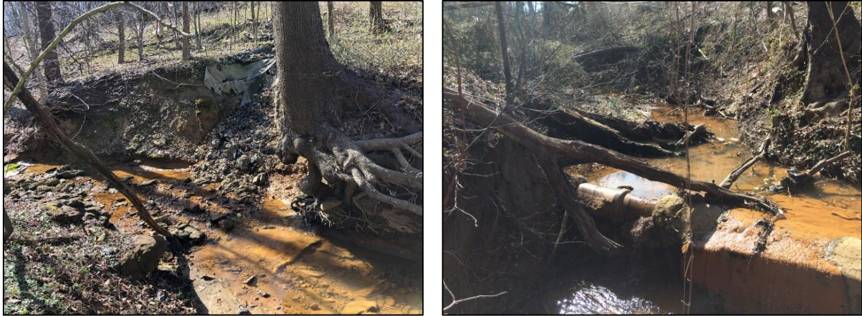
Figure 3. Streambank Erosion (left) and Exposed Sewer Line (right)
