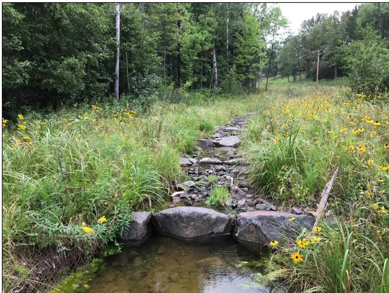
Figure 5. Representative Photograph of Post-Construction Restoration Conditions using Natural Channel Design Techniques
