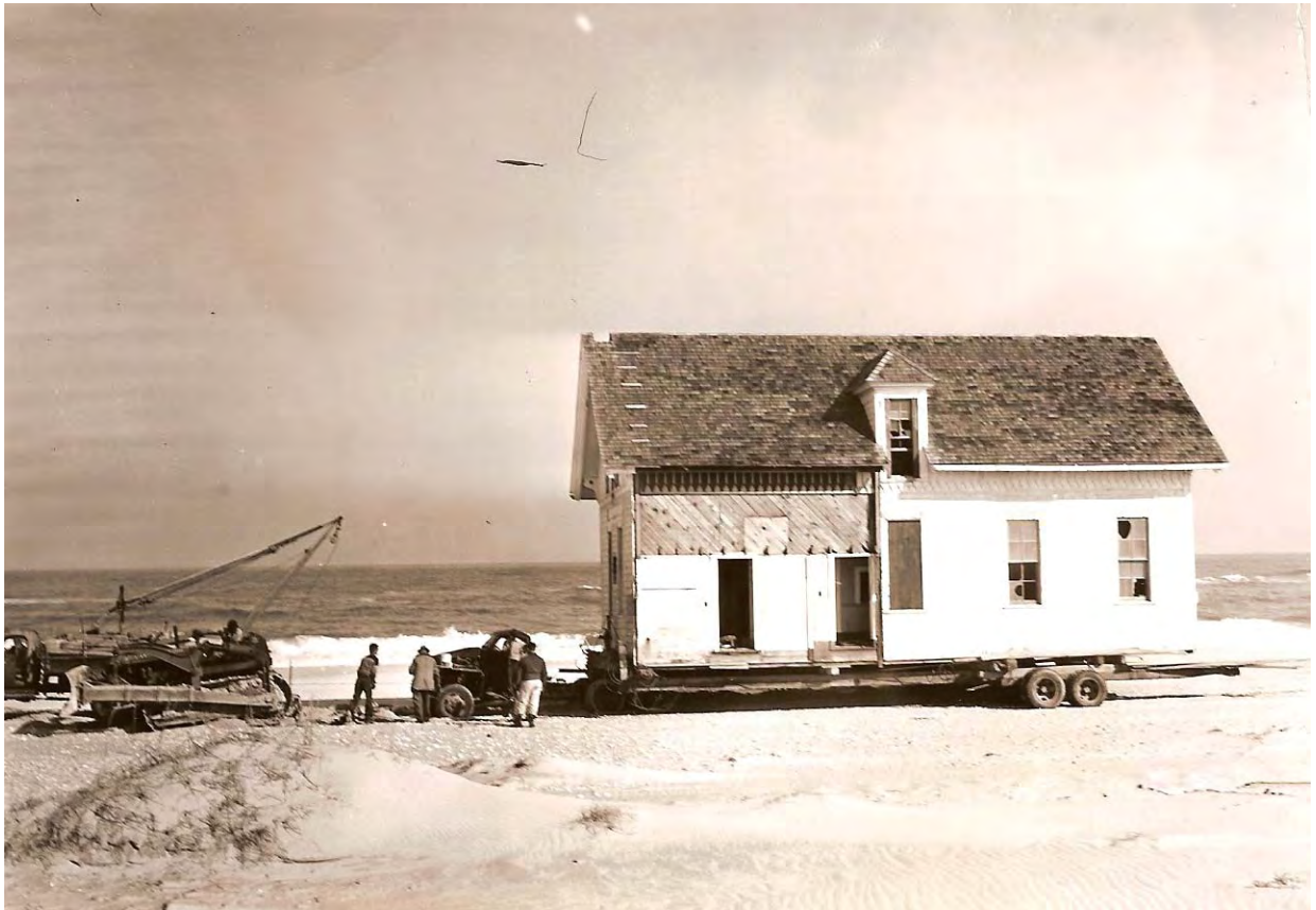
Figure 12. Relocation of the USLS Station in progress during 1955.
