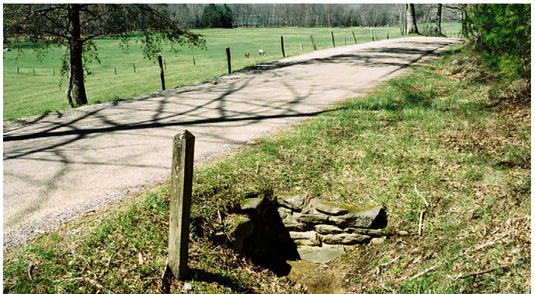
Figure 45. Stone headwalls around culvert and fence. JMA 2003
