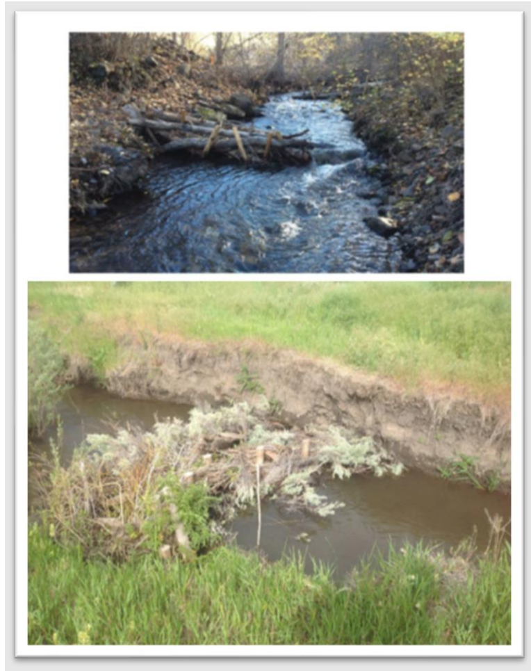
Figure 3. Two examples of post-assisted log structures or PALS (Wheaton et al. 2019).
