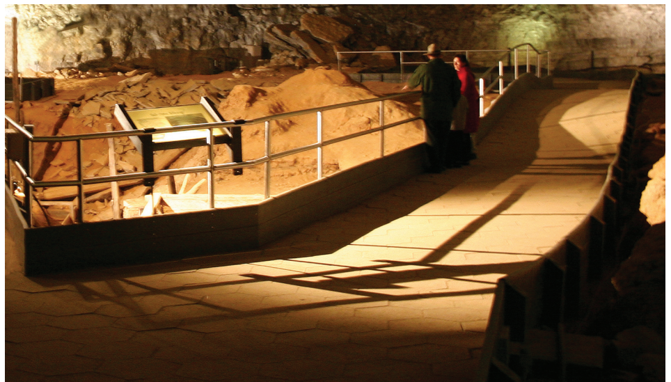
Concrete pavers on the prototype trail installed in the Historic Section of Mammoth Cave.
