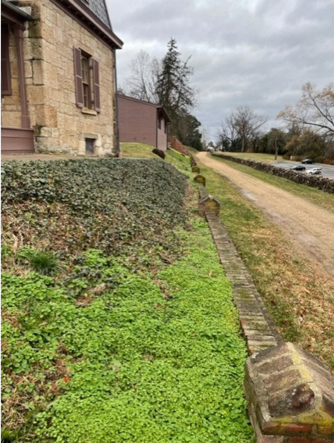
View of the steep escarpment adjacent to the cemetery's eastern wall and panels 142-145. This area will be excavated, and temporary shoring provided while the panels are reconstructed. Looking north up Sunken Road.
