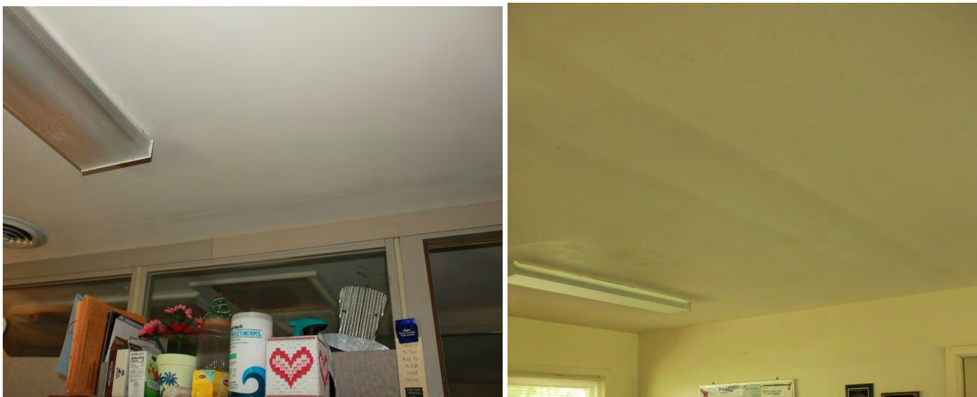
Caption: ED 221_7, Building 40, Interior ceiling showing sagging central support resulting from removed walls
