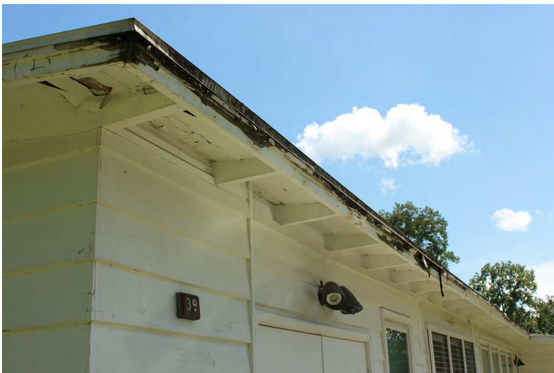
Caption: ED 220_6, Building 39, Fascia boards, showing severe deterioration due to no gutters in original design
