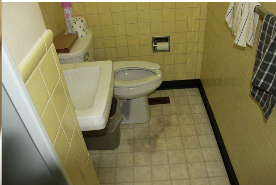
Caption: ED 220_10, Building 39, Bathroom floors that are rotted and creating mold conditions
