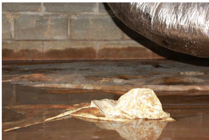
Caption: ED 222_8, Building 41, Crawl space showing standing water and mold on surfaces
