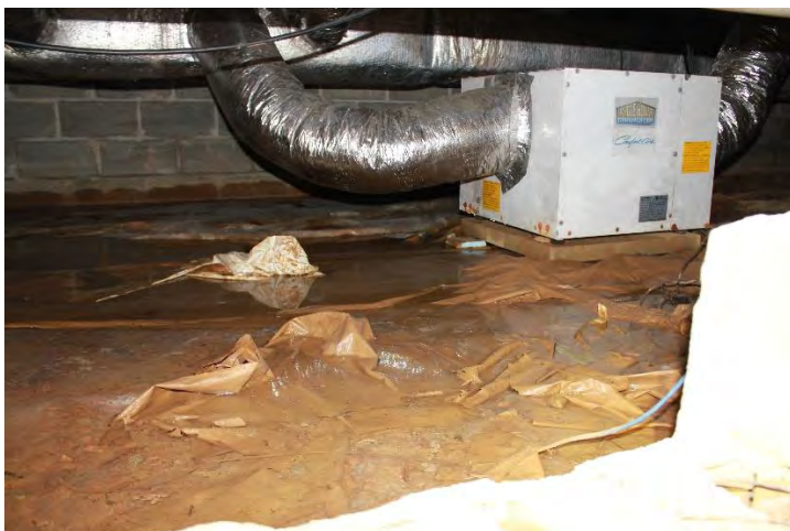
Caption: ED 222_8, Building 41, Crawl space showing standing water and mold on surfaces
