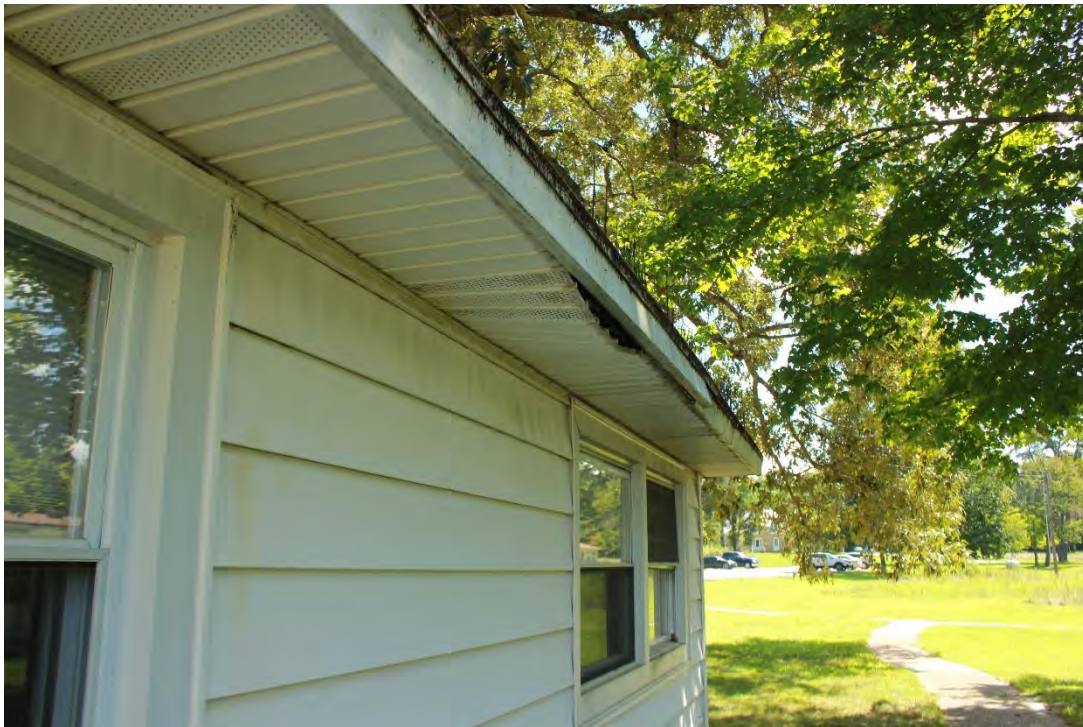
Caption: ED 219_4, Building 37, Soffits are collapsing in multiple places from the eaves and fascia is deteriorated
