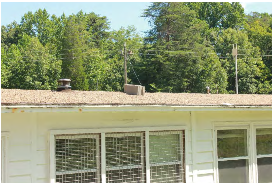
Caption: ED 220_5, Building 39, Built up roof, showing signs of failure and blocks holding down loose tar paper
