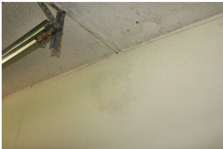
Caption: Ed 223_5, Building 42, Water damage and cracking in the ceiling and wall
