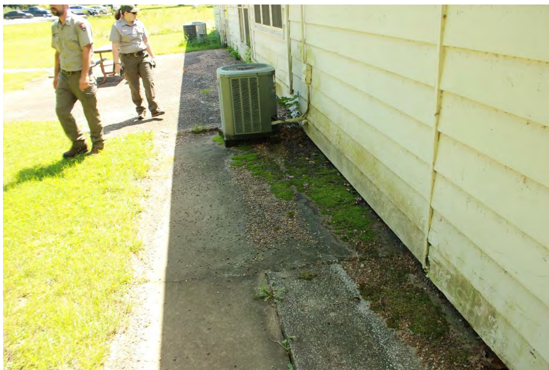
Caption: ED 220_7, Building 39, Washed out gravel accumulating below eaves of built up roof
