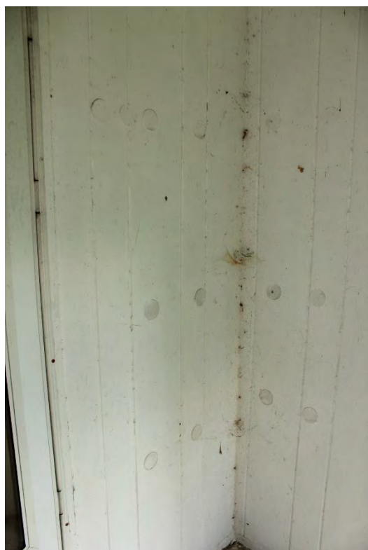
Caption: ED 217_6, Building 34, siding has been perforated with ~4" holes and plugged across the walls of the entire building
