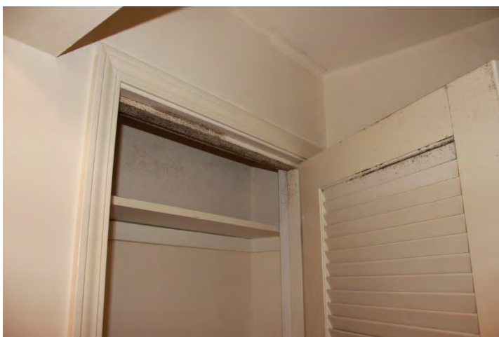
Caption: ED 217_8, Building 34, mold is present in nearly every room and in closets and storage areas
