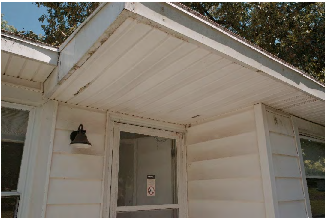
Caption: ED 219_5, Building 37, Doorway awning is deteriorated and sagging
