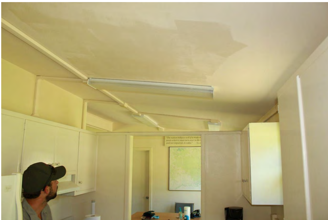
Caption: ED 220_9, Building 39, Water damage in the ceiling, repaired and continuing to fail
