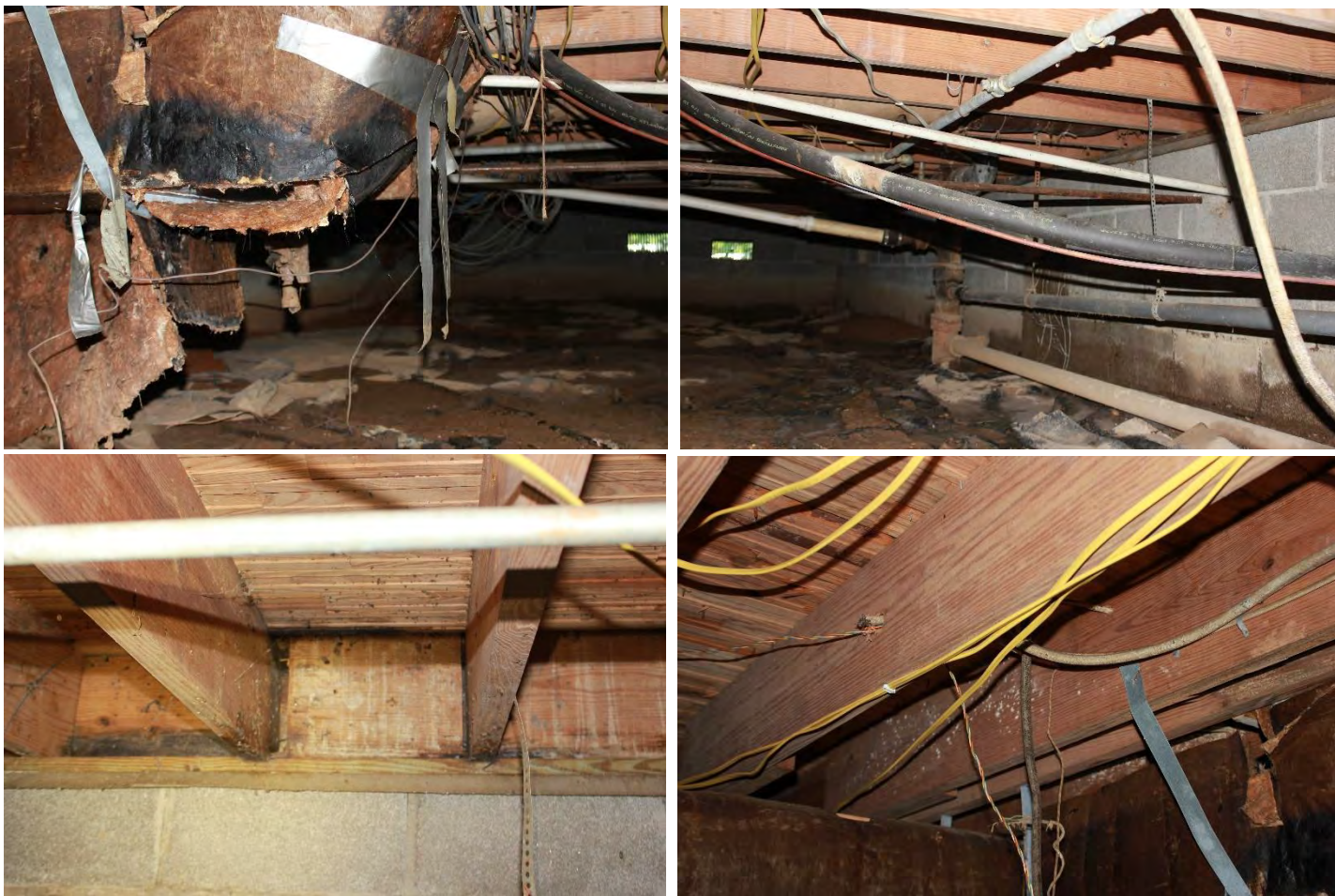
Caption: ED 221_9, Building 40, Collage of images from the crawl space, showing mold and moisture damage throughout
