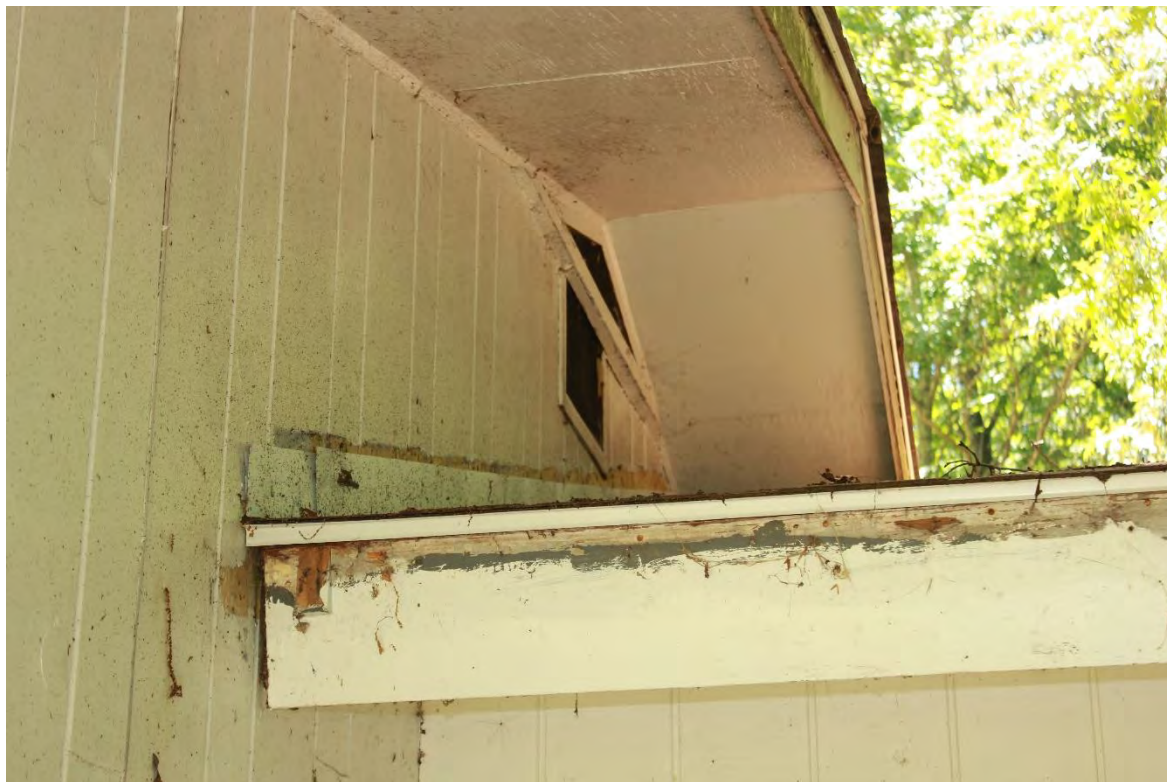
Caption: ED 217_5, Building 34, garage extension roof is pulling away from house and sagging
