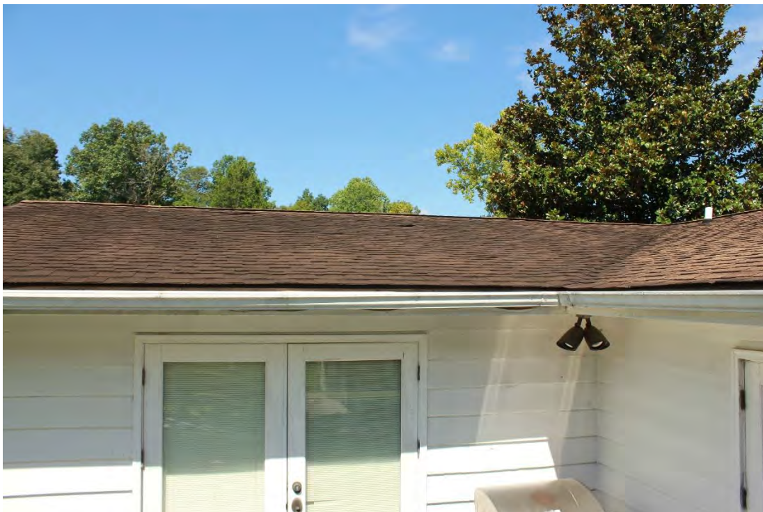
Caption: ED 222_5, Building 41, Roof line above addition, showing uneven and wavy surface with shingles coming loose.
