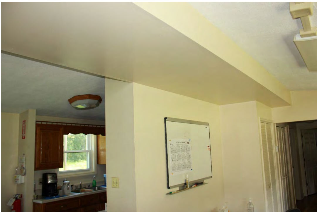
Caption: ED 219_7, Building 37, Central rafter beam is covered and ceiling dropped to house ductwork
