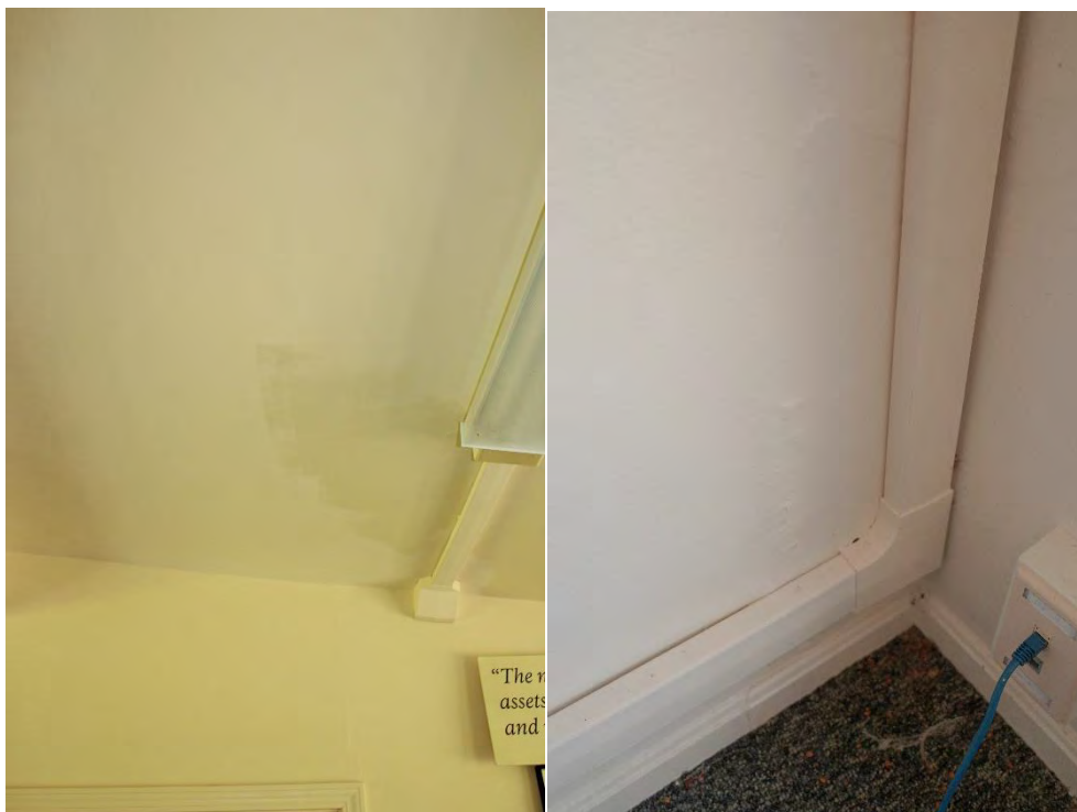
Caption: ED 220_8, Building 39, Samples of water damage on the ceiling and walls, evident in over 12 locations in the building
