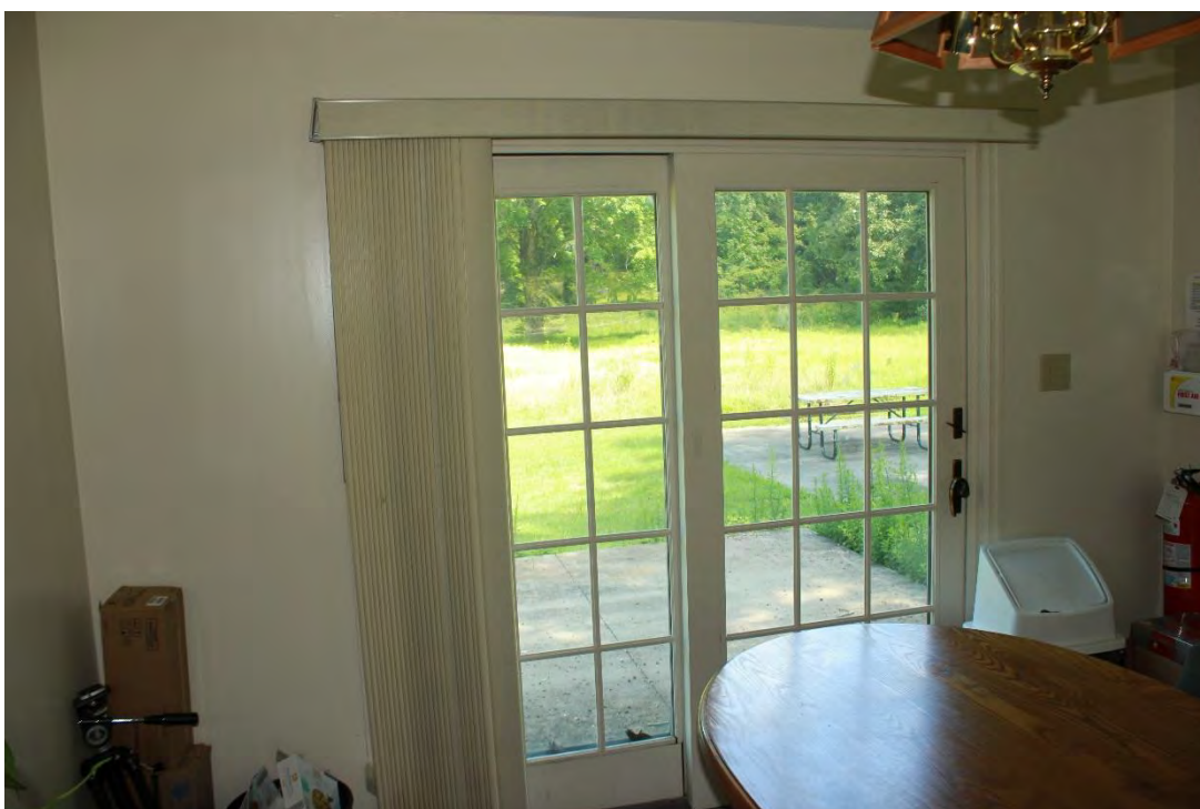
Caption: ED 219_8, Building 37, French door-style slider installed to replace original sliding patio door
