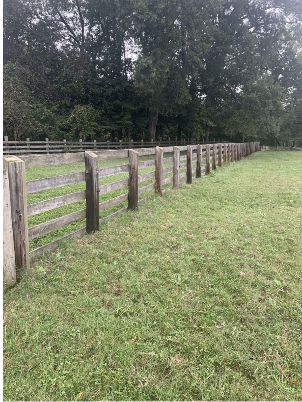
Figure 3. Existing north side of the corral fence.
