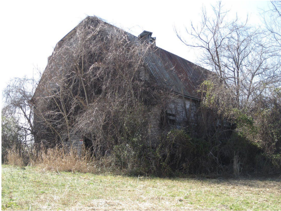
Link Dairy Barn – Northeast
