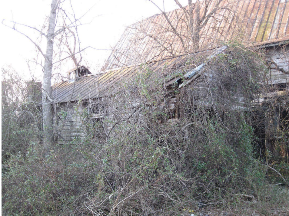
Link Pole Vehicle Shed – Northwest
