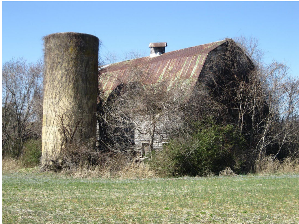
Link Dairy Barn and Silo– Southeast
