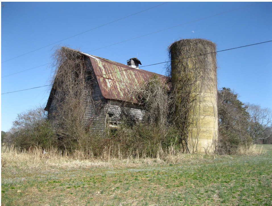
Link Dairy Barn and Silo– Southwest
